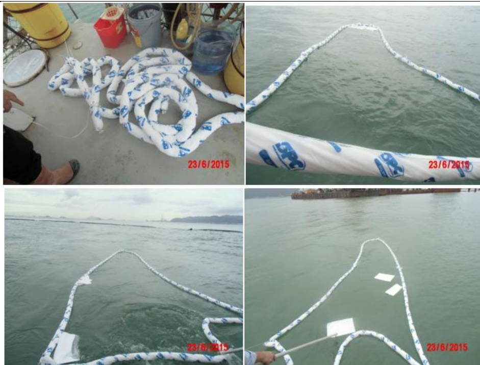
6.4.23 The used absorption booms were collected using disposal bags as part of the spill kits item. The used absorption booms were disposed of as chemical waste by the Contractor. (Also refer to photo record below)
