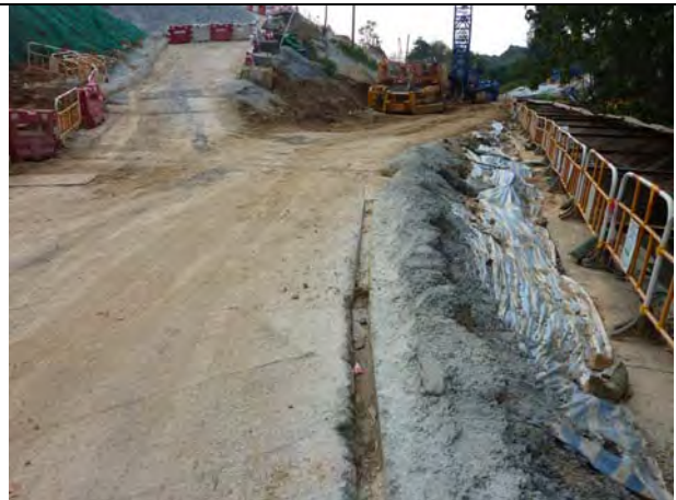
Photo 4 Concrete bund was constructed next to the channel.
