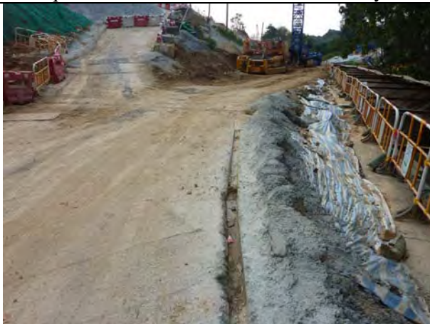
Photo 5 Concrete bund was constructed next to the channel.
