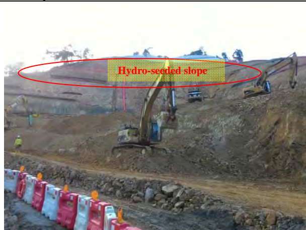
Photo 3 Slope excavation at North Portal was carried out on 28 and 29 January 2016
