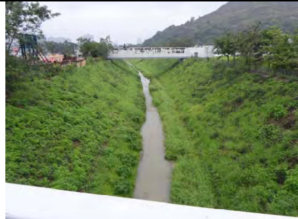
Photo 1 Turbid water was observed at WM4 on 15 January 2016
