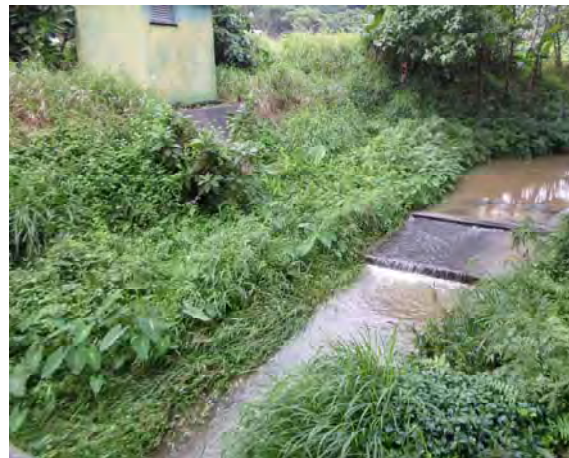
Photo 1 Turbid water was observed at WM2A during water monitoring on 16 January 2016.
