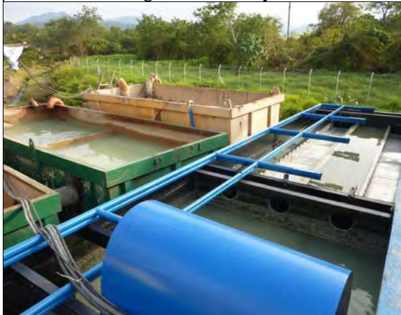
Photo 3 Wastewater treatment facilities was installed for piling work at Bridge D.
