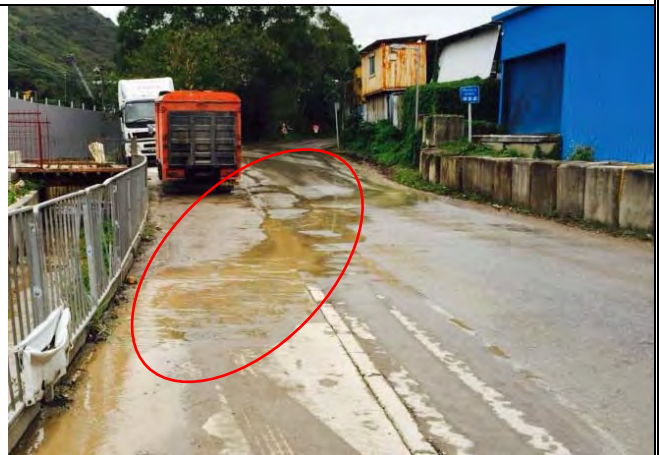
Photo 6 During the course of monitoring on 16 January 2016, muddy runoff from the public road surface into the existing channel was observed after rain.
