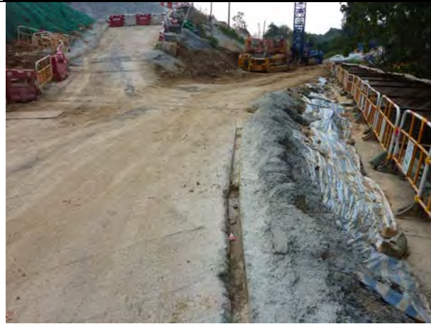
Photo 7 Concrete bund was constructed next to the channel.
