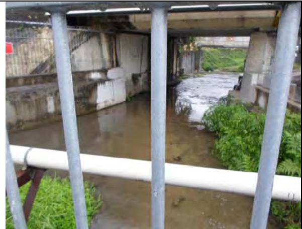
Photo 2 Turbid water was observed at WM4-CA on 15 January 2016
