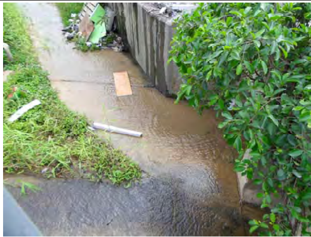
Photo 1 Very shallow water at WM2B on 18 January 2016 and cumulated silt was observed at the channel bed.
