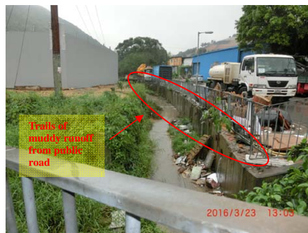
Photo 1 During water sampling on 23 March 2016, shallow water was observed at WM2B and the water quality at WM2B was turbid.
