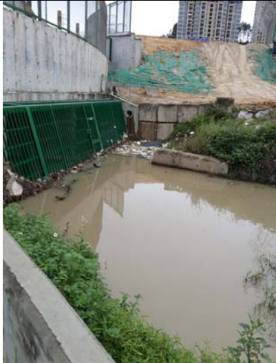
Photo 1 During water sampling on 10 March 2016, turbid water was observed at WM1.
