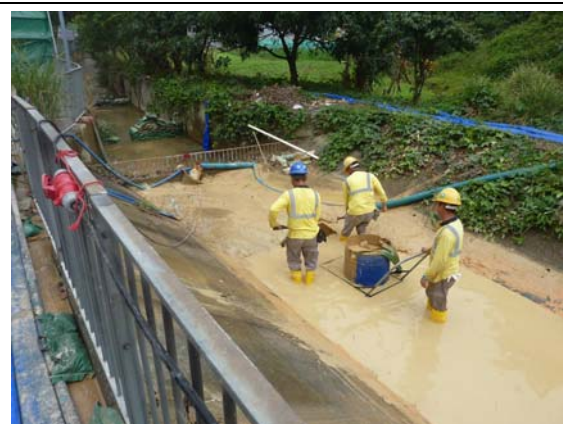
Photo 6 Desilting of open channel was carried on 8 March 2016. The turbid water was blocked by the bar screen to prevent it flowing further downstream.
