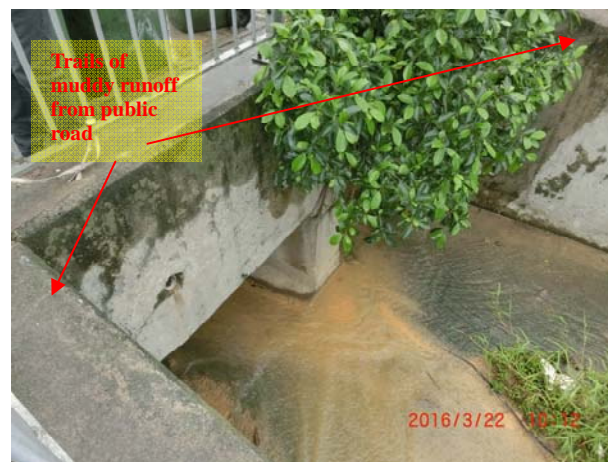
Photo 3 During water sampling on 22 March 2016, shallow water was observed at WM2B and the water quality at WM2B was slightly turbid.
