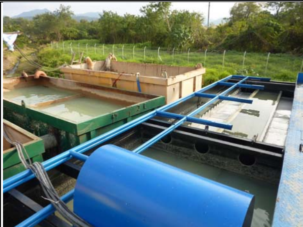
Photo 3 Wastewater treatment facilities was installed for piling work at Bridge D.
