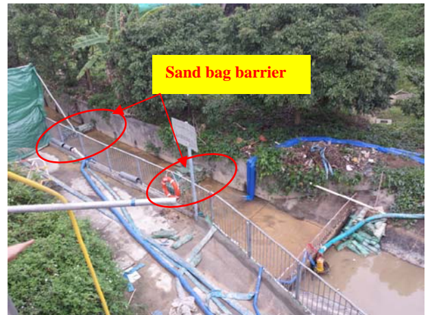
Photo 8 During site inspection on 10 March 2016, it was observed that desilting of open channel was carried out.
