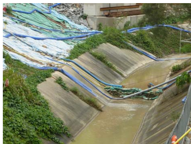
Photo 5 The effluent of the AquaSed was visually clear.
