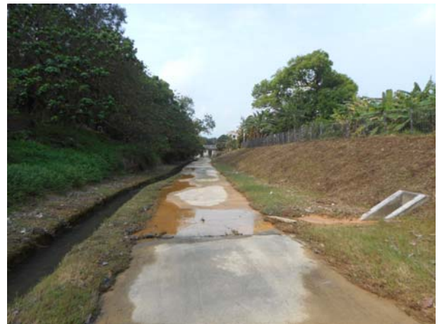
Photo 8 Discharge of turbid water and accumulated silt was observed from an unknown outfall which located at between the works area of C6 and WM3 on 30 March 2016.
