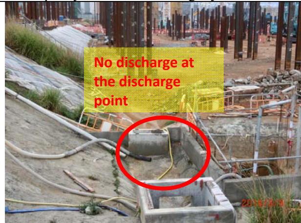
Photo 4 During site inspection on 9 March 2016, there was no discharge observed from the wastewater treatment system.
