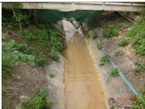
Photo 5 The effluent in the nullah which connected to Ng Tung River was visually clear during site inspection on 7 April 2016.
