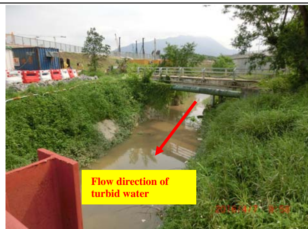
Photo 12 On 7 April 2016, turbid water was observed at upstream of the works area of Contract 6. (works area of Contract 6 is after the Bridge)
