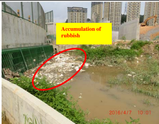
Photo 9 During water sampling on 7 April 2016, accumulation of rubbish were observed at the bar screen of the box culvert near WM1 and cumulated turbid water was observed at WM1.
