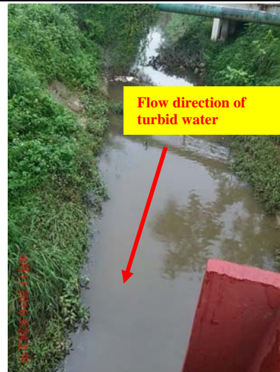
Photo 16 On 8 April 2016, turbid water was observed at upstream of the works area of Contract 6. (works area of Contract 6 is after the Bridge)
