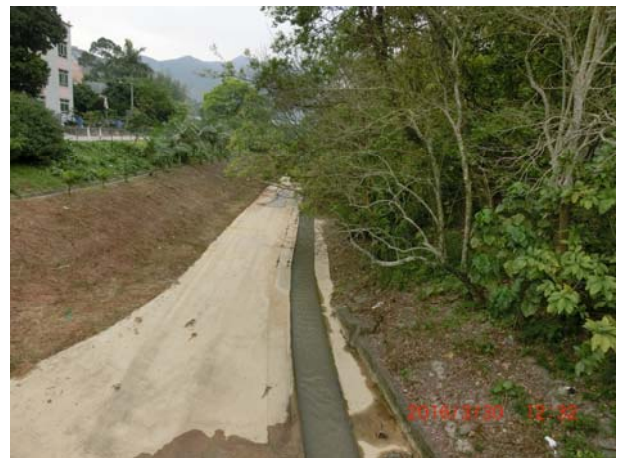
Photo 2 Muddy water was observed at WM3 on 29 March 2016
