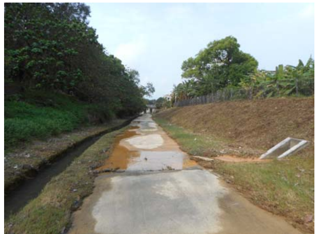
Photo 8 Discharge of turbid water and accumulated silt was observed from an unknown outfall which located at between the works area of C6 and WM3 on 30 March 2016.
