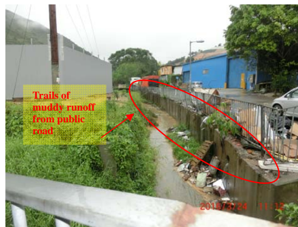
Photo 3 During water sampling on 24 March 2016, shallow water was observed at WM2B and the water quality at WM2B was slightly turbid.
