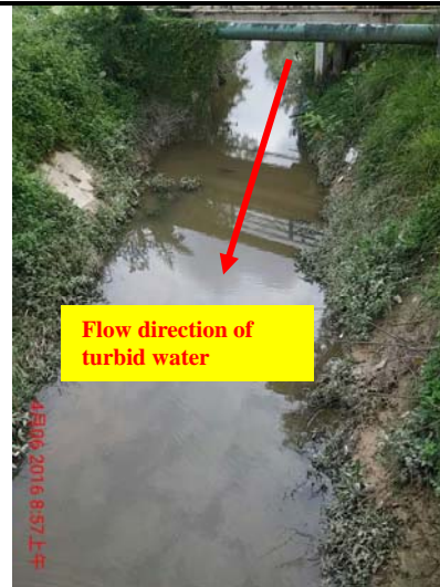
Photo 8 On 6 April 2016, turbid water was observed at upstream of the works area of Contract 6. (works area of Contract 6 is after the Bridge)
