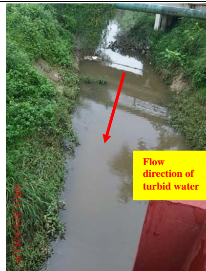
Photo 4 On 11 April 2016, turbid water was observed at upstream of the works area of Contract 6. (works area of Contract 6 is after the Bridge)
