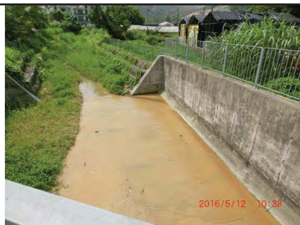
Photo 6 Turbid water was observed at WM3-C on 12 May 2016.
