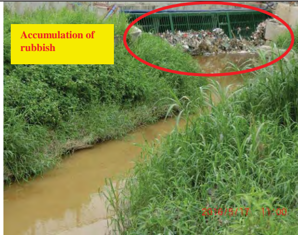
Photo 1 During water sampling on 17 May 2016, turbid water was observed at WM1. Accumulation of rubbish was also observed at the Box Culvert at WM1.
