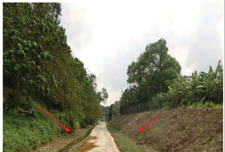
Photo 4 Surface runoff from the nearby slopes into the river channel may make the water become more turbid under heavy rain.
