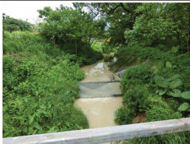
Photo 1 During water sampling on 27 May 2016, turbid water was observed at WM2A.
