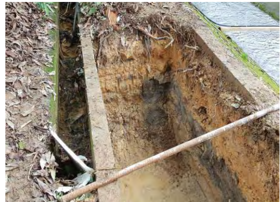
Photo 10 Temporary drain ditch was constructed to collect runoff.
