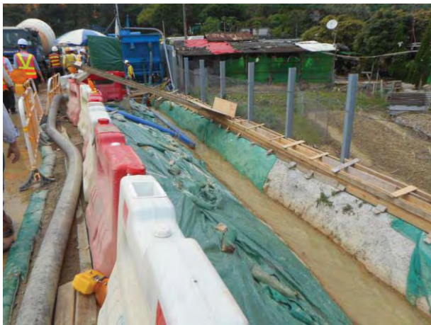
Photo 7 During site inspection on 21 April 2016, the effluent of the AquaSed (SH-8) was found to be turbid.
