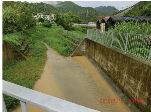
Photo 4 Turbid water was observed at WM3-C on 10 May 2016.
