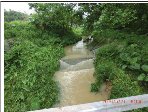
Photo 1 During water sampling on 21 May 2016, turbid water was observed at WM2A.
