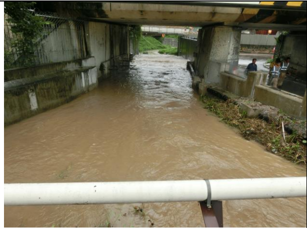
Photo 2 Turbid water was observed at WM4-CA on 6 June 2016.
