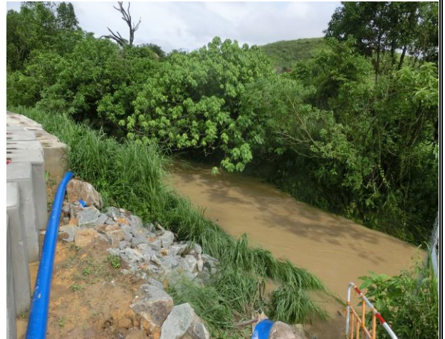
Photo 4 During water sampling on 6 June 2016, turbid water was observed at WM2A.
