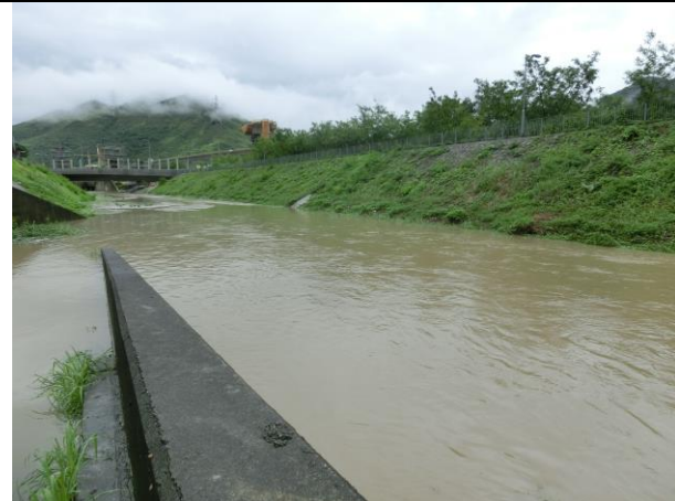
Photo 3 Turbid water was observed at WM4-CB on 6 June 2016.
