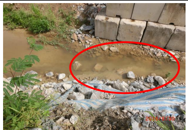
Photo 6 During joint site inspection on 30 June 2016, it was observed that unknown source of turbid water was seeping out from the river bed.
