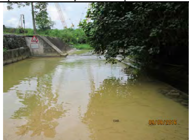
Photo 6 During site inspection on 9 September 2016, it was observed that the water quality at downstream of site area was clear but some obvious silt and sediment was observed at the channel bed.
