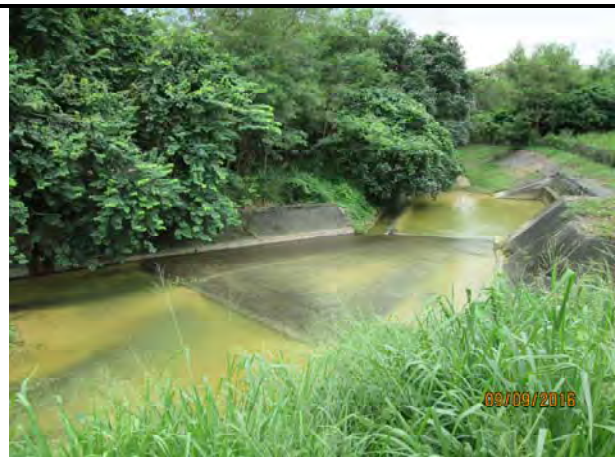
Photo 5 During site inspection on 9 September 2016, it was observed that the water quality at downstream of site area was clear but some obvious silt and sediment was observed at the channel bed.
