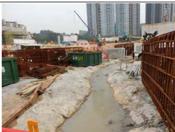
Photo 5 If water discharge is required, it will follow the temporary site drainage plan in which wastewater would be diverted to the perimeter channel and then collected to the wastewater treatment plant for treatment before discharge.
