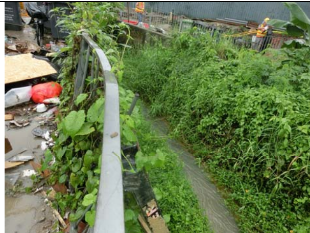
Photo 5 On 10 September 2016, the water flowing at WM2B was slight cloudy after rain.
