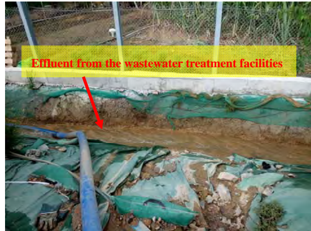
Photo 4 The effluent from the wastewater treatment facilities was visually clear.
