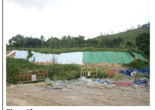
Photo 12 The exposed slopes have been covered with tarpaulin as far as practicable.
