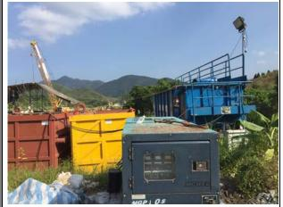
**Photo 9** Wastewater treatment facilites were provided for Bridge D
