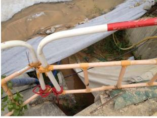
**Photo 6** Discharge of turbid water to the gully by other Contractor at Sha Tau Kok Road was observed on 16 November 2016.
