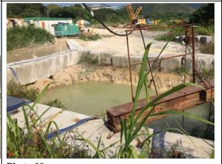
**Photo 10** A sump pit was constructed to preliminary settled the particulates in the water before diverted to the AquaSed for proper treatment.
