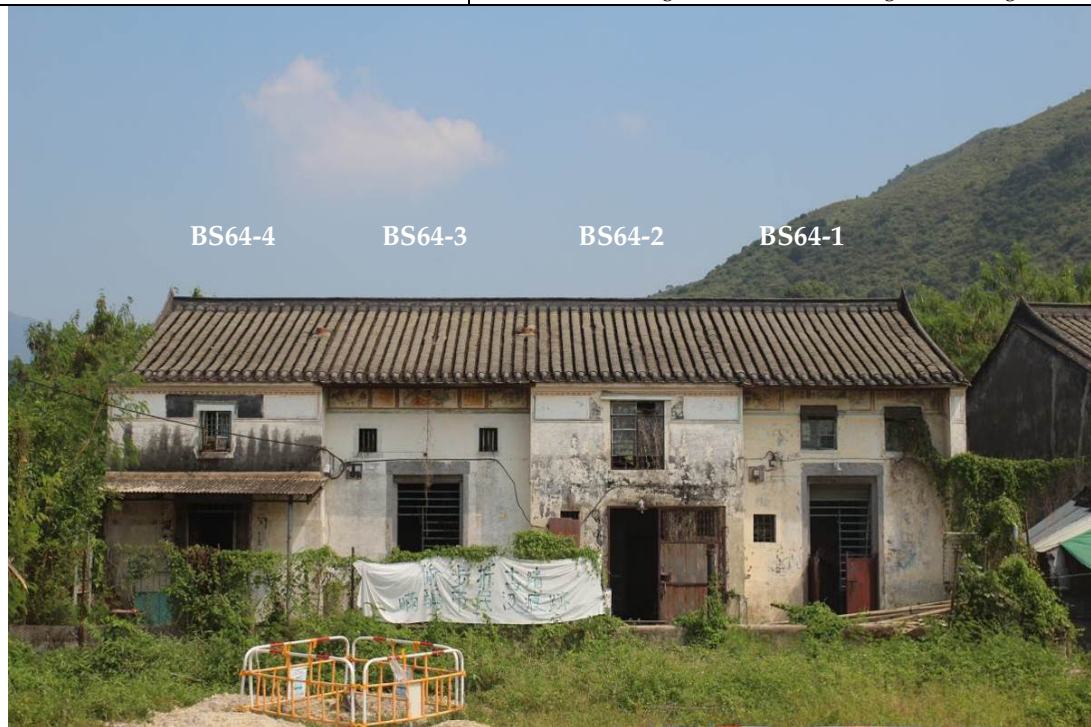
BS64-overall-P3 Façade of BS64 BS64正立面
