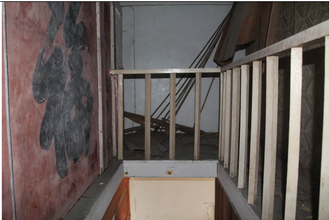
BS64-1-P21 View of the balustrade of the stair 樓梯欄杆概貌
