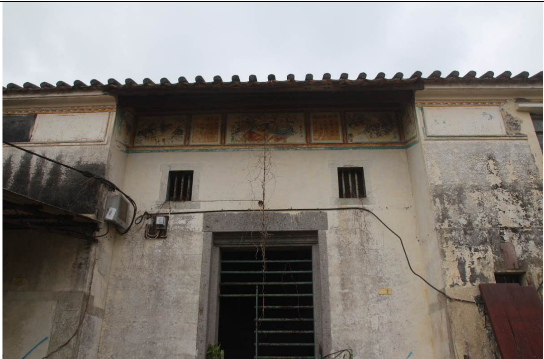
BS64-3-P3 Wall decoration of the façade of BS64-3 BS64-3正立面裝飾
