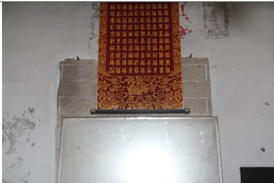
BS65-2-P38 Brick line decoration on the mud wall beneath the cockloft 閣樓下泥牆的牆線裝飾
