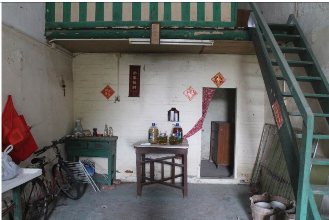
BS65-1-P9 Brick wall under the cockloft 閣樓下磚牆
