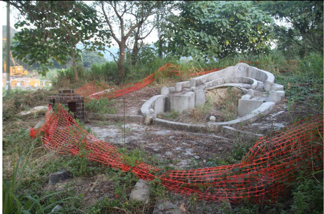
GR08-P1 Identification view of GR08 (view from west) GR08識別圖(攝自西方)
