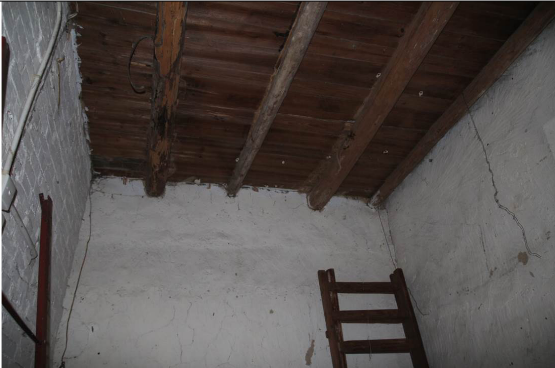
BS65-1-P10 General view of the room 房間概貌
