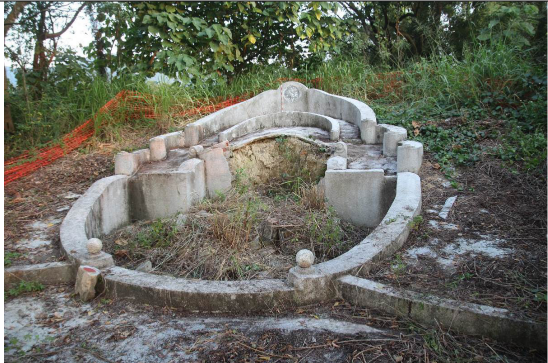
GR08-P2 Oblique view of GR08 (view from west) GR08斜視圖(攝自西方)
