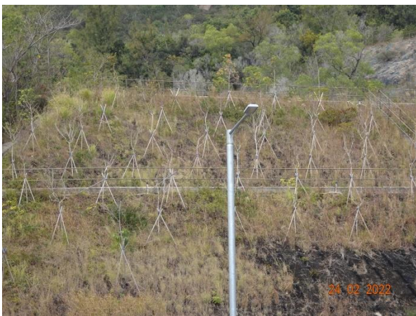
General View for Slope TP_B
