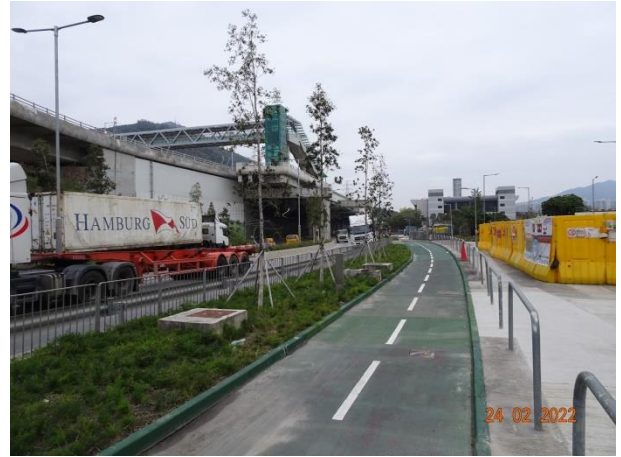
General View for Lung Mun Road
