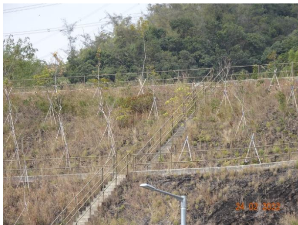
General View for Slope TP_B
