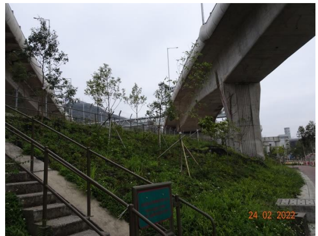
General View for Slope 5SE-D/C16
