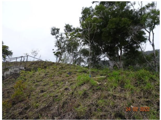
General View for Slope 5SE-D/C21
