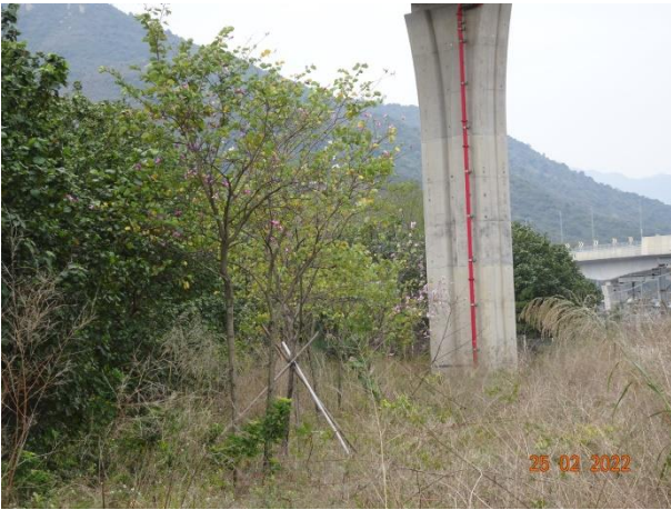
General View for Zone 3D
