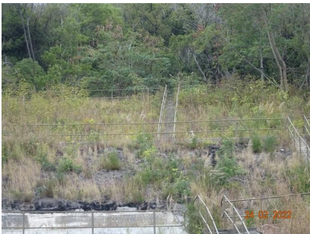
General View for Slope TP_A
