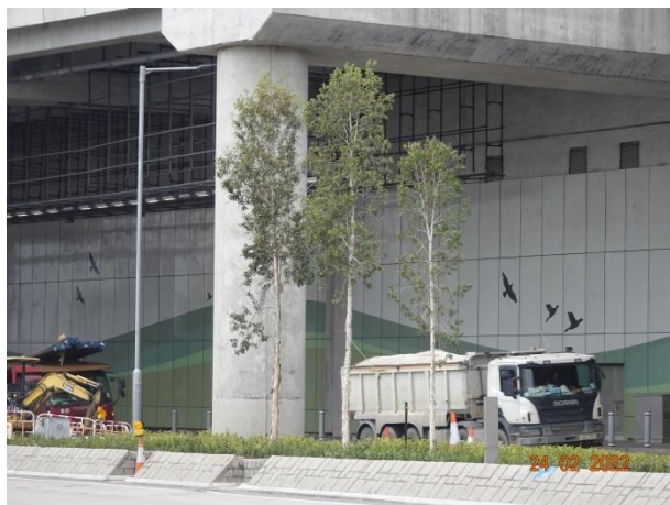
General View for Lung Mun Road
