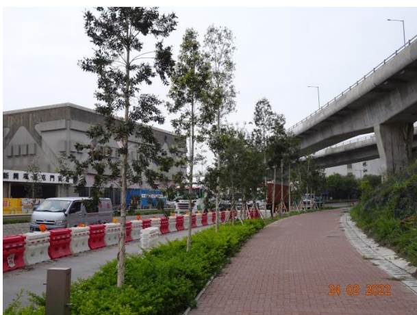
General View for Lung Mun Road
