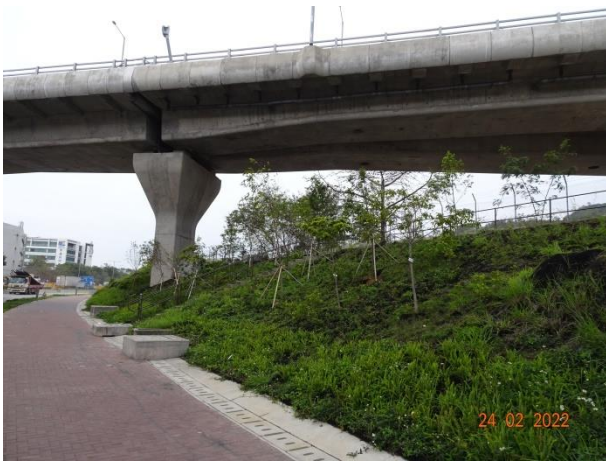
General View for Slope 5SE-D/C16
