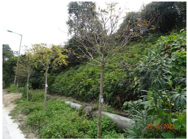
General View for Zone 1D
