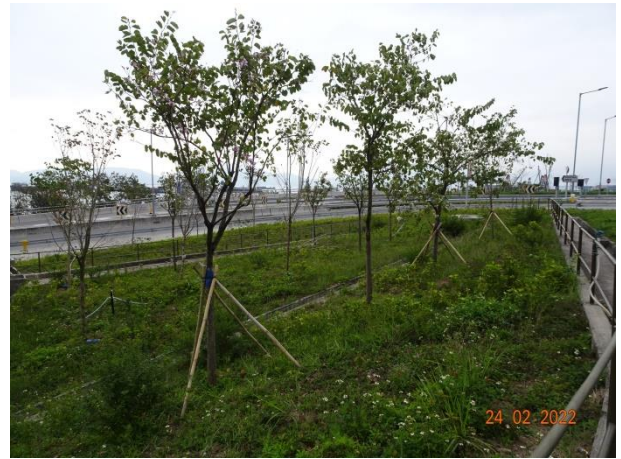
General View for Slope 5SE-D/C215
