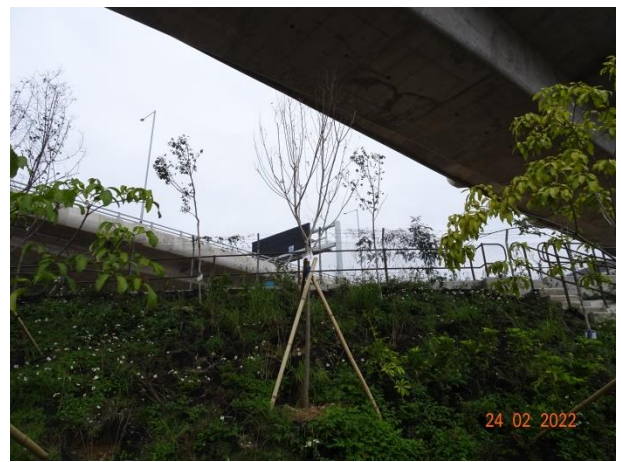
General View for Slope 5SE-D/C16
