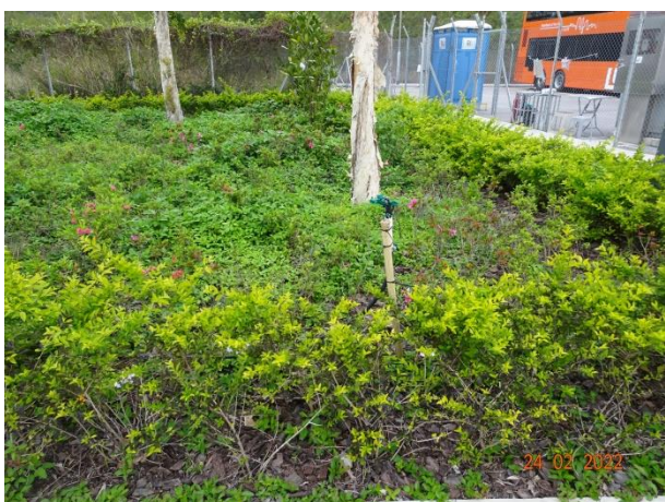
Watering system at Toll Plaza Interchange
