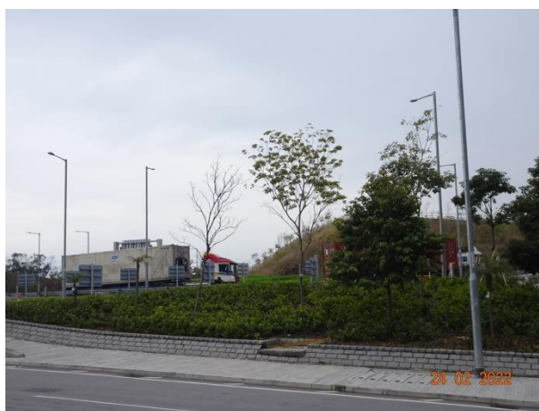
General View for planter near the Tunnel
