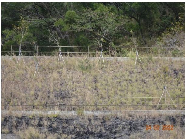
General View for Slope TP_B
