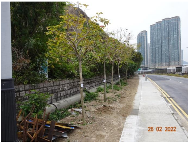
General View for Zone 1D
