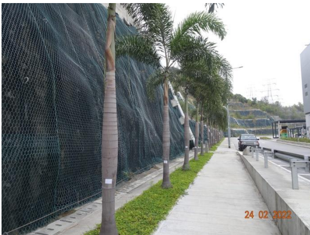
General View for Toe Planter
