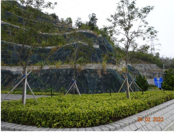
General View for Toe Planter
