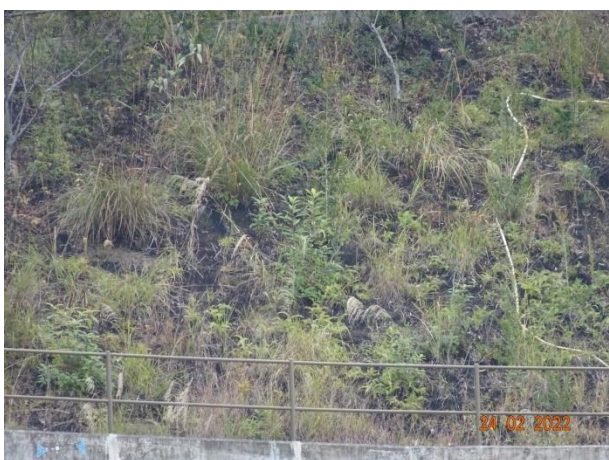
General View for Slope TP_D
