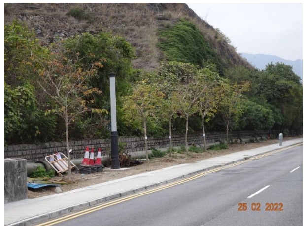
General View for Zone 1D
