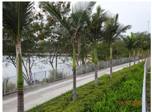
General View for cycling track near Butterfly Bay Beach
