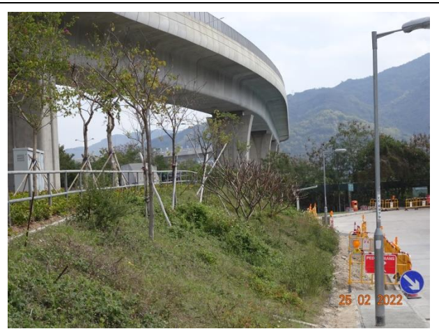
General View for Zone 1B
