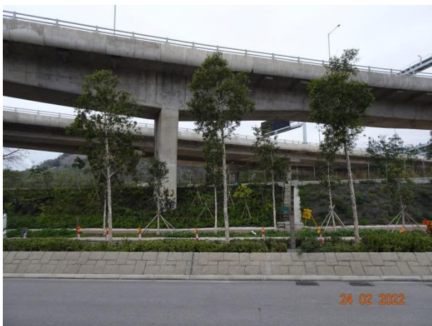
General View for Lung Mun Road
