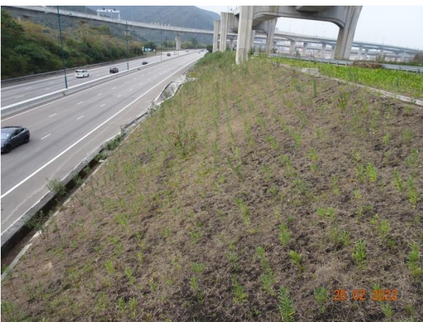
General View for Zone 3D
