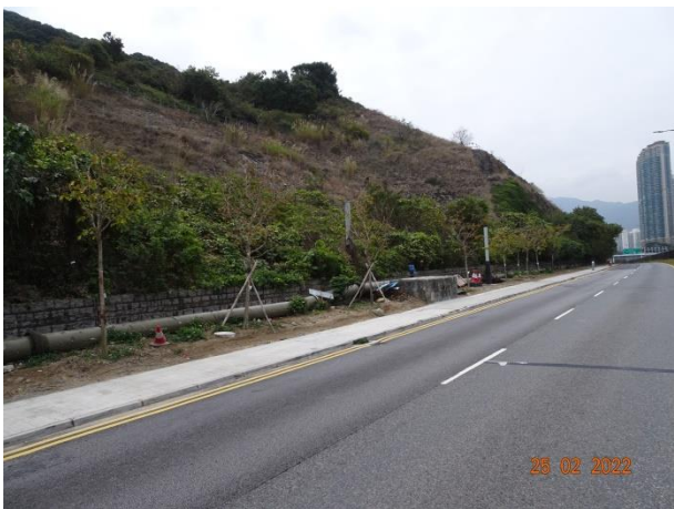
General View for Zone 1D
