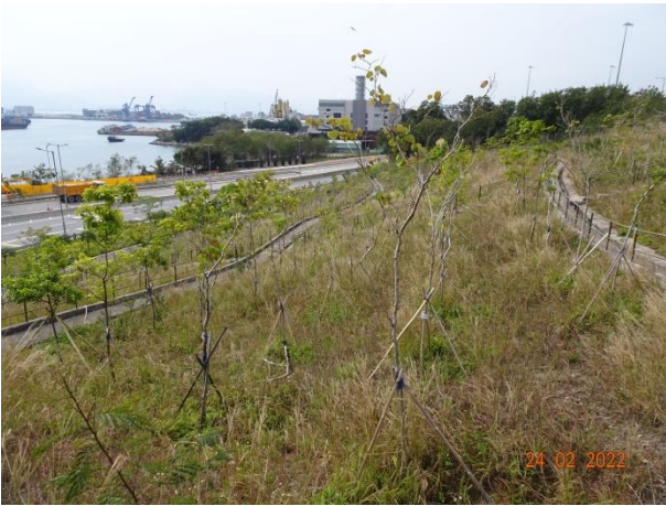
General View for Slope 5SE-D/C170
