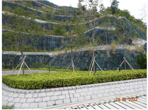
General View for Toe Planter
