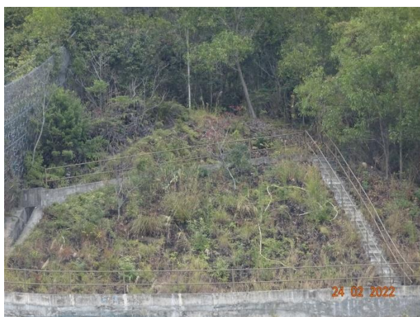
General View for Slope TP_D
