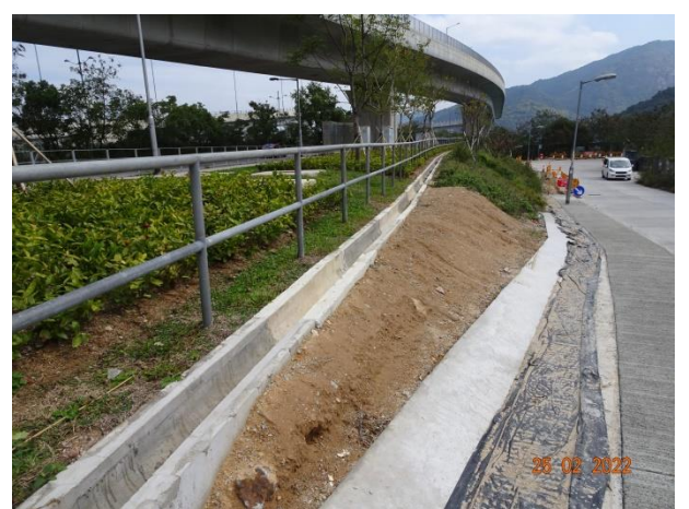
General View for Zone 1B
