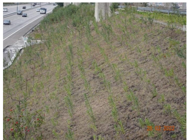
General View for Zone 3D
