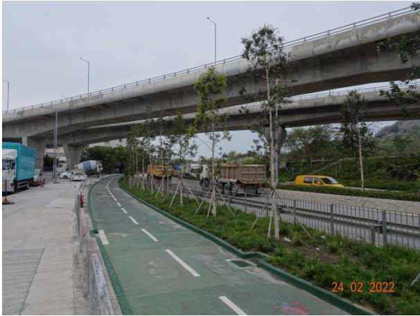
General View for Lung Mun Road
