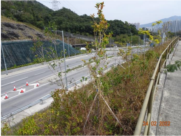
General View for Slope TP_C
