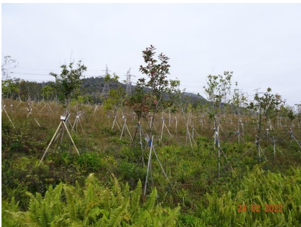
General View for Slope 5SE-D/C170
