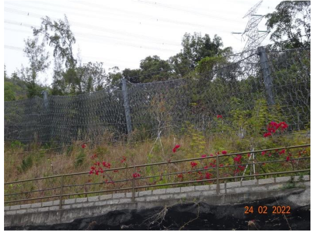
General View for Slope TP_A
