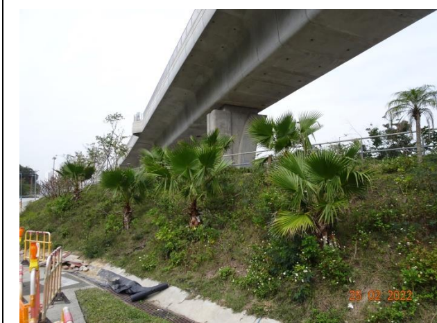
General View for Zone 1B
