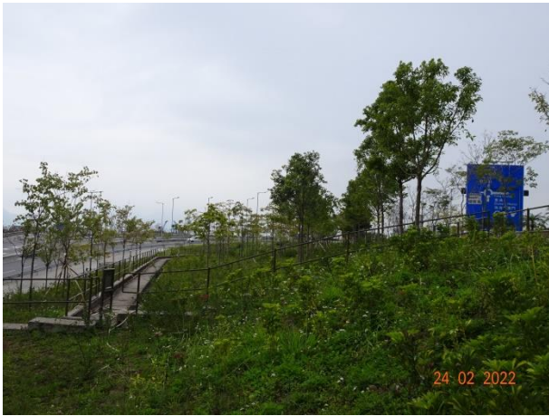
General View for Slope 5SE-D/C215
