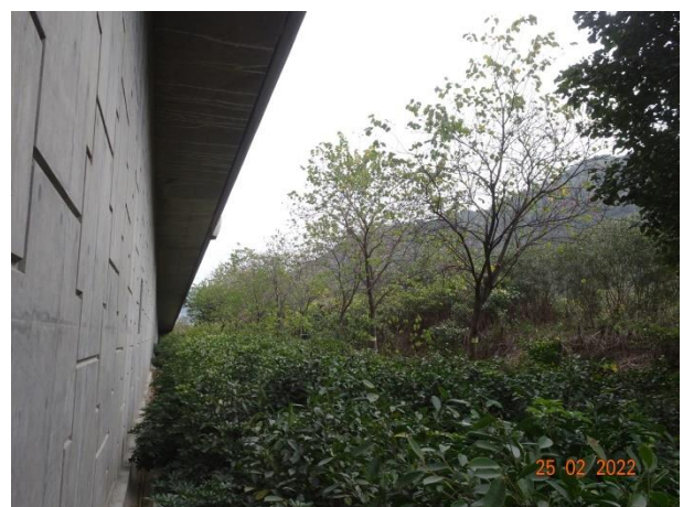
General View for Zone 3D
