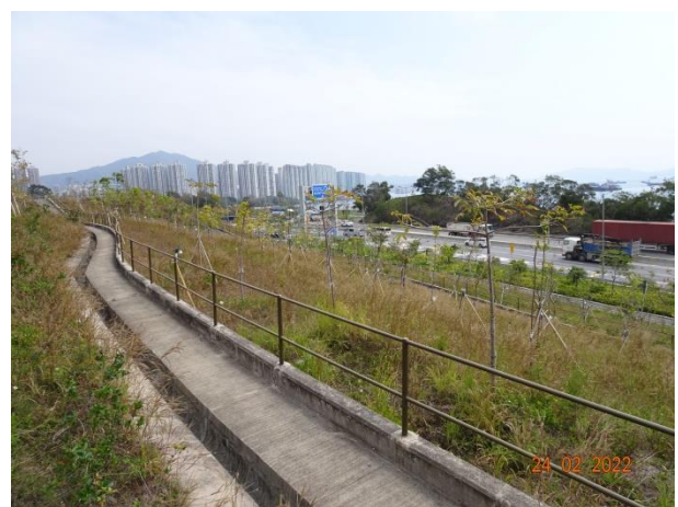
General View for Slope 5SE-D/C170
