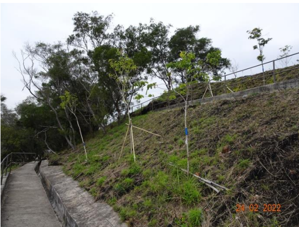
General View for Slope 5SE-D/C21
