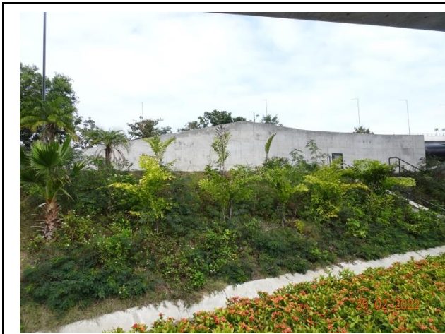
General View for Zone 1B
