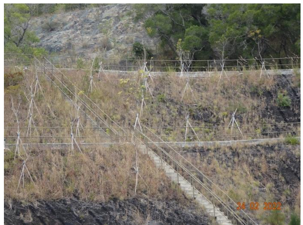
General View for Slope TP_B
