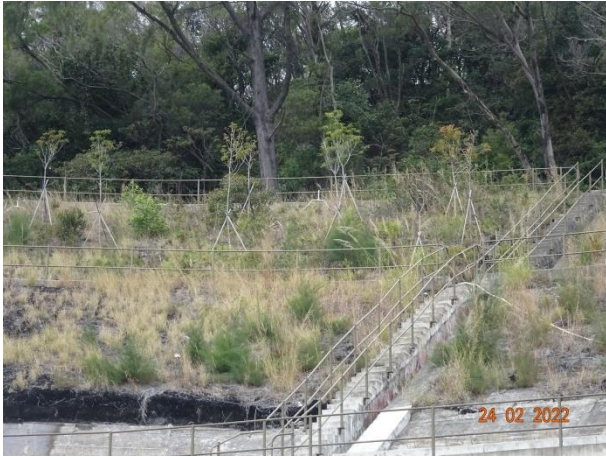
General View for Slope TP_A
