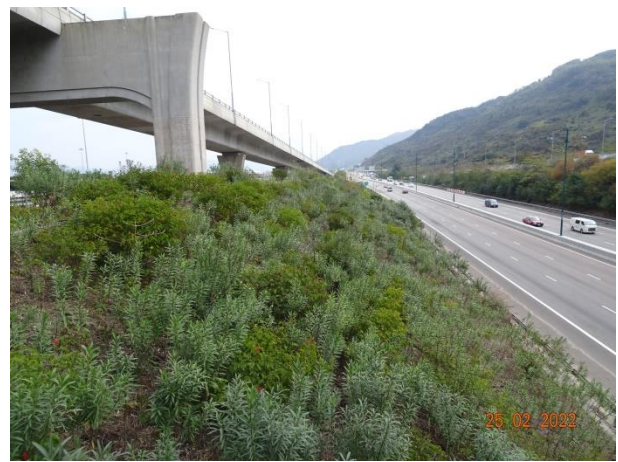
General View for Zone 3D
