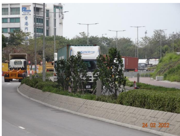
General View for Lung Mun Road
