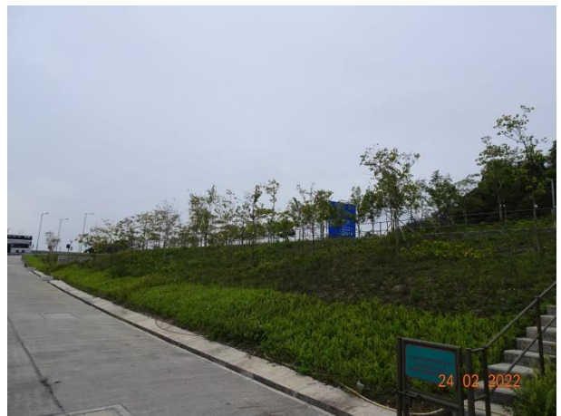
General View for Slope 5SE-D/C215
