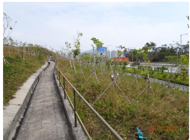
General View for Slope 5SE-D/C170
