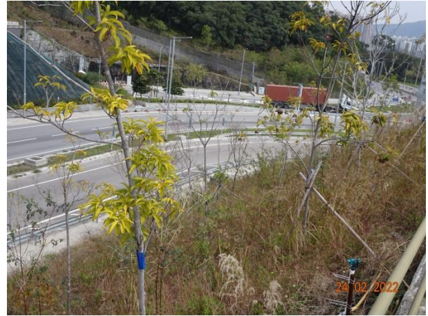
General View for Slope TP_C
