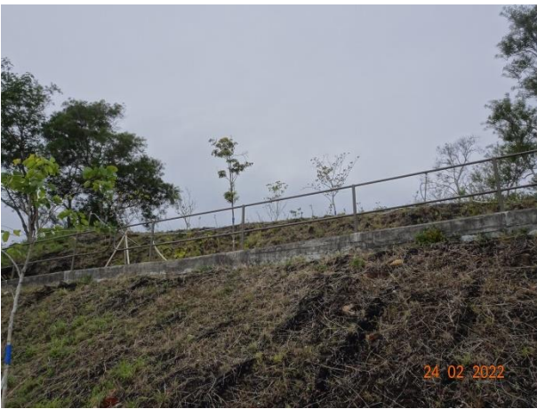
General View for Slope 5SE-D/C171
