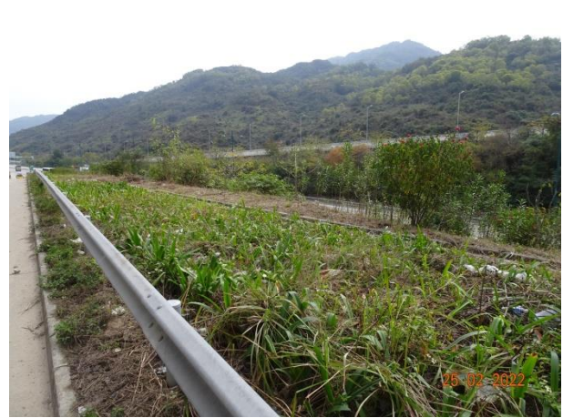
General View for Zone 3D
