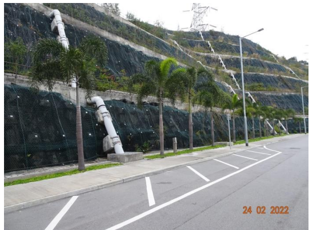
General View for Toe Planter
