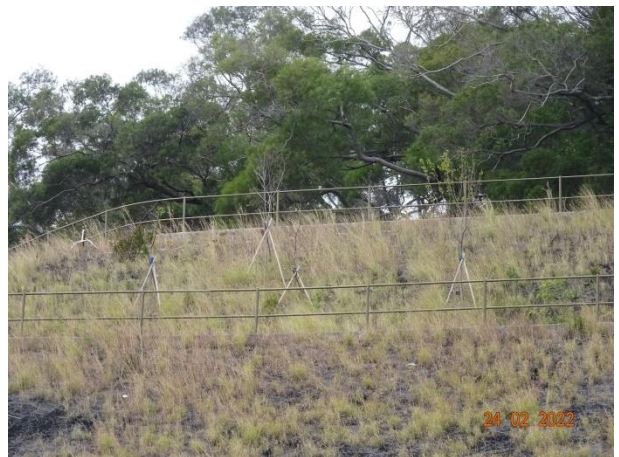
General View for Slope TP_A
