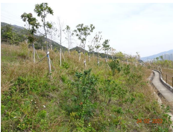
General View for Slope 5SE-D/C170
