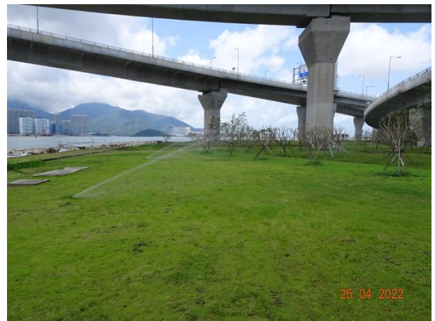
Watering system at Zone 2
