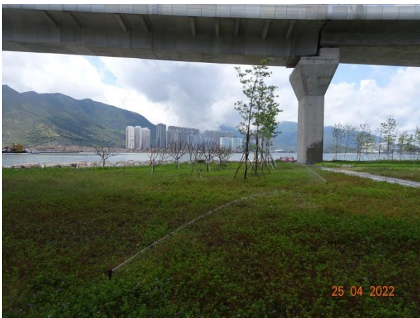
Watering system at Zone 2
