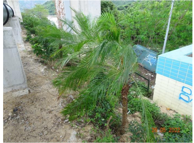
General View for Zone 1B
