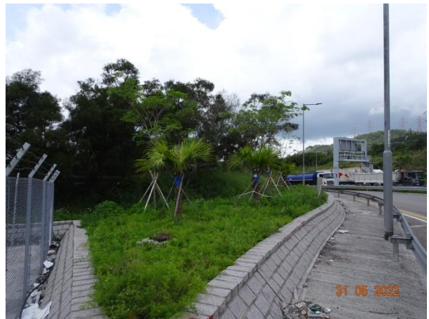
General View for Roundabout Area
