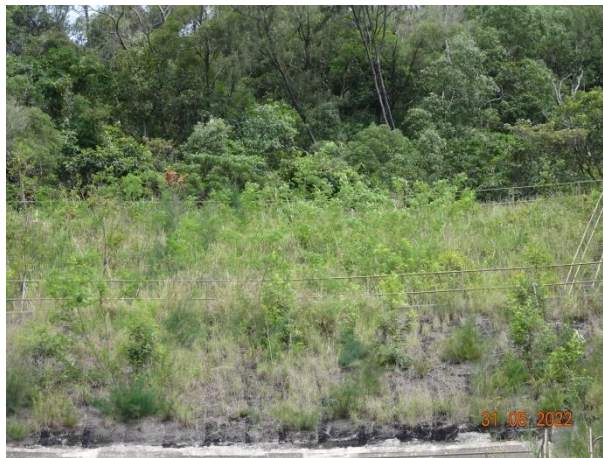
General View for Slope TP_A
