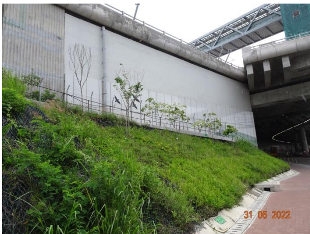
General View for Slope 5SE-D/C16
