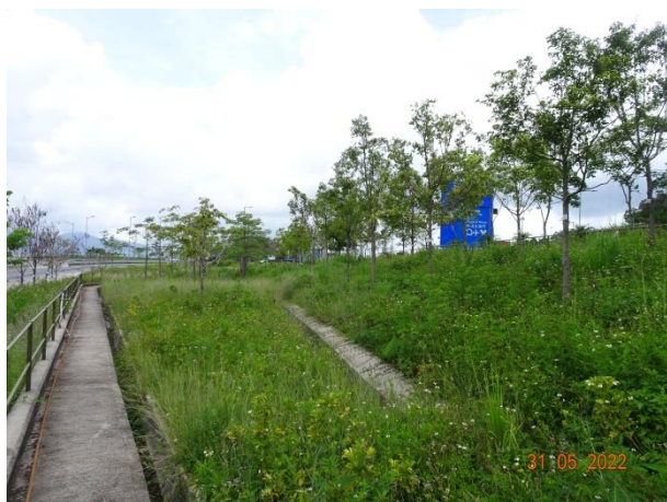
General View for Slope 5SE-D/C215
