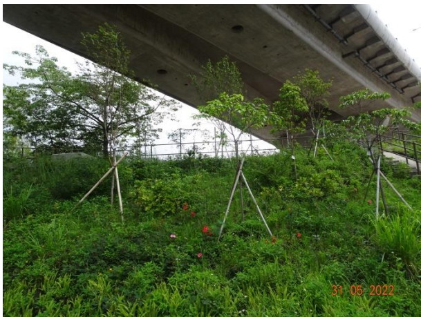
General View for Slope 5SE-D/C16
