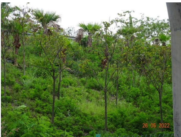
General View for Zone 3E
