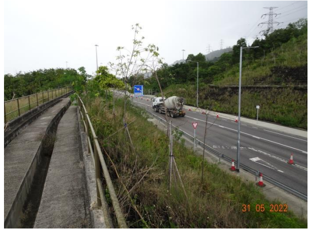
General View for Slope TP_C
