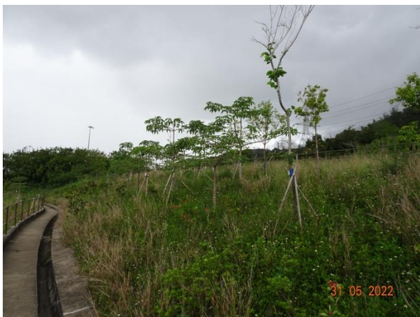
General View for Slope 5SE-D/C170
