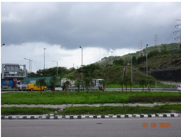
General View for Roundabout Area
