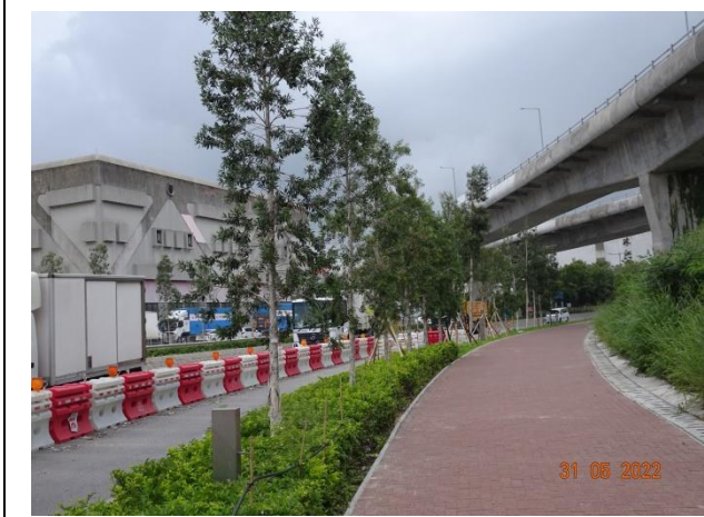
General View for Lung Mun Road
