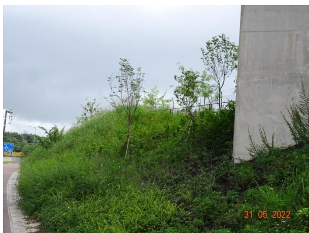
General View for Slope 5SE-D/C16
