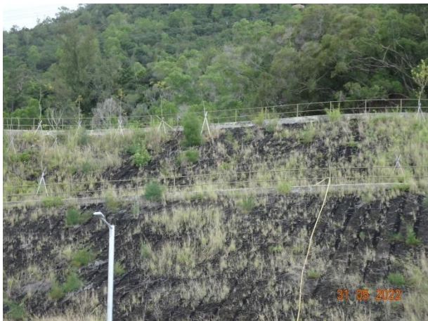
General View for Slope TP_B
