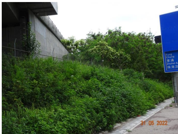
General View for Slope 5SE-D/C18
