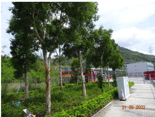
General View for Toll Plaza Interchange
