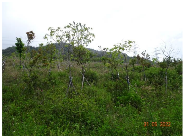
General View for Slope 5SE-D/C170
