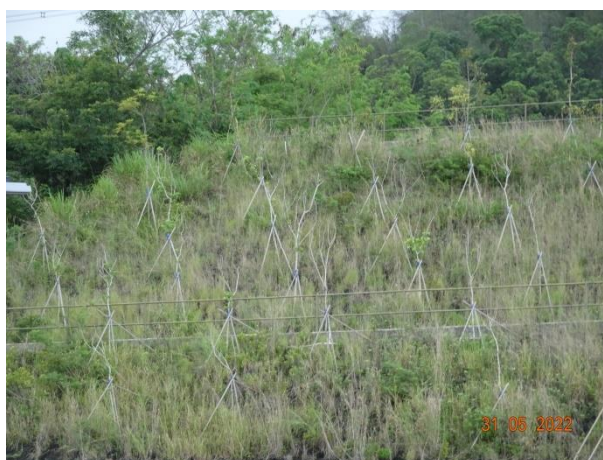
General View for Slope TP_B
