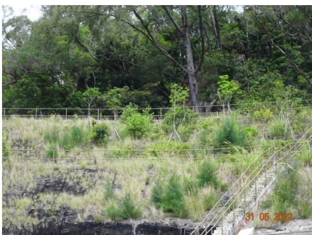
General View for Slope TP_A
