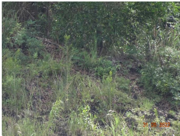
General View for Slope TP_D
