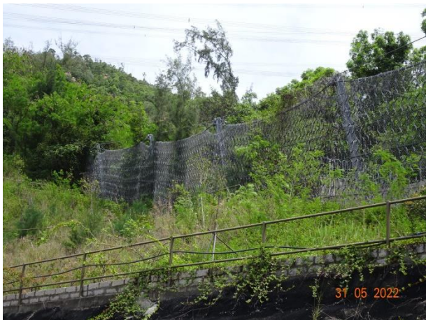
General View for Slope TP_A
