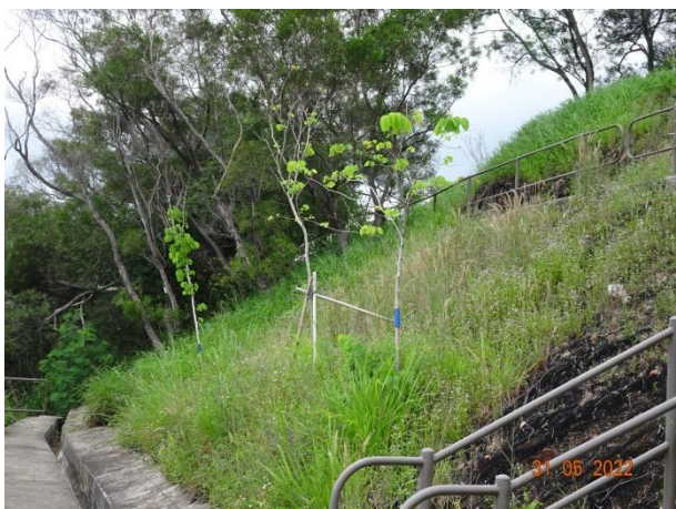
General View for Slope 5SE-D/C21
