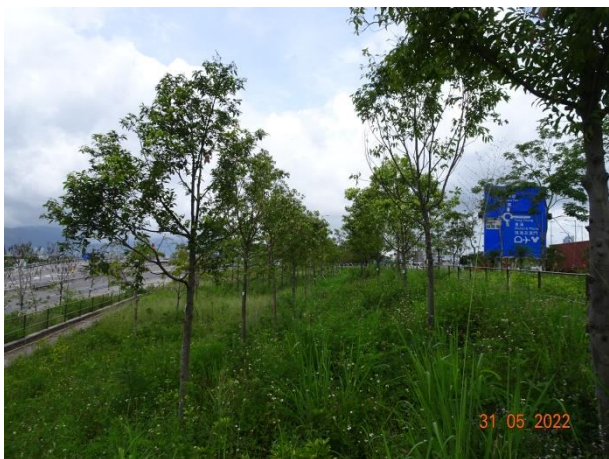
General View for Slope 5SE-D/C215
