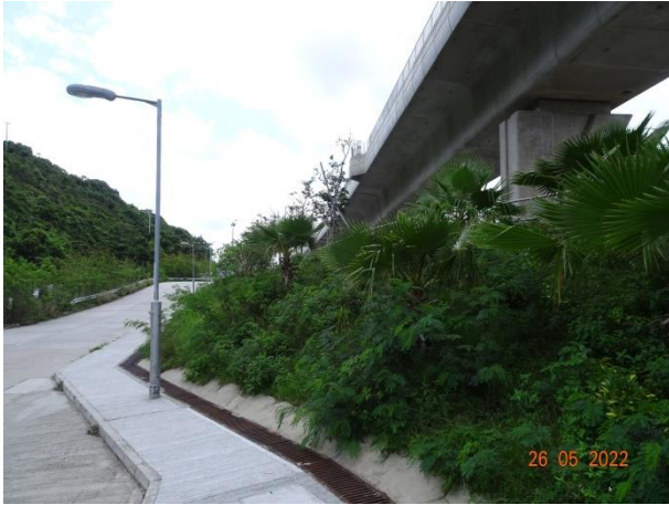
General View for Zone 1B
