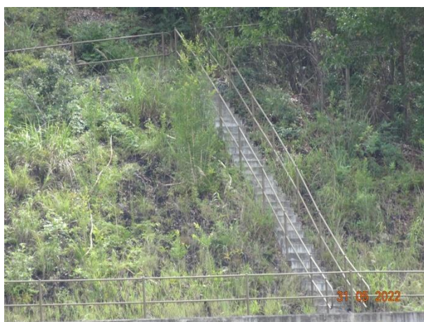
General View for Slope TP_D
