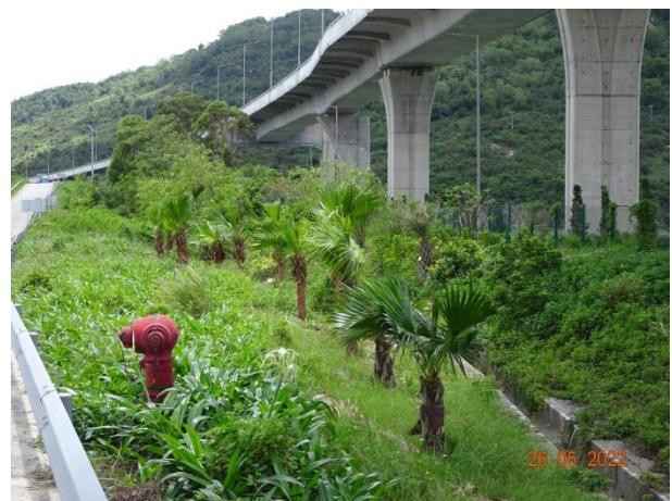
General View for Zone 3E
