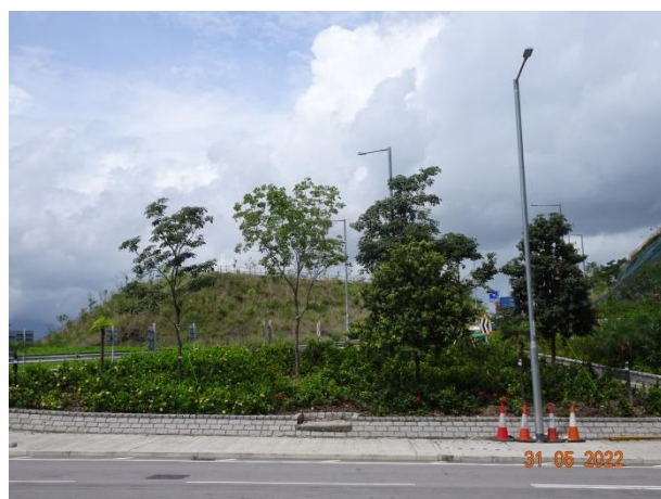
General View for planter near the Tunnel
