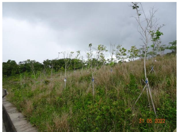
General View for Slope 5SE-D/C170
