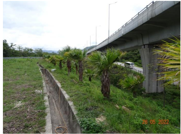
General View for Zone 3E
