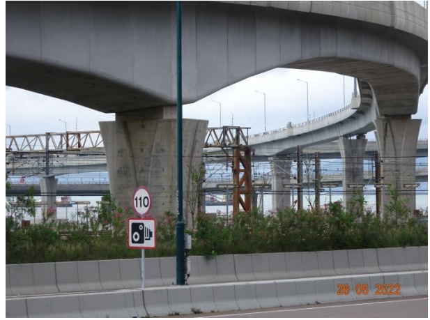
General View for Zone 3B
