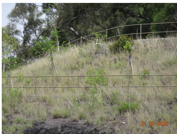
General View for Slope TP_A
