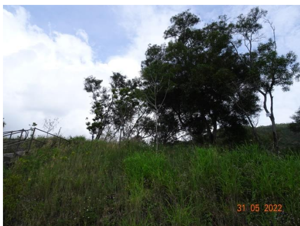
General View for Slope 5SE-D/C21
