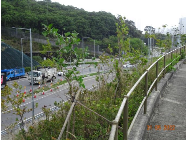
General View for Slope TP_C
