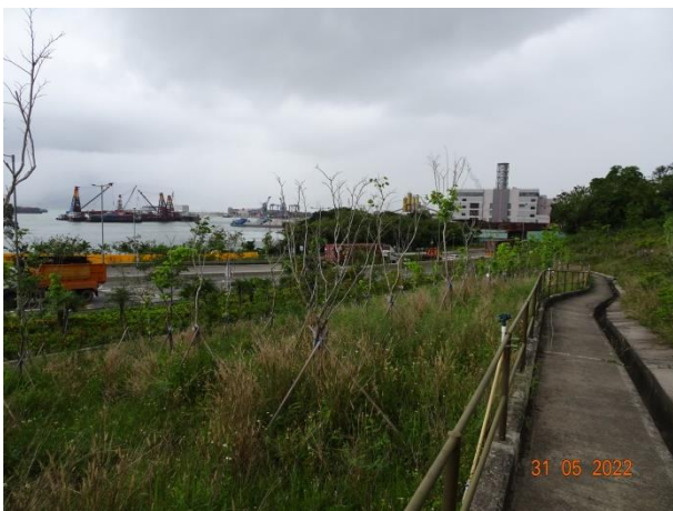
General View for Slope 5SE-D/C170
