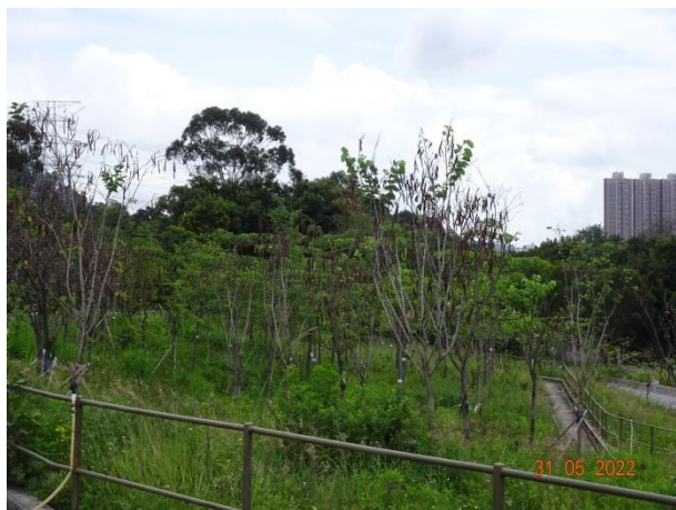
General View for Slope 5SE-D/C215
