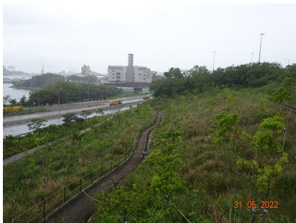
General View for Slope 5SE-D/C170
