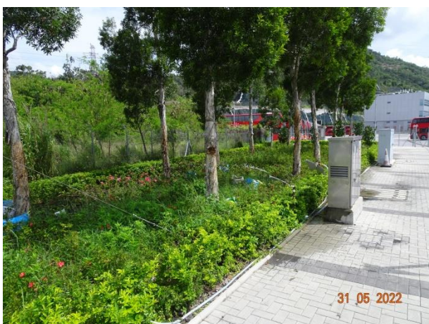
Watering system at Toll Plaza Interchange
