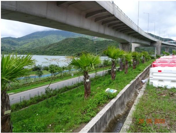
General View for Zone 3E
