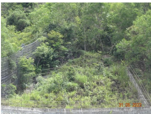
General View for Slope TP_D
