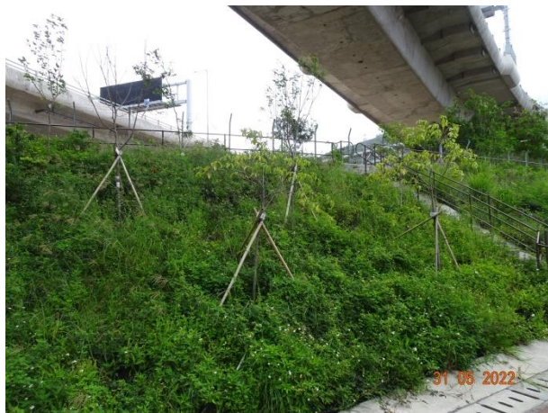
General View for Slope 5SE-D/C16
