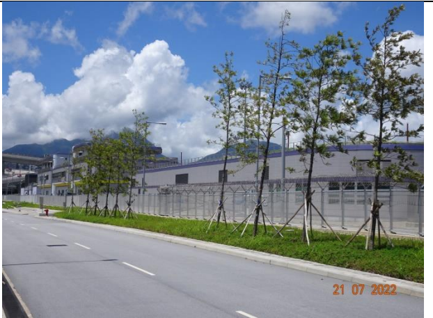
General View for Zone 6
