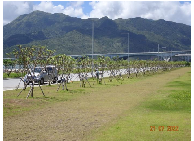
General View for Zone 6
