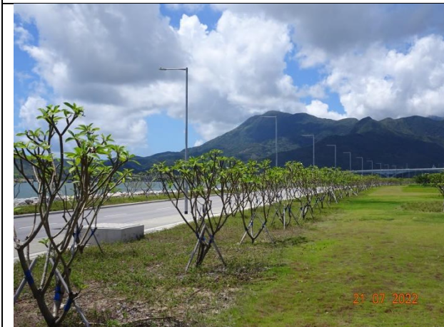
General View for Zone 6
