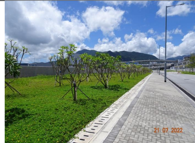
General View for Zone 6
