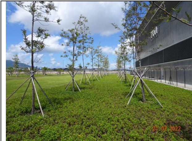
General View for Zone 6
