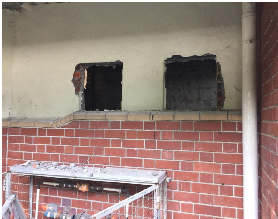
Maintenance works are carried out near ASR10.
