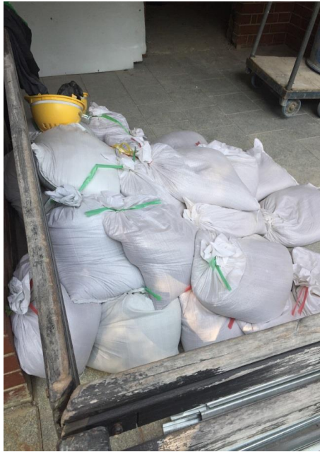
Dusty materials are placed on the ground near ASR10.
