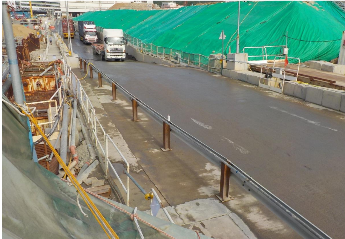
Exposed soil are covered by tarpaulin sheets. (Works Area Portion N-A)
