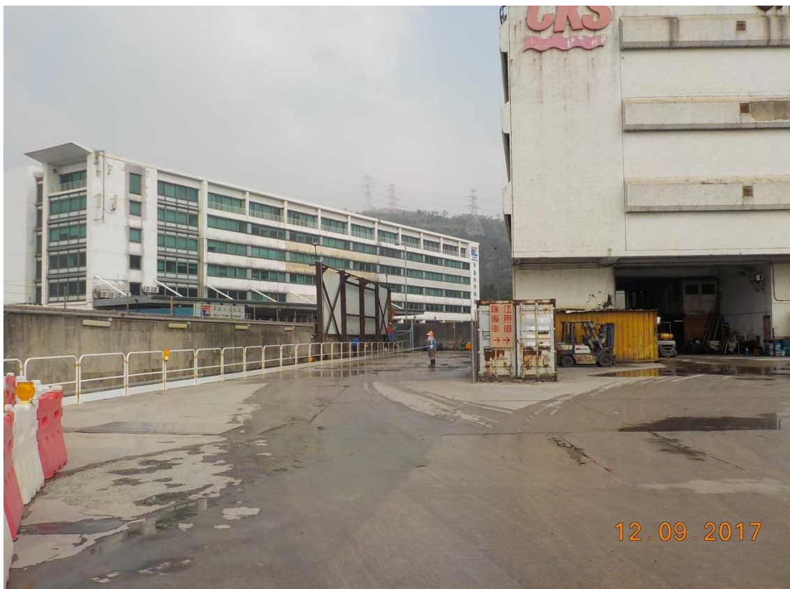
Water spraying was applied frequently during dry conditions. (Works Area Portion N-A)
