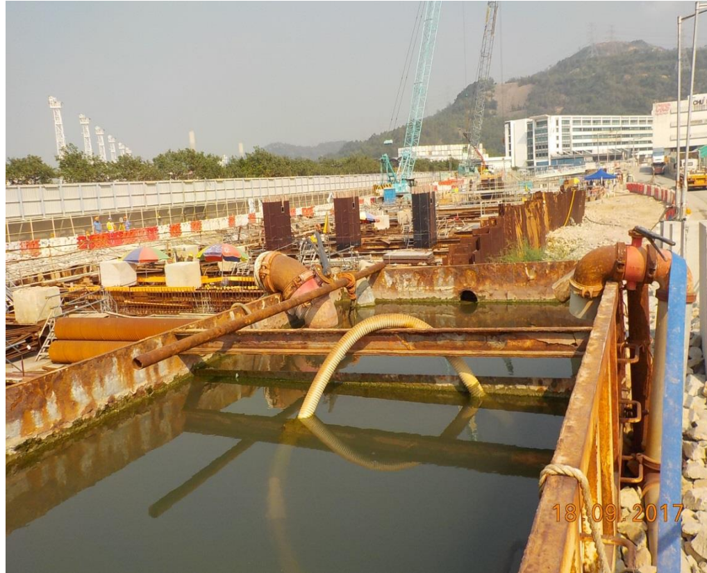
Box Culvert Extension. (Works Area Portion N-A)
