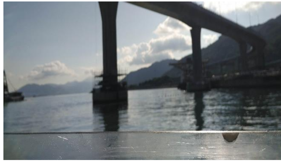
Photo 5 - Mid-Flood at SR4a on 7 September 2018
