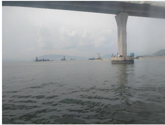
Photo 4 - Mid-Flood at SR4a on 05 September 2018
