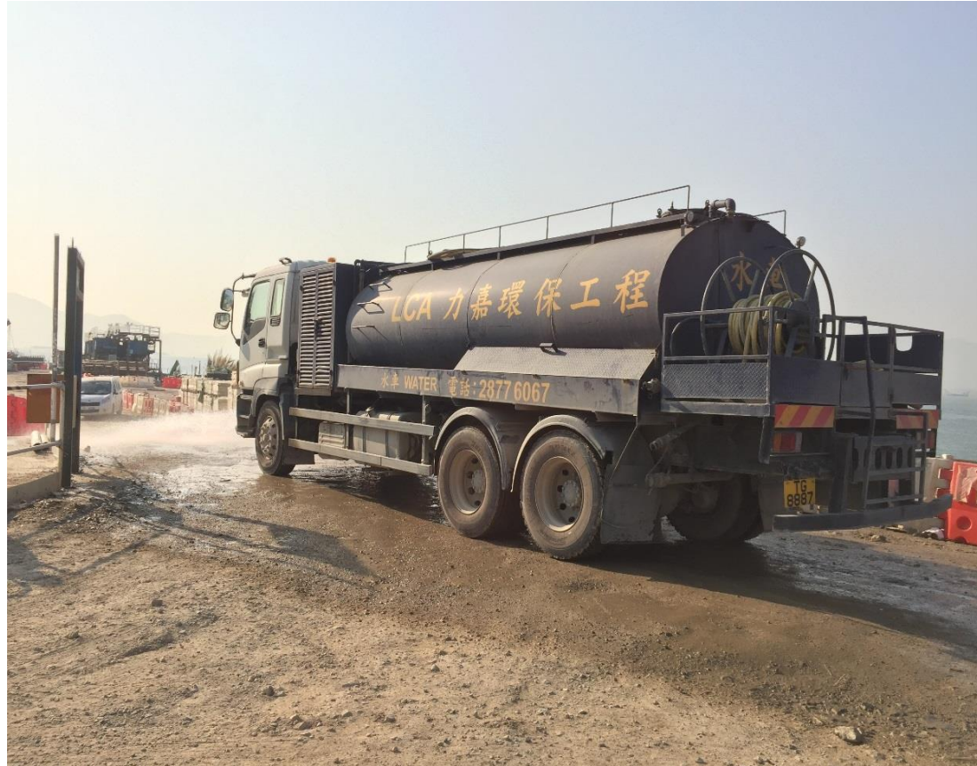
Water truck is used for water spraying at works area. (Works Area Portion N-C)
