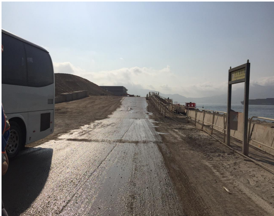
Water spraying was applied on the main haul road. (Works Area Portion N-C)
