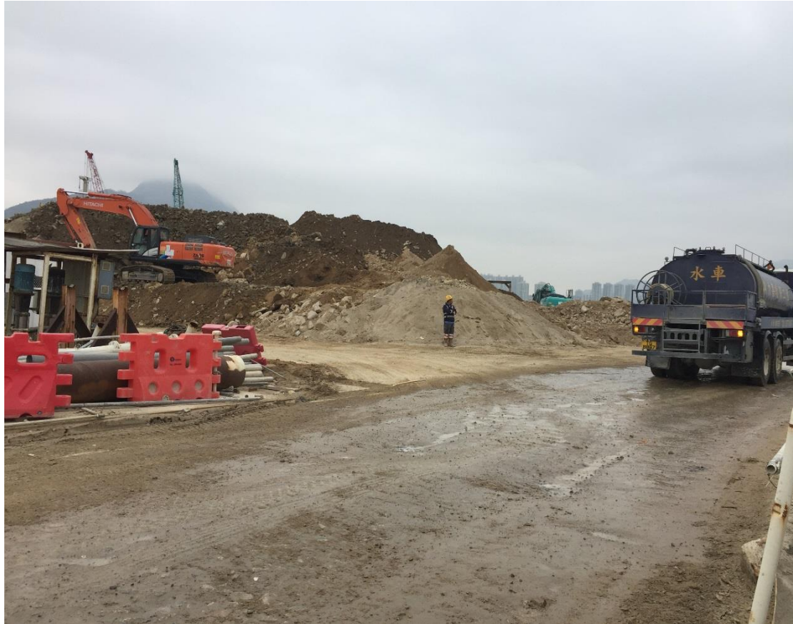
Water truck is used for water spraying at the works area. (Works Area Portion N-C)
