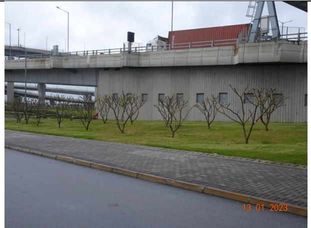
General View for Zone 6
