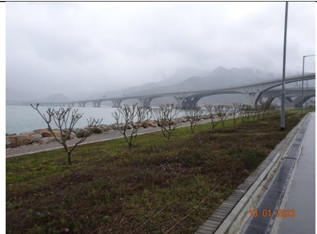
General View for Zone 6
