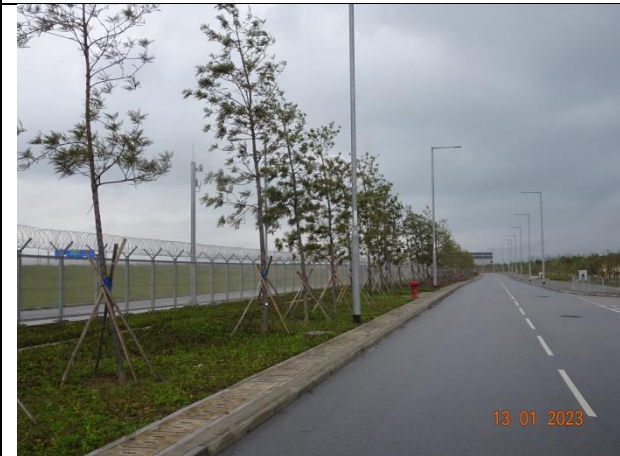
General View for Zone 6
