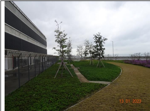
General View for Zone 6
