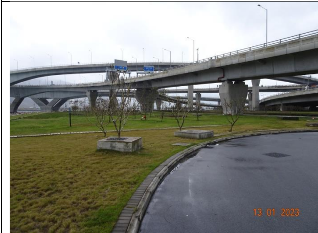
General View for Zone 6
