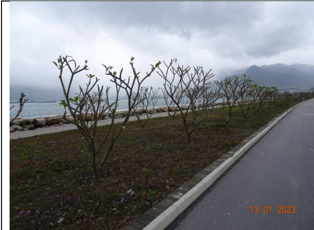
General View for Zone 6
