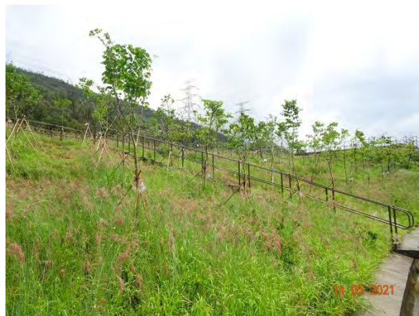
General View for Slope 5SE-D/C170
