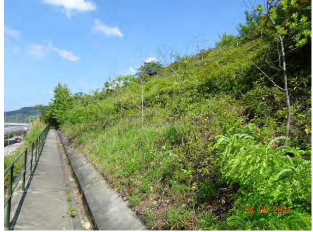
General View for Zone 4
