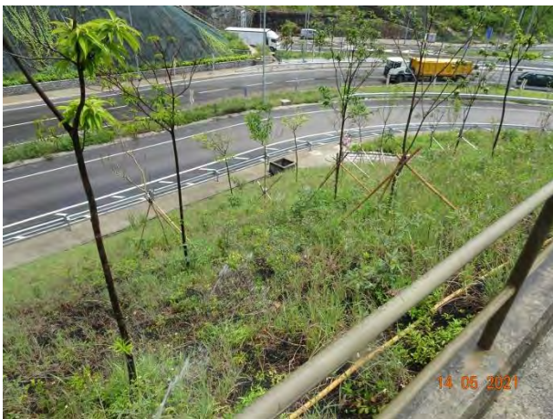
General View for Slope TP_C
