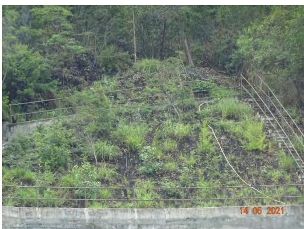
General View for Slope TP_D
