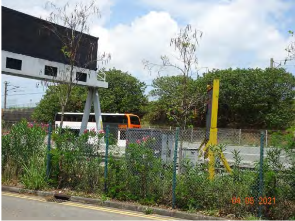
General View for Zone 3F
