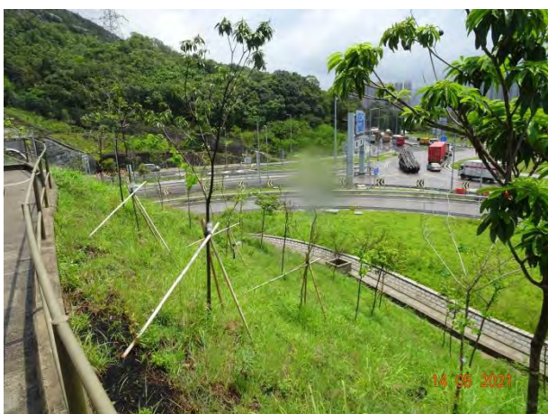
General View for Slope 5SE-D/C170
