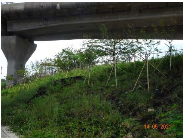
General View for Slope 5SE-D/C16
