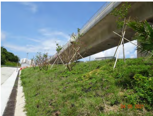
General View for Zone 1B
