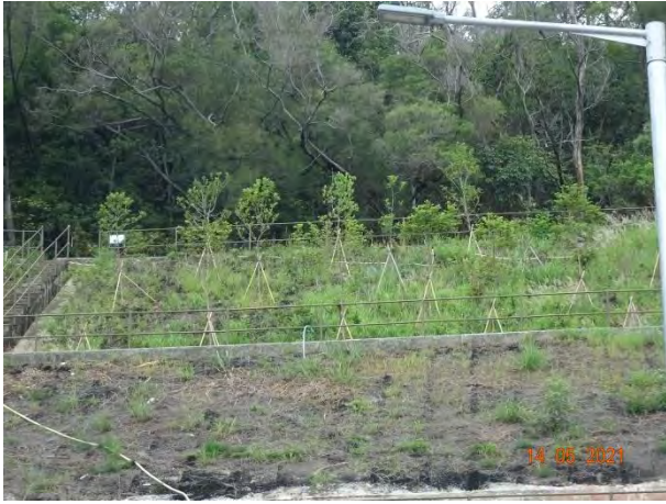
General View for Slope TP_A
