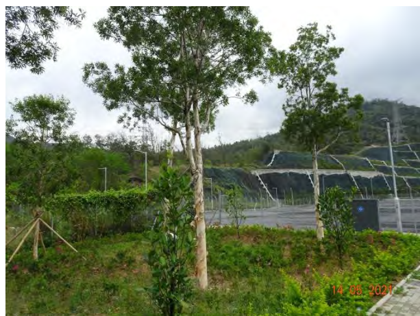
General View for Toll Plaza
