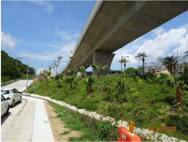
General View for Zone 1B
