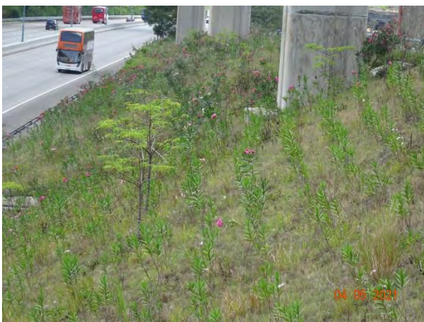
General View for Zone 3D
