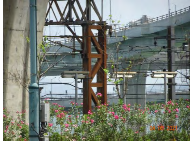
General View for Zone 3B
