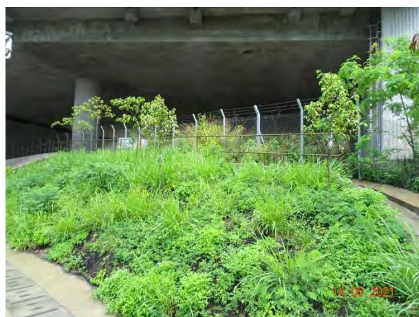
General View for Slope 5SE-D/C18
