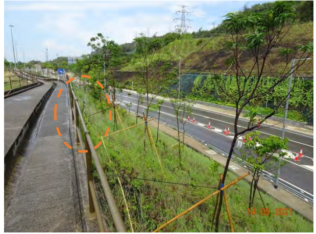
Watering system at Slope TP_C
