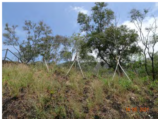
General View for Slope 5SE-D/C21
