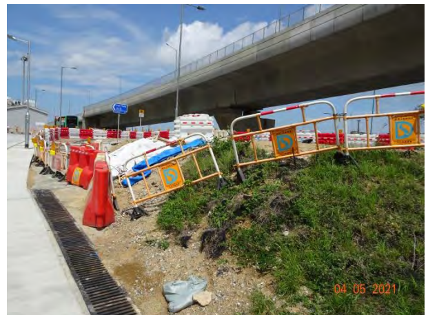
General View for Zone 1B
