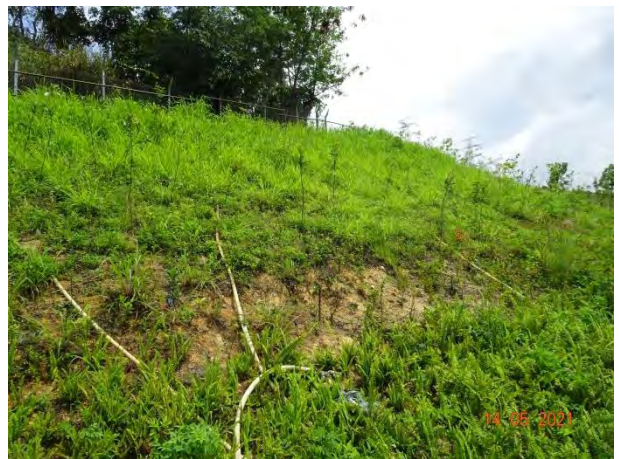
General View for Slope 5SE-D/C170
