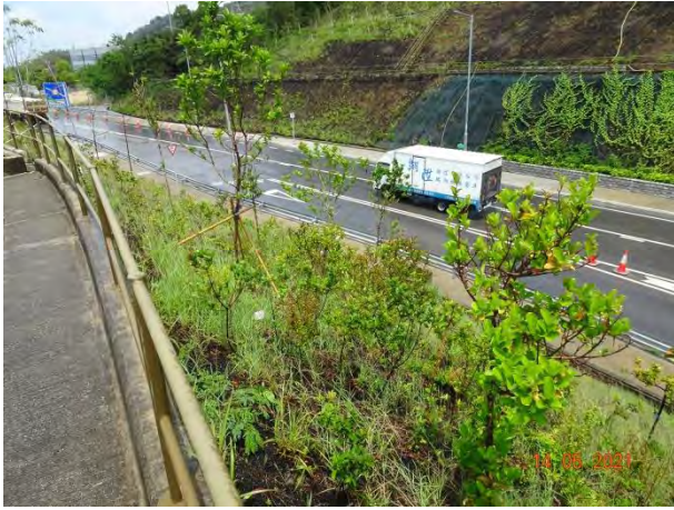
General View for Slope TP_C
