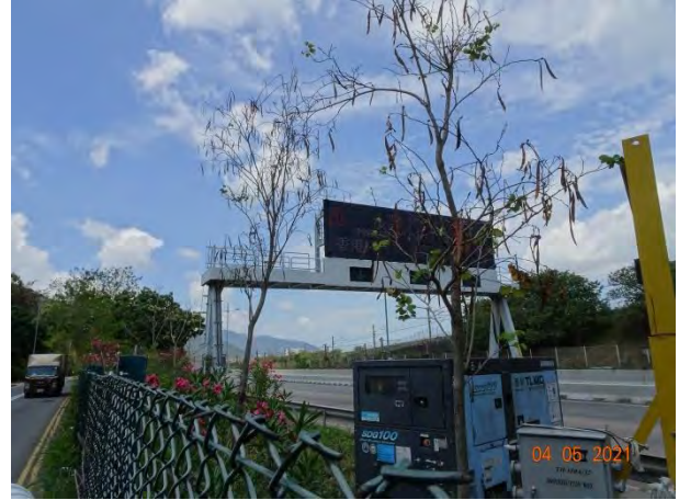
General View for Zone 3F
