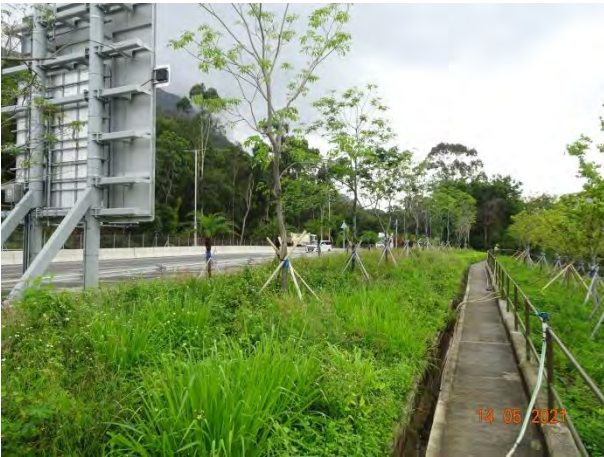
General View for Roundabout Area
