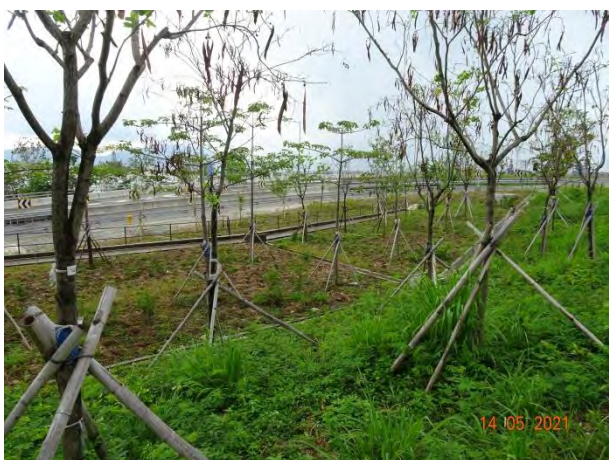
General View for Slope 5SE-D/C215
