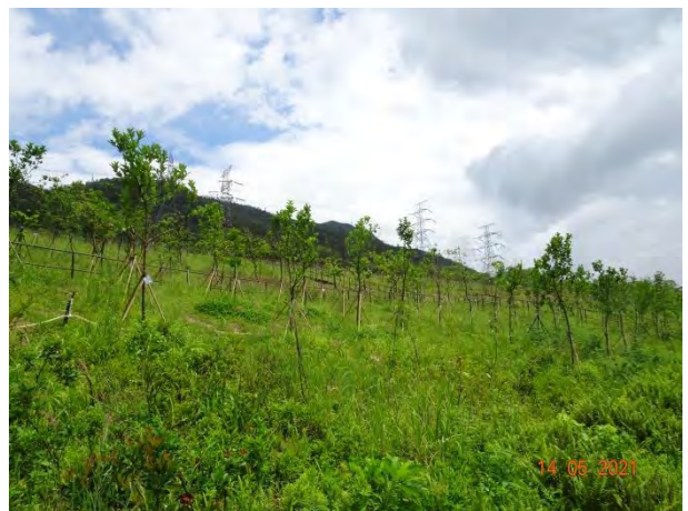
General View for Slope 5SE-D/C170
