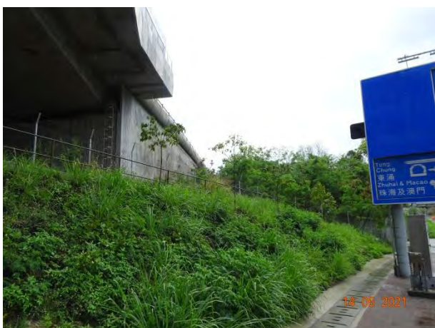
General View for Slope 5SE-D/C18
