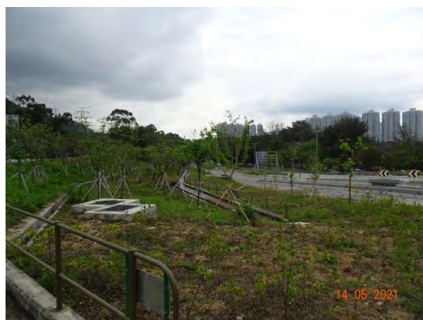
General View for Slope 5SE-D/C215
