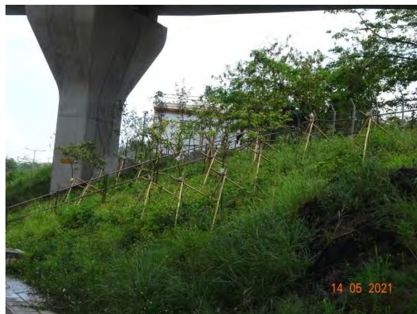
General View for Slope 5SE-D/C16
