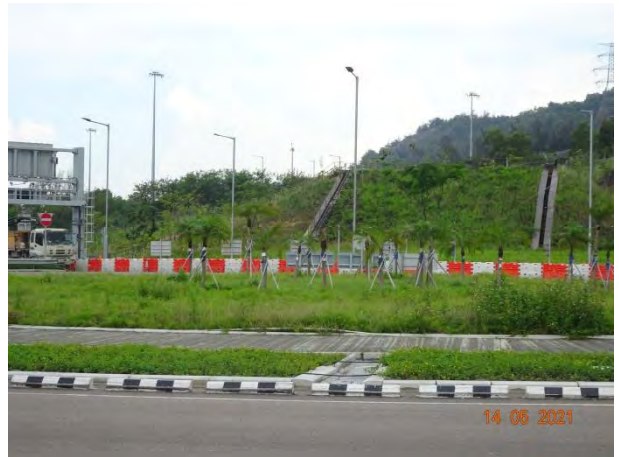
General View for Roundabout Area
