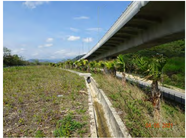
General View for Zone 3E
