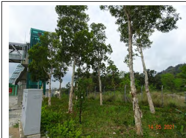
General View for Toll Plaza
