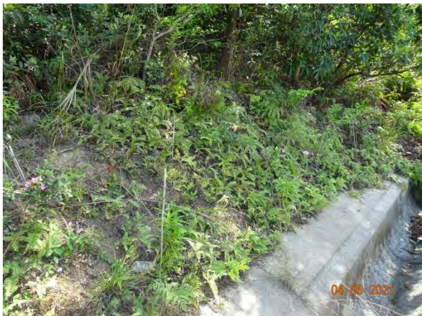
General View for Zone 4
