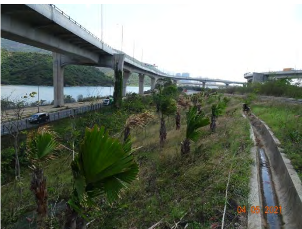
General View for Zone 3E
