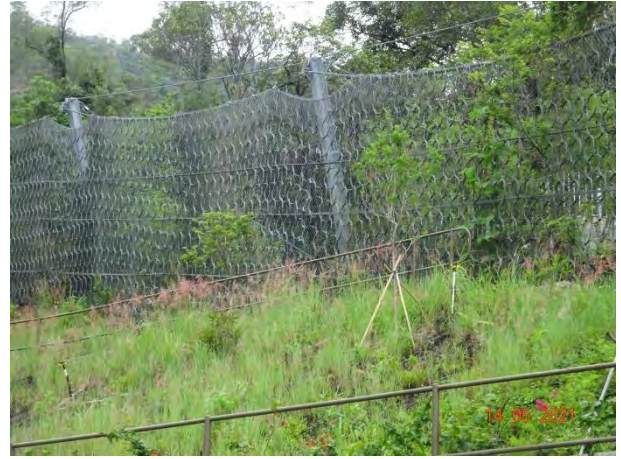
General View for Slope TP_A
