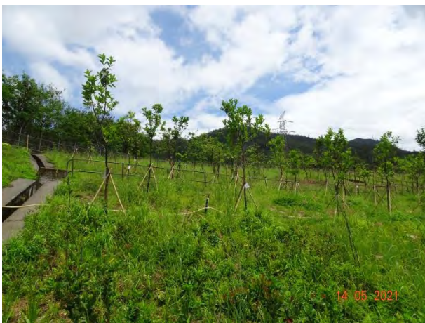
General View for Slope 5SE-D/C170
