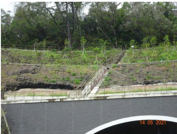
General View for Slope TP_A
