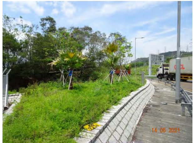
General View for Roundabout Area
