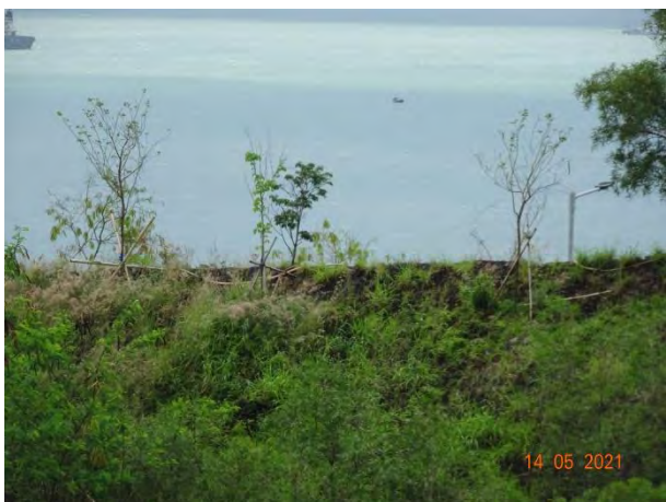
General View for Slope 5SE-D/C171
