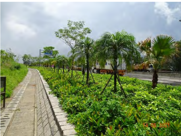
General View for Roundabout Area
