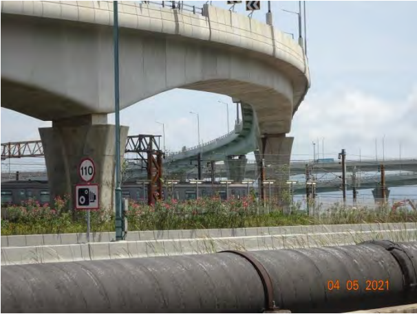
General View for Zone 3B
