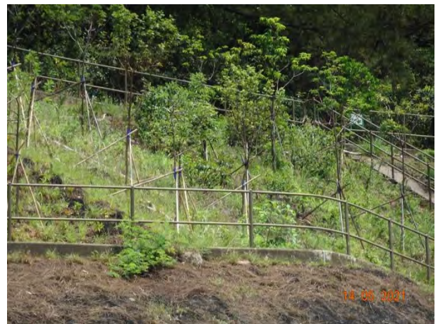
General View for Slope TP_A
