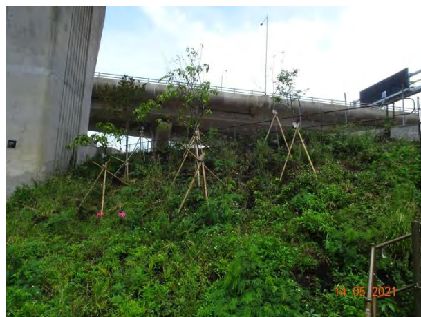
General View for Slope 5SE-D/C16
