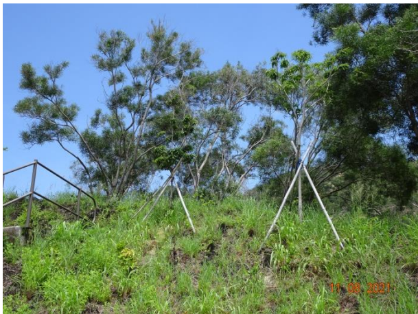
General View for Slope 5SE-D/C21
