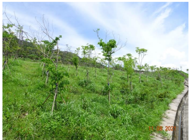
General View for Slope 5SE-D/C170
