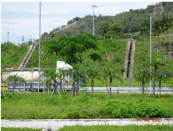
General View for Roundabout Area
