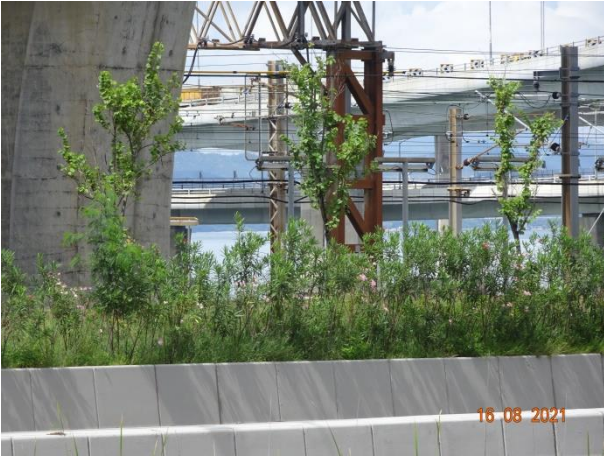
General View for Zone 3B
