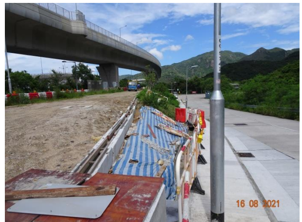
General View for Zone 1B
