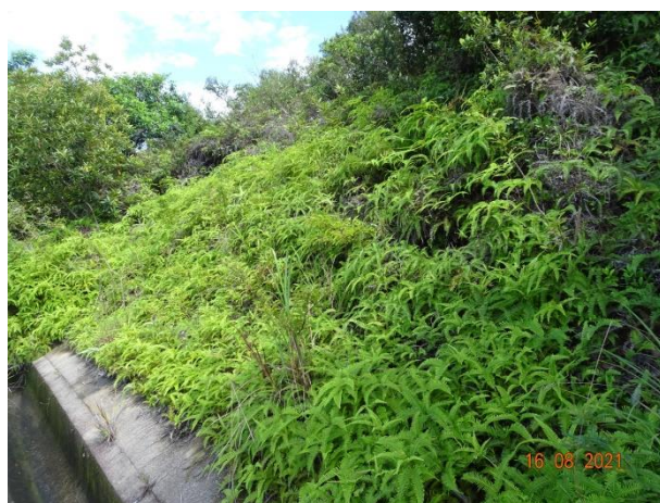
General View for Zone 4
