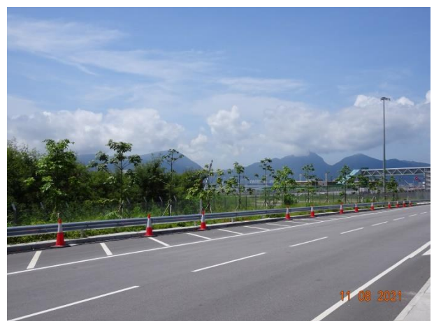
General View for Toe Planter
