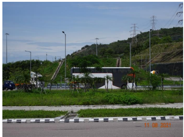
General View for Roundabout Area
