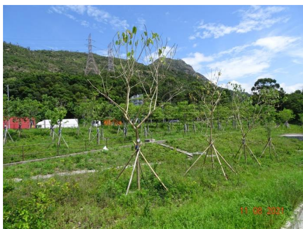
General View for Slope 5SE-D/C215
