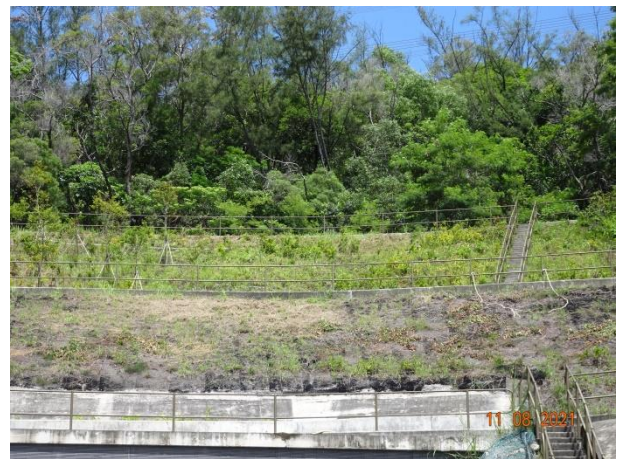
General View for Slope TP_A
