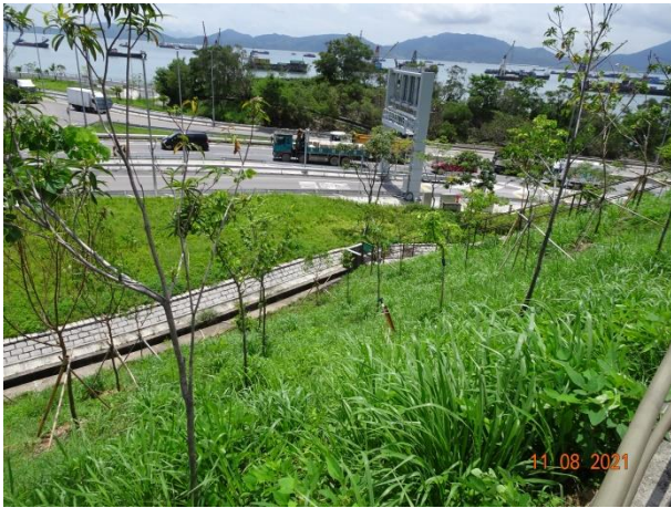
General View for Slope 5SE-D/C170
