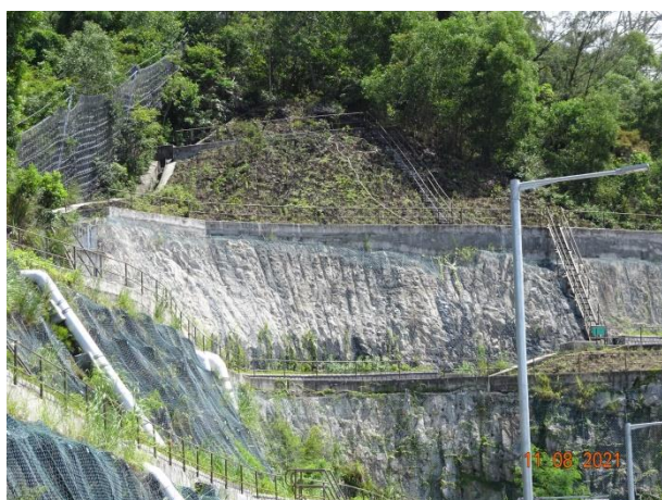
General View for Slope TP_D
