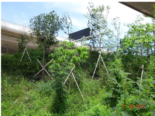
General View for Slope 5SE-D/C16
