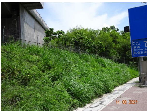
General View for Slope 5SE-D/C18
