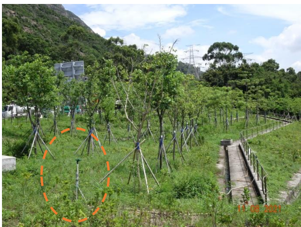
Watering system at Slope 5SE-D/C215
