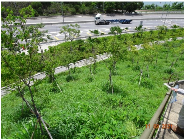
General View for Slope 5SE-D/C170
