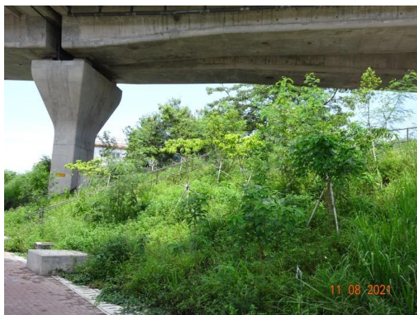
General View for Slope 5SE-D/C16
