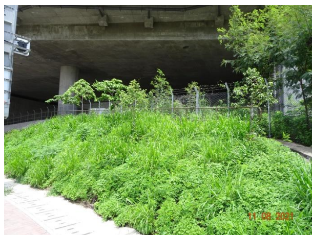
General View for Slope 5SE-D/C18
