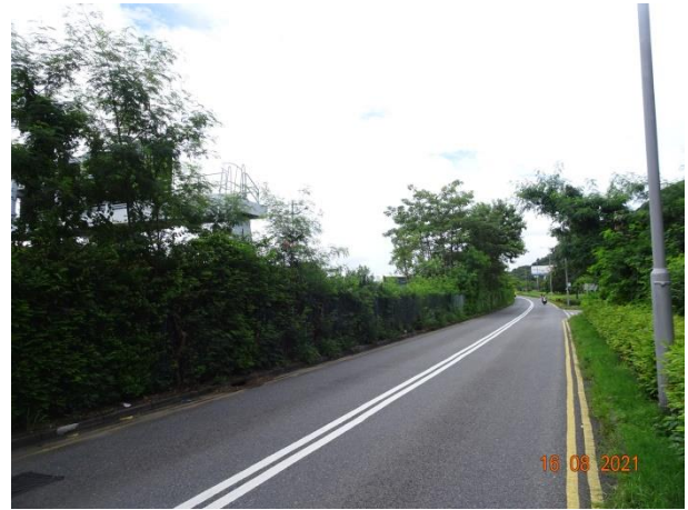
General View for Zone 3F
