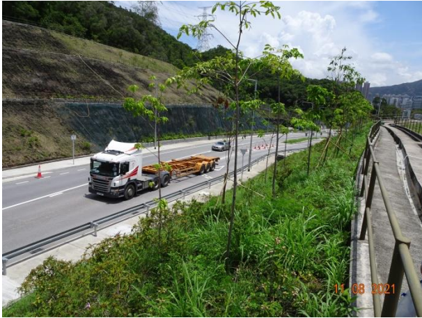
General View for Slope TP_C
