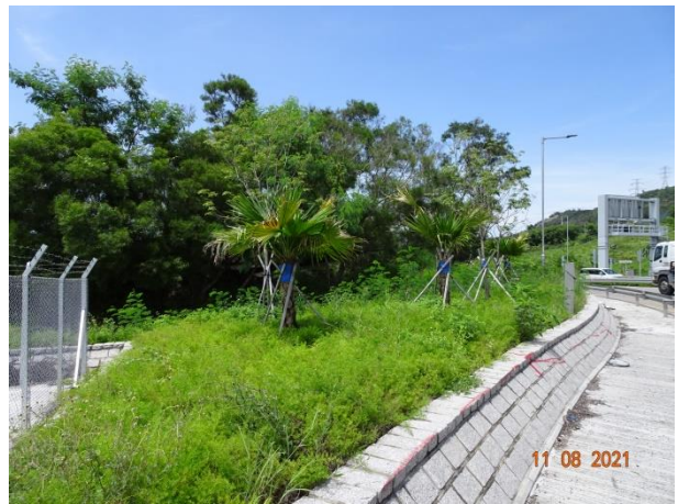
General View for Roundabout Area
