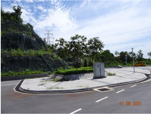
General View for Toe Planter
