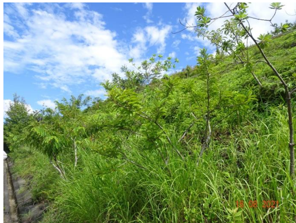
General View for Zone 4
