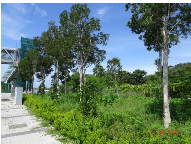
General View for Toll Plaza
