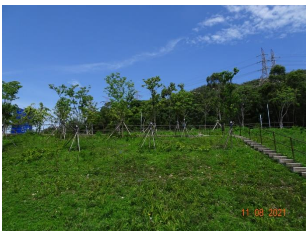
General View for Slope 5SE-D/C215
