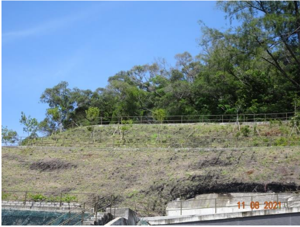
General View for Slope TP_A
