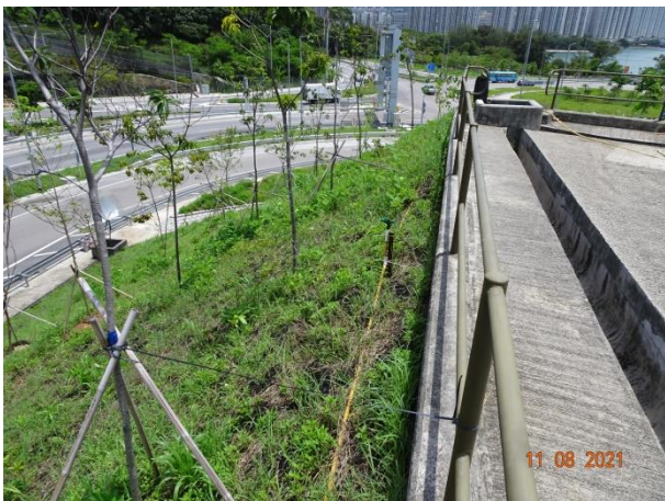
General View for Slope TP_C
