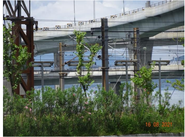
General View for Zone 3B
