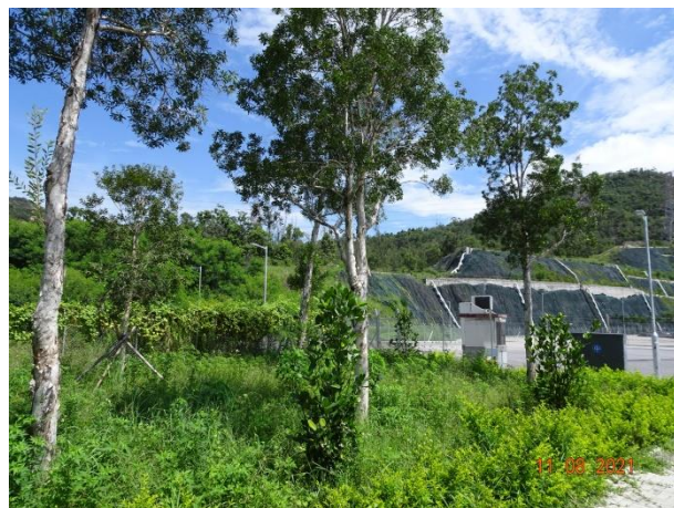
General View for Toll Plaza
