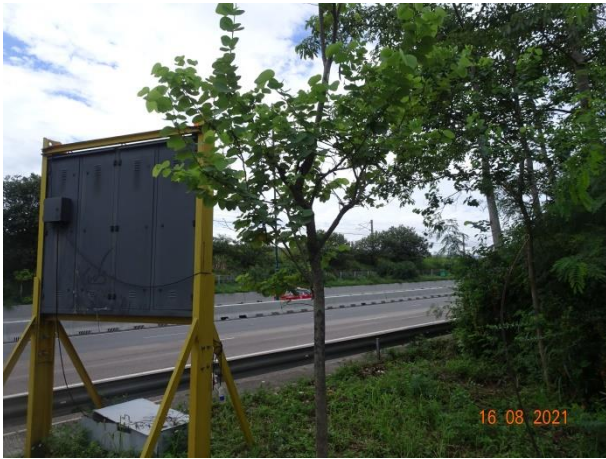
General View for Zone 3F
