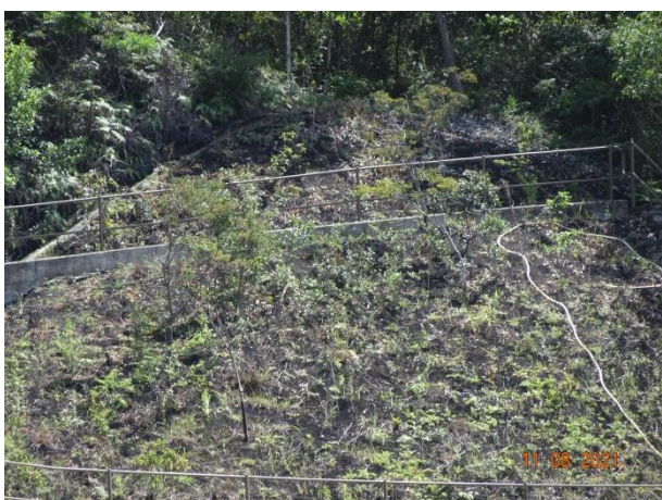
General View for Slope TP_D
