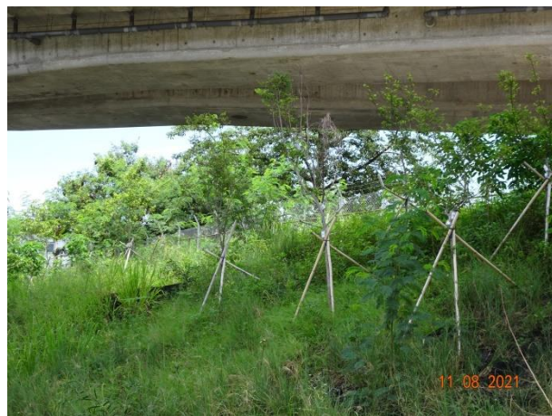
General View for Slope 5SE-D/C16
