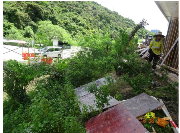
General View for Zone 1B
