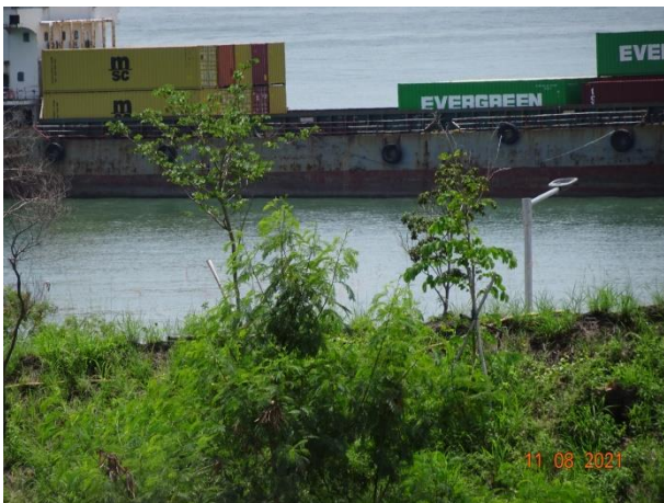
General View for Slope 5SE-D/C171
