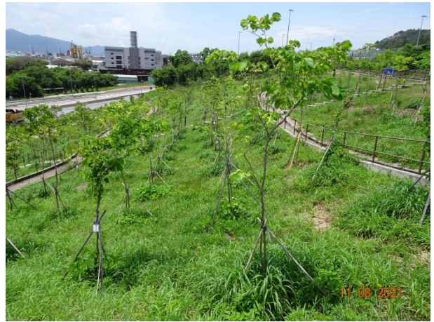
General View for Slope 5SE-D/C170
