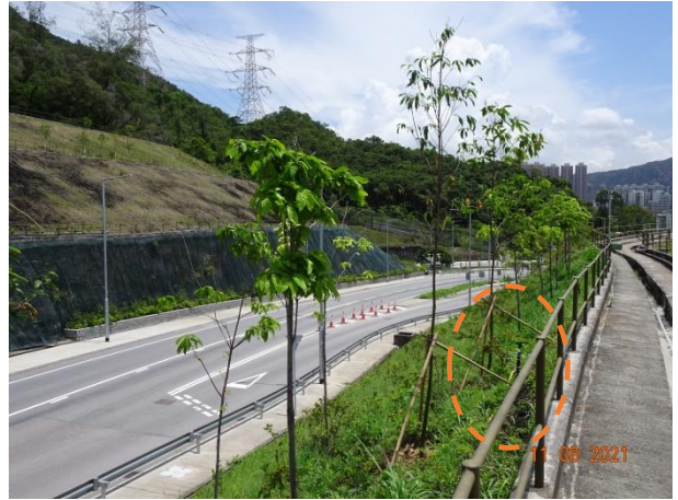
Watering system at Slope TP_C
