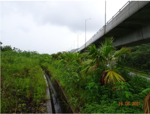
General View for Zone 3E
