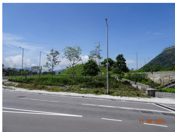
General View for planter near the Tunnel
