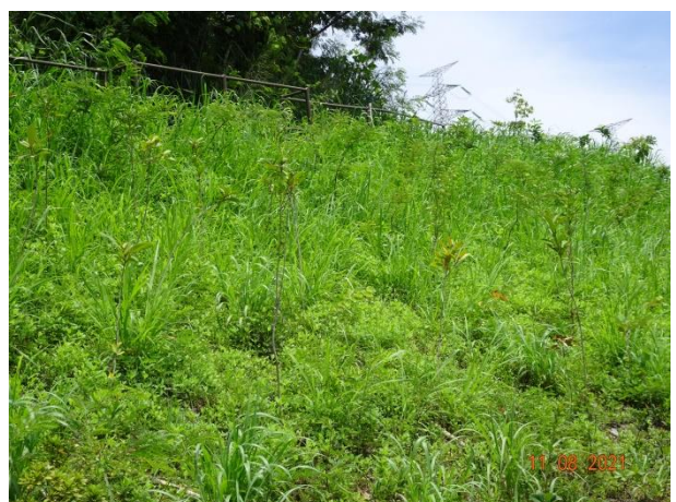
General View for Slope 5SE-D/C170
