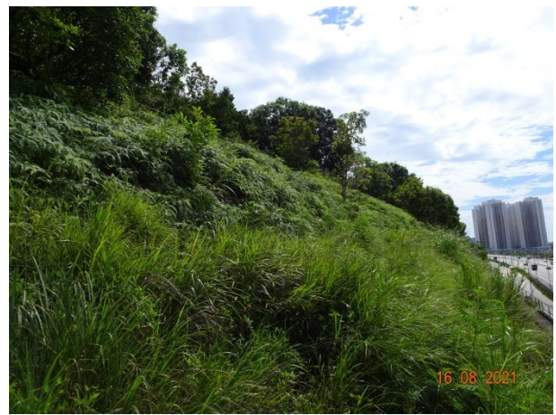
General View for Zone 4
