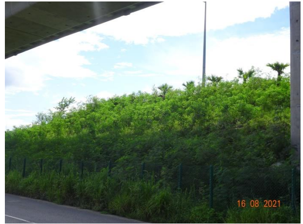
General View for Zone 3E
