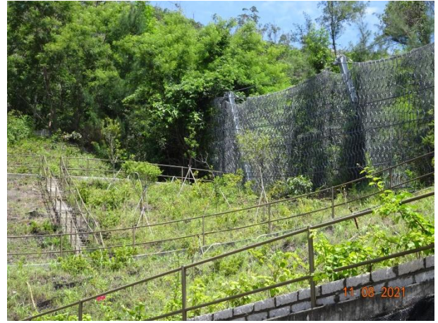
General View for Slope TP_A
