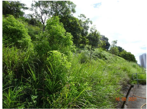
General View for Zone 4
