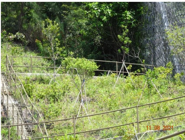
General View for Slope TP_A
