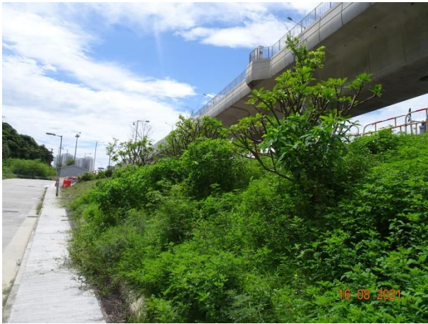
General View for Zone 1B
