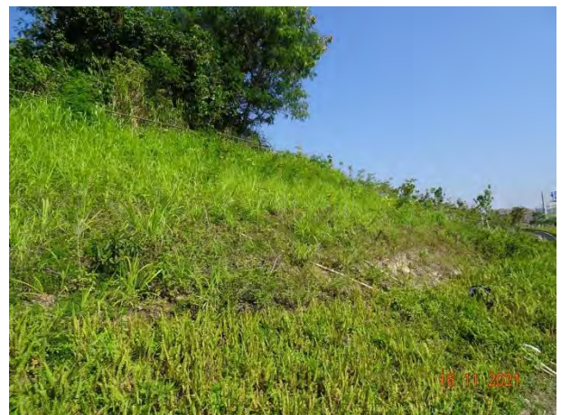
General View for Slope 5SE-D/C170
