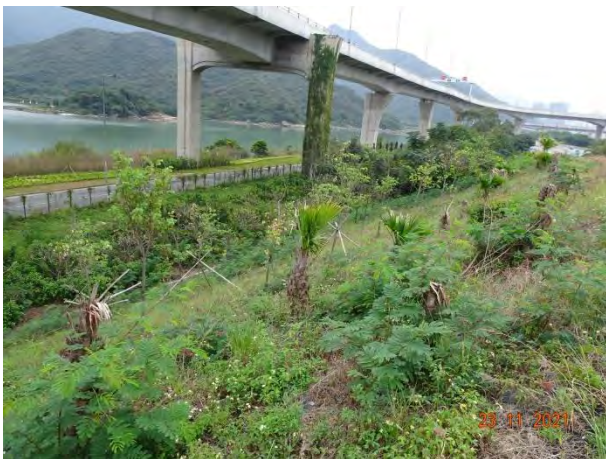
General View for Zone 3E
