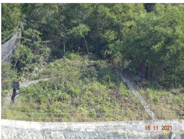
General View for Slope TP_D
