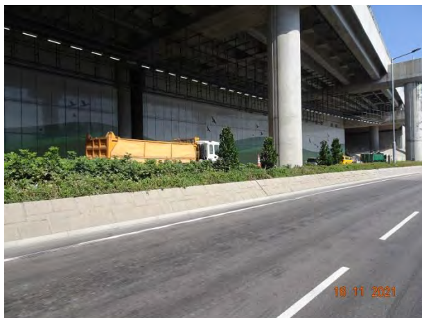
General View for Lung Mun Road
