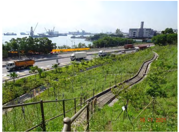
General View for Slope 5SE-D/C170
