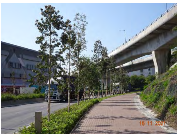
General View for Lung Mun Road
