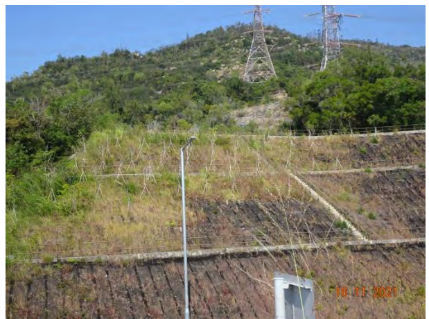
General View for Slope TP_B
