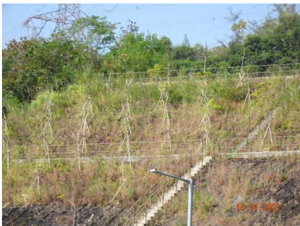
General View for Slope TP_B
