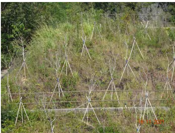
General View for Slope TP_B
