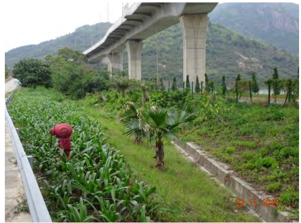
General View for Zone 3E
