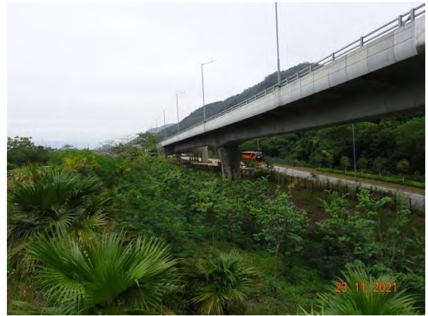
General View for Zone 3E
