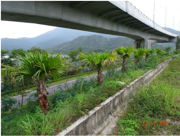
General View for Zone 3E
