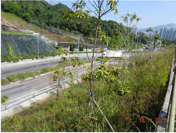
General View for Slope TP_C
