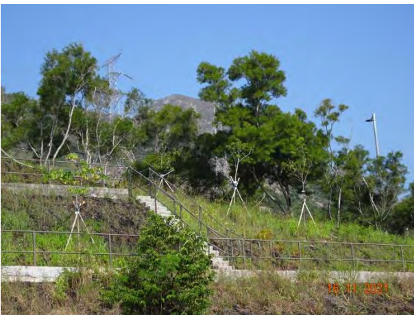
General View for Slope 5SE-D/C21
