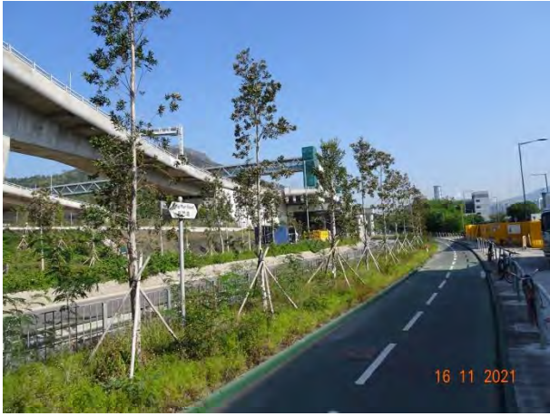
General View for Lung Mun Road
