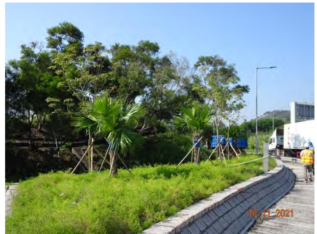
General View for Roundabout Area
