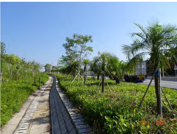
General View for Roundabout Area
