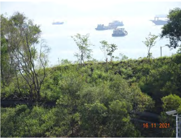
General View for Slope 5SE-D/C171
