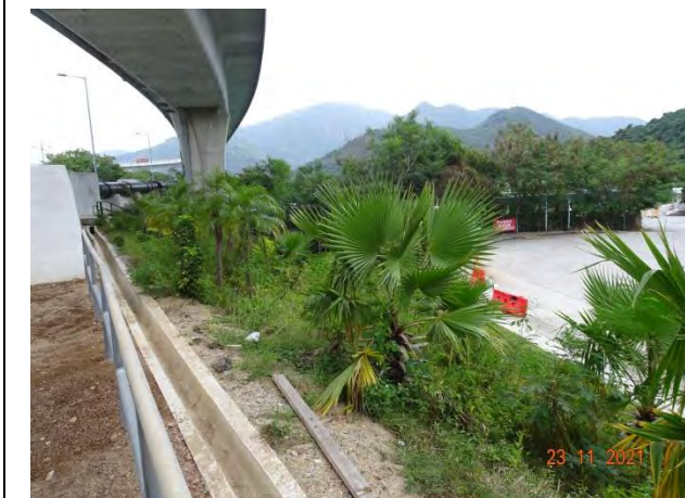
General View for Zone 1B
