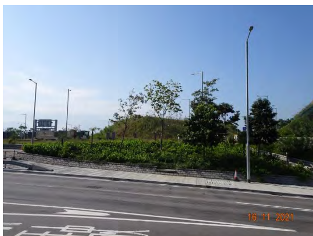
General View for planter near the Tunnel
