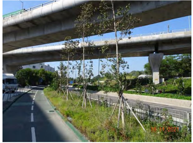
General View for Lung Mun Road
