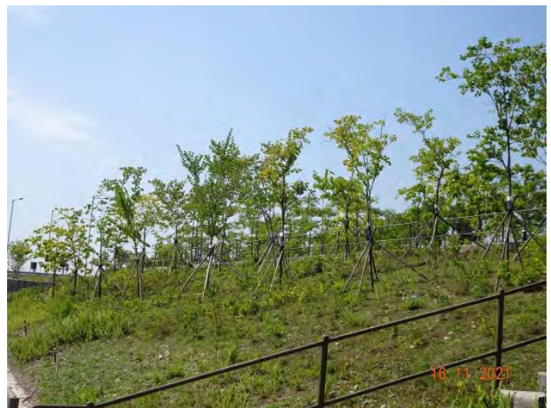
General View for Slope 5SE-D/C215
