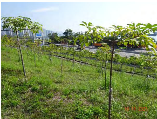
General View for Slope 5SE-D/C170
