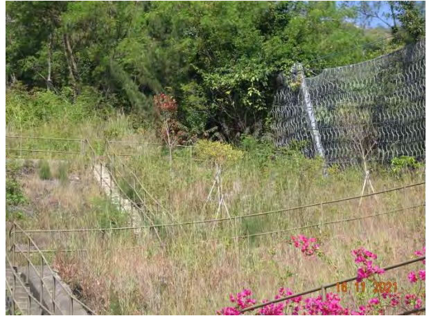
General View for Slope TP_A
