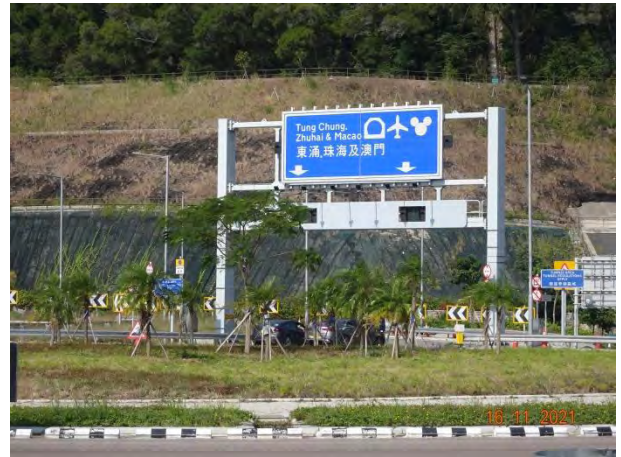
General View for Roundabout Area
