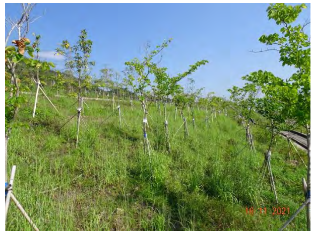
General View for Slope 5SE-D/C170
