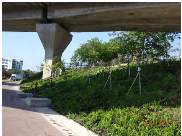
General View for Slope 5SE-D/C16
