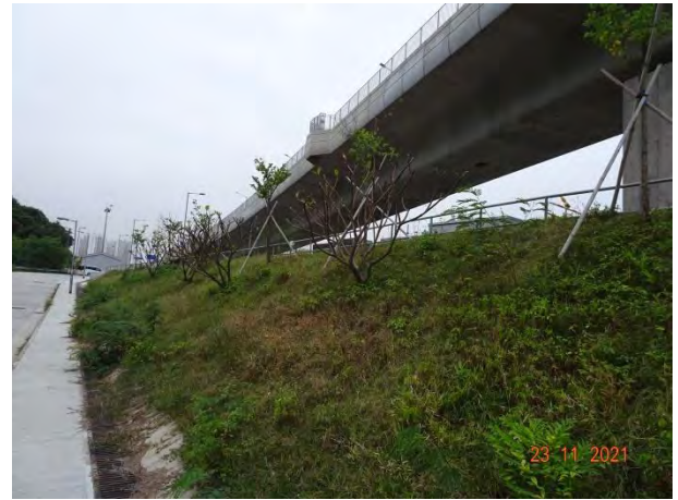
General View for Zone 1B
