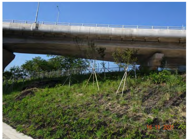
General View for Slope 5SE-D/C16
