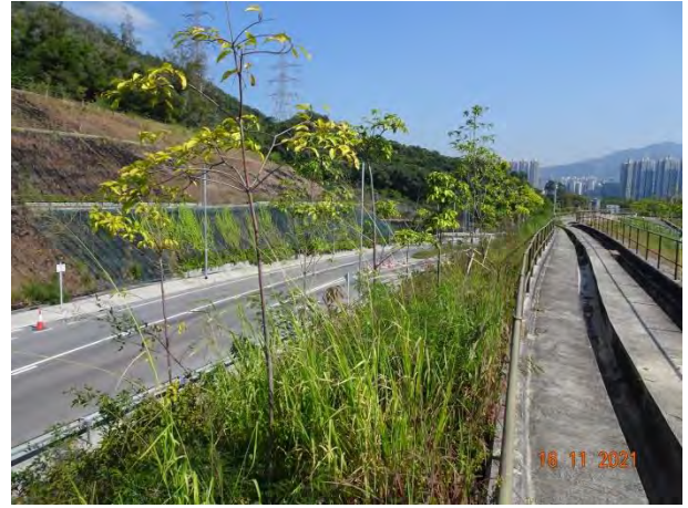
General View for Slope TP_C
