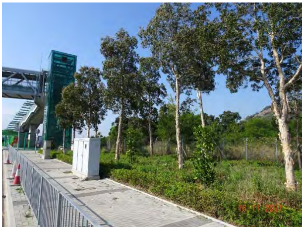
General View for Toll Plaza Interchange
