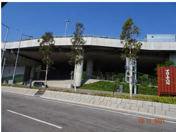
General View for Lung Mun Road
