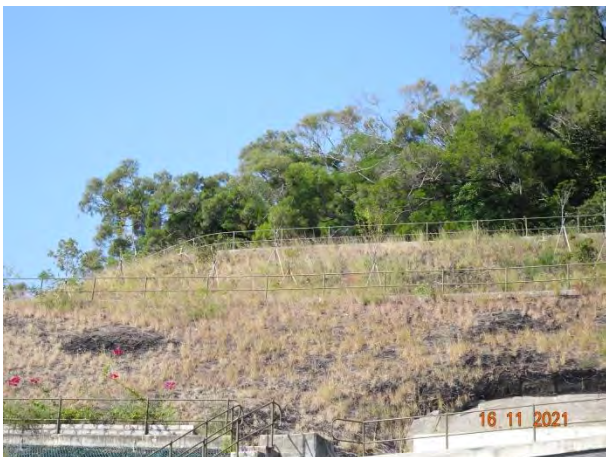
General View for Slope TP_A
