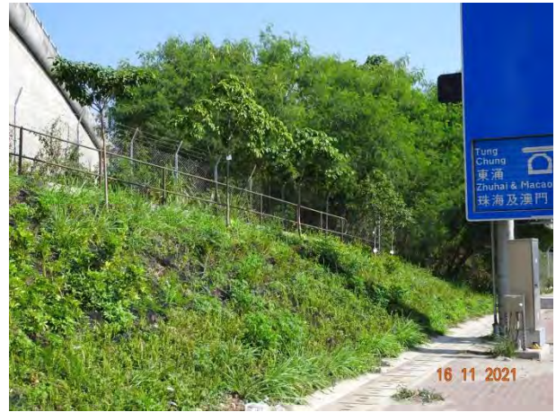
General View for Slope 5SE-D/C18
