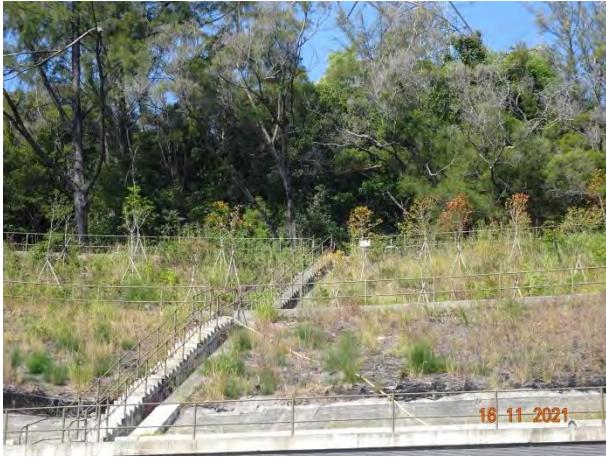
General View for Slope TP_A
