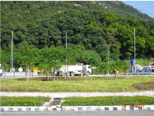
General View for Roundabout Area
