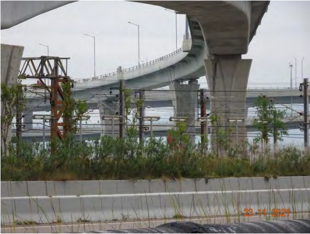
General View for Zone 3B
