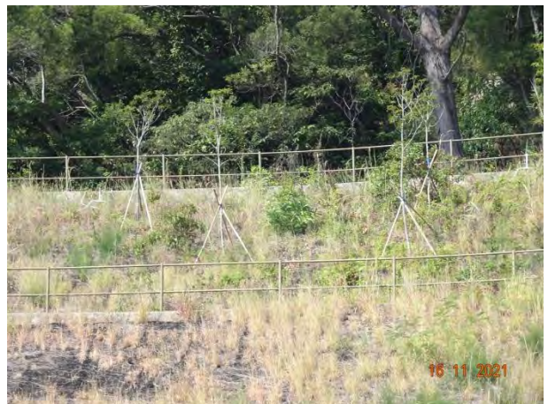
General View for Slope TP_A
