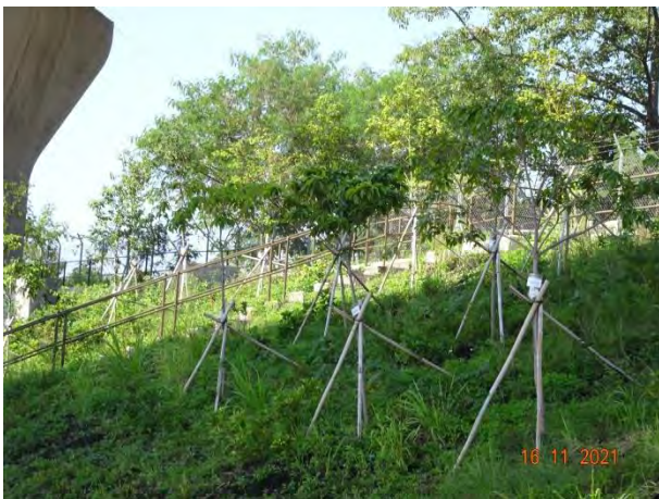
General View for Slope 5SE-D/C16
