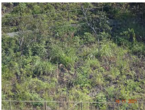
General View for Slope TP_D
