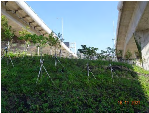
General View for Slope 5SE-D/C16
