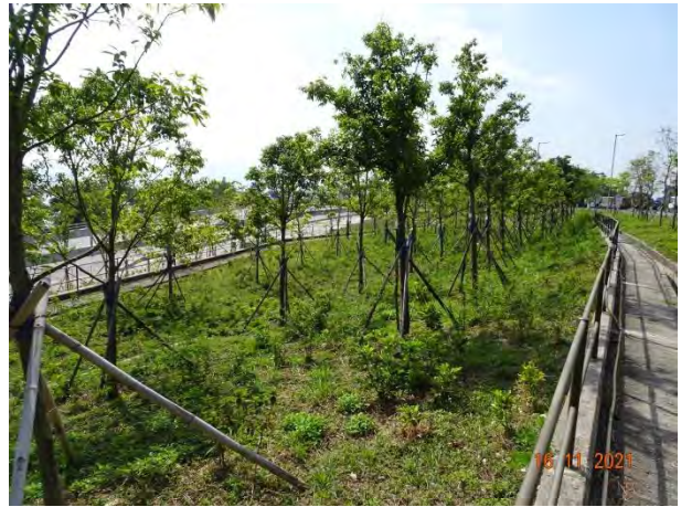
General View for Slope 5SE-D/C215
