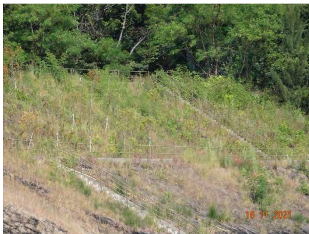
General View for Slope TP_B
