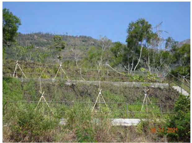
General View for Slope 5SE-D/C21
