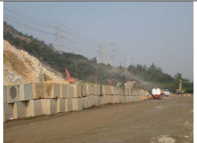
Photo 4 Water spraying and damp haul road was observed on 19 November 2014.
