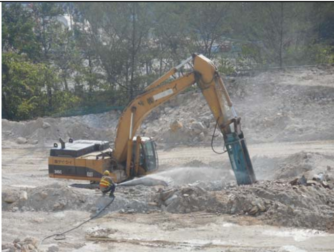
Photo 3 Water spraying during rock breaking work
