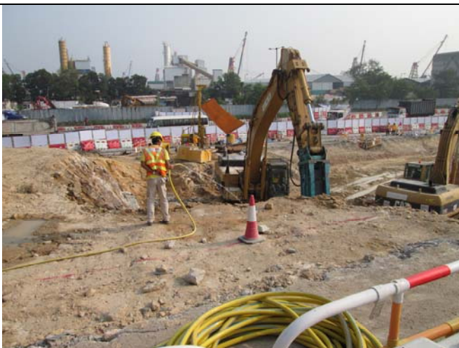
Photo 5 Water spraying during rock breaking work was observed on 19 November 2014.
