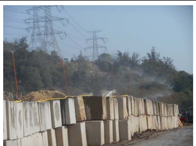
Photo 2 Installation of auto-water sprinkler in dusty area
