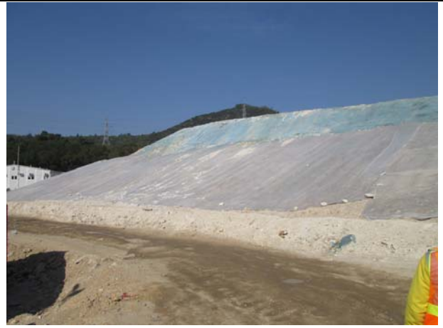
Photo 7 Covering of the exposed slopes by geotextile net was observed on 17 December 2014.
