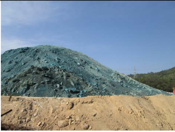
Photo 6 Hydro-seeding applied for the exposed slope was observed on 17 December 2014.
