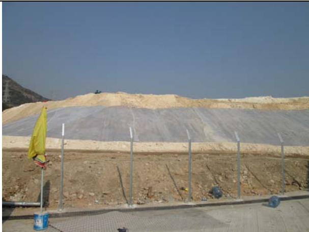
Photo 7 Covered part of the exposed slopes by geotextile net was observed on 12 December 2014.
