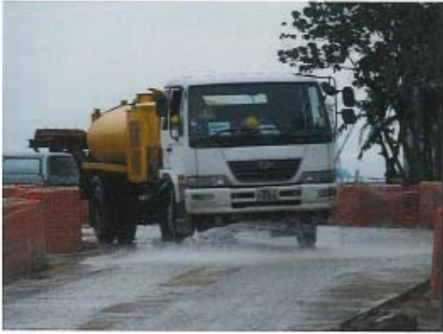
Photo 1 to 4 - Watering of haul road by water truck to keep road surface wet
