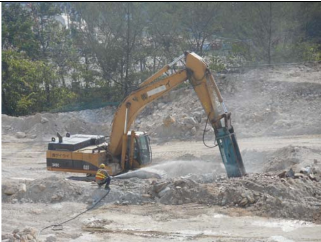
Photo 3 Water spraying during rock breaking work
