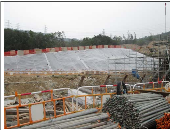
Photo 4 Covering of the exposed slopes by geotextile net was observed on 2 December 2014.
