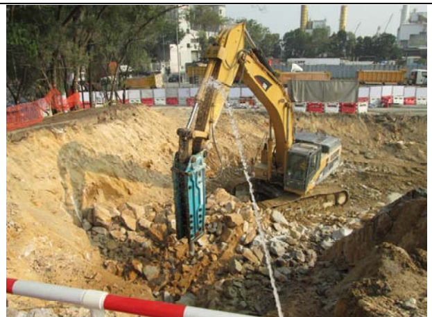
Photo 6 Water spraying during rock breaking work was observed on 12 December 2014.
