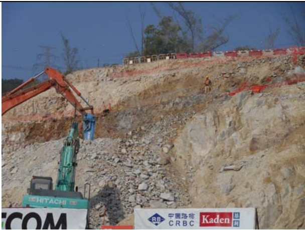
Photo 8 Water spraying during rock breaking work was observed on 17 December 2014.
