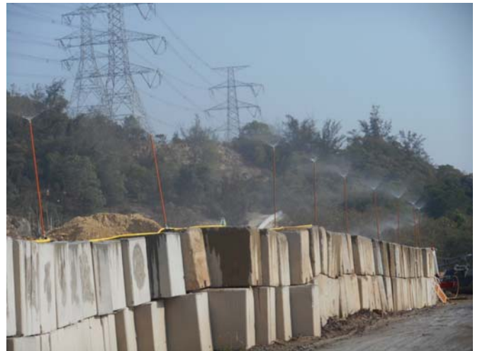
Photo 2 Installation of auto-water sprinkler in dusty area
