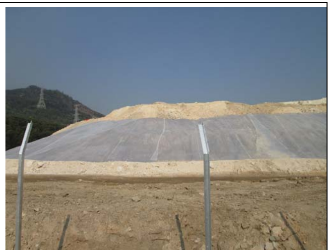
Photo 5 Covering of the exposed slopes by geotextile net was observed on 9 December 2014.
