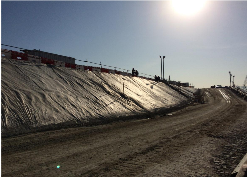
Hydro-seeding of area where works have been completed. (Reclamation Works Area)
