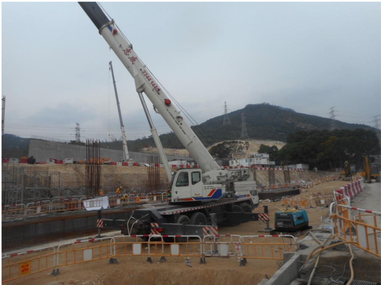
Location of the Retaining Wall B
