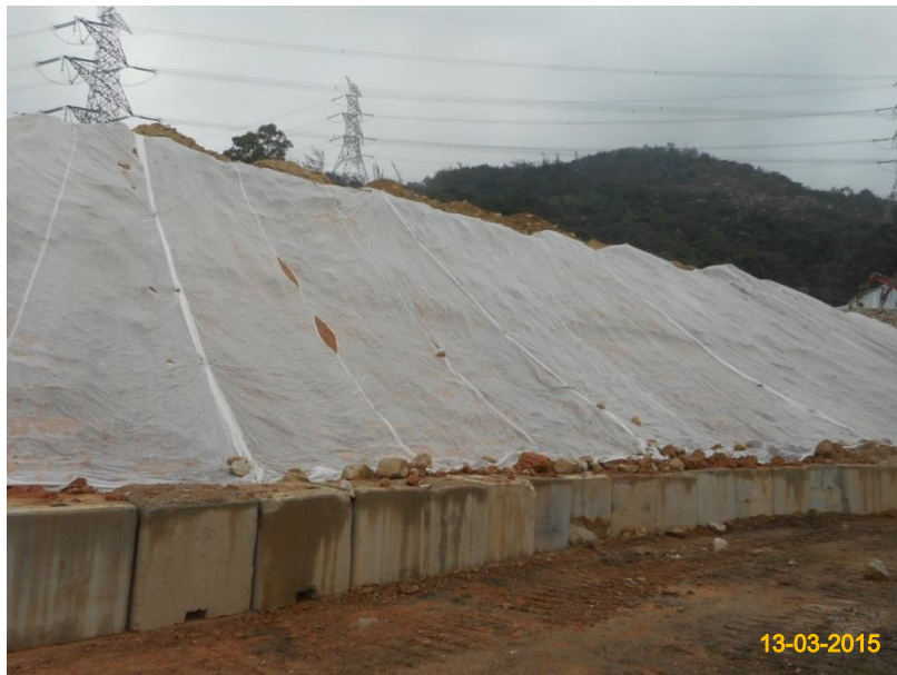
Item 4. Hydro-seeding or sheeting provided at stockpile.
