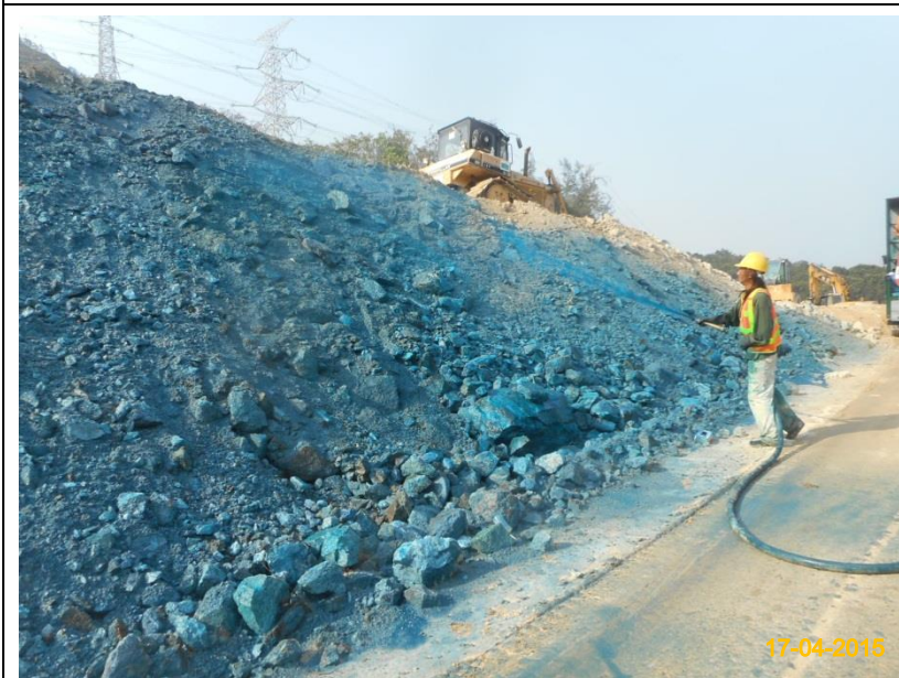
Item 4. Hydro-seeding or sheeting provided at stockpile.
