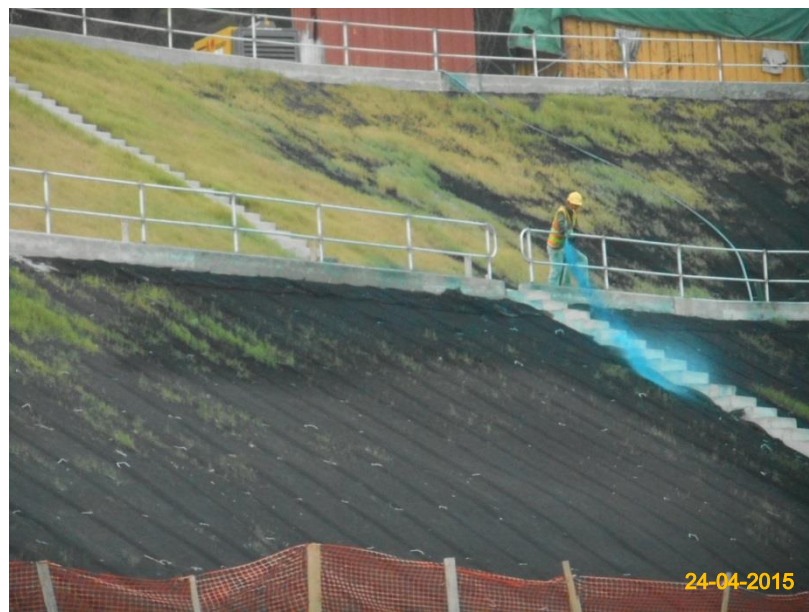
Item 4. Hydro-seeding or sheeting provided at stockpile.
