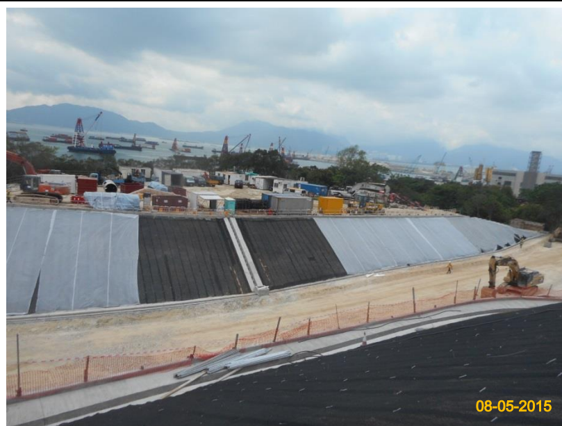
Item 4. Hydro-seeding or sheeting provided at stockpile.
