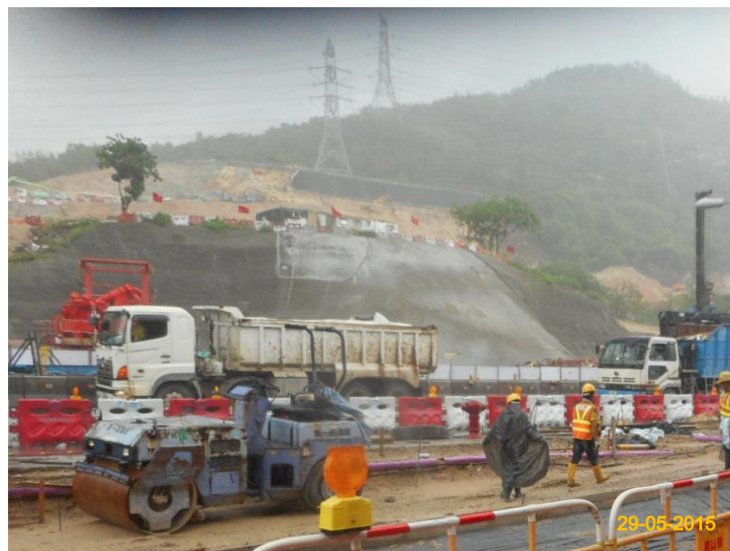
Item 4. Hydro-seeding or sheeting provided at stockpile.
