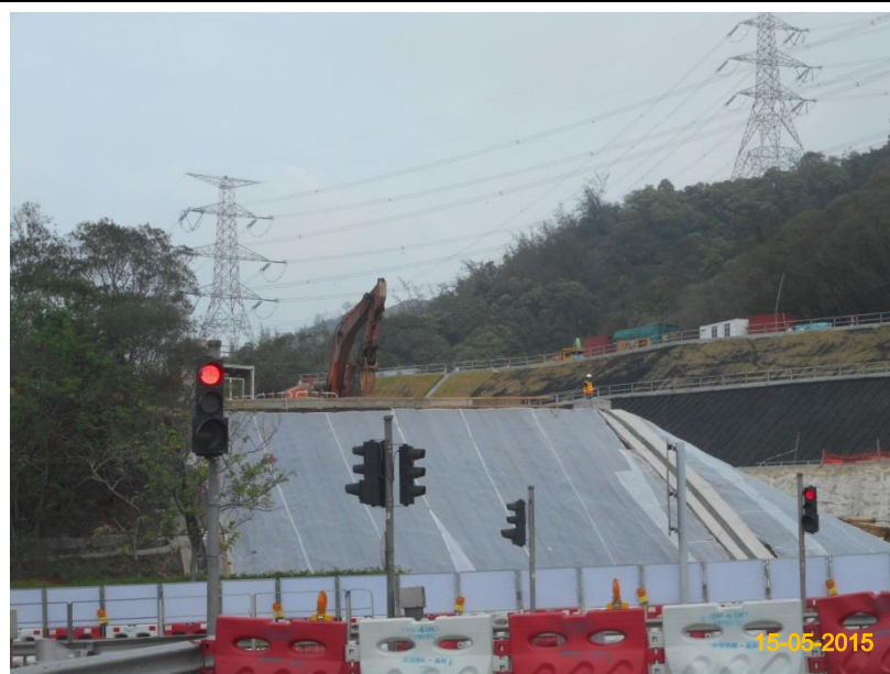
Item 4. Hydro-seeding or sheeting provided at stockpile.
