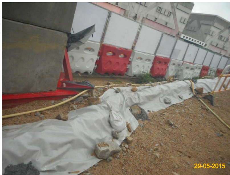
Item 7. Ensure no run-off into water body.
