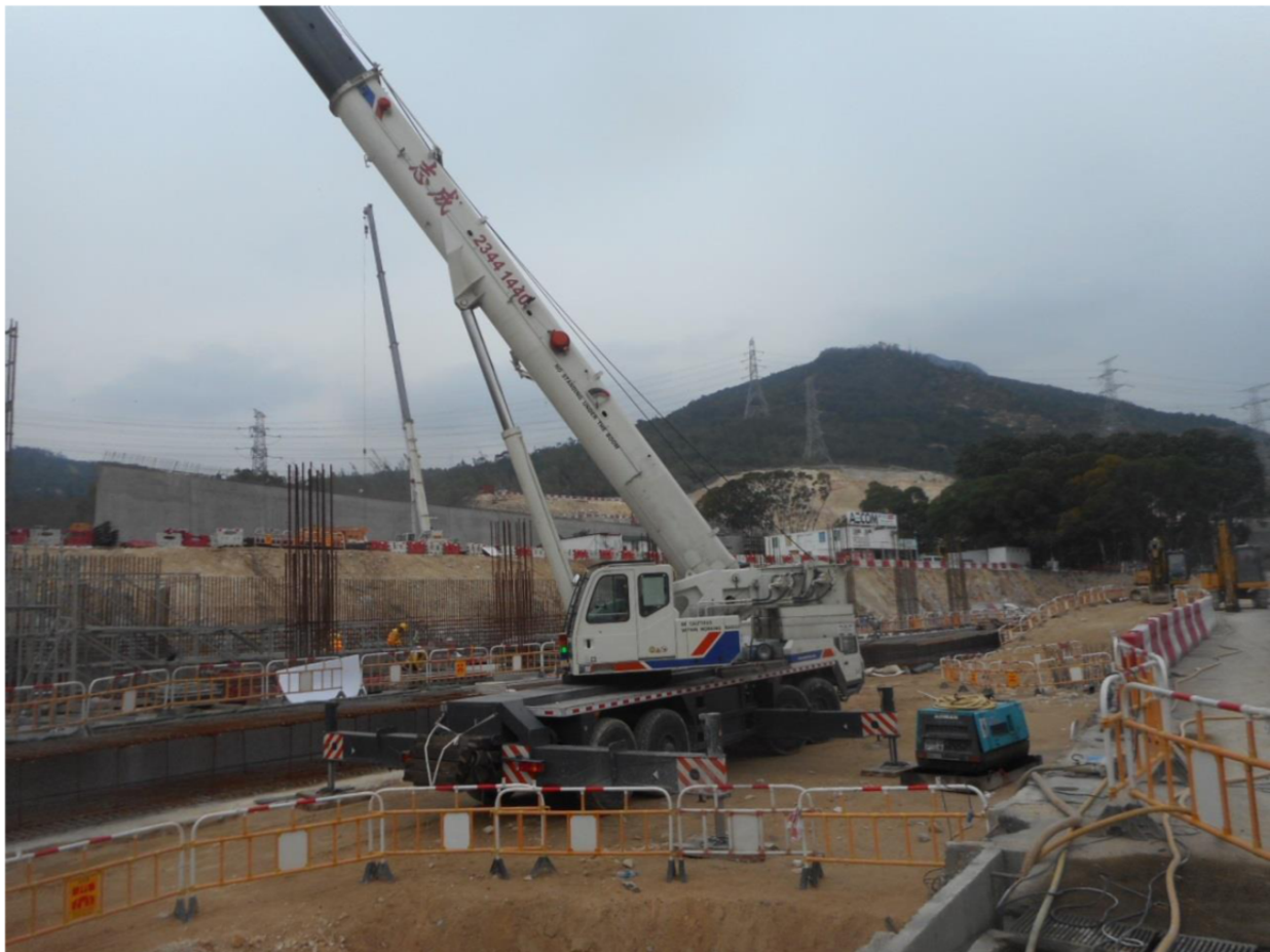
Location of the Retaining Wall B
