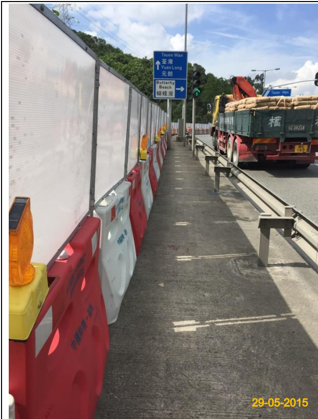
Item 5. Hoarding with panel around works area & Item 6. Temporary traffic management lighting.
