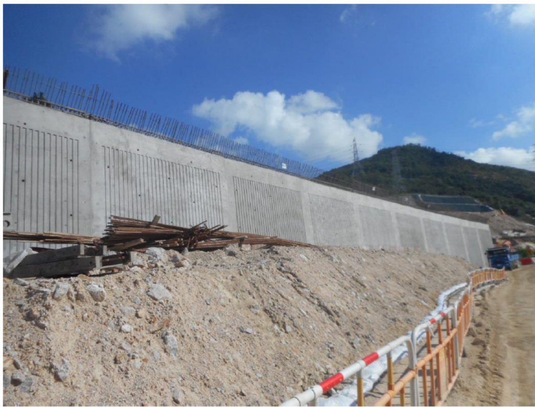
Location of the Retaining Wall F
