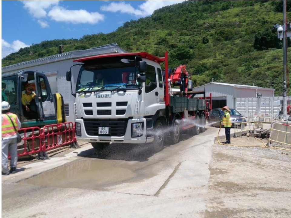
Truck wheel washing at Site Access 9B (without loading)
