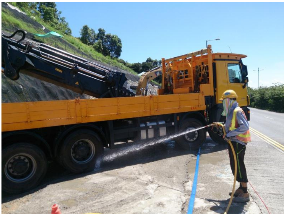
Truck wheel washing at Site Access 9B (without loading)
