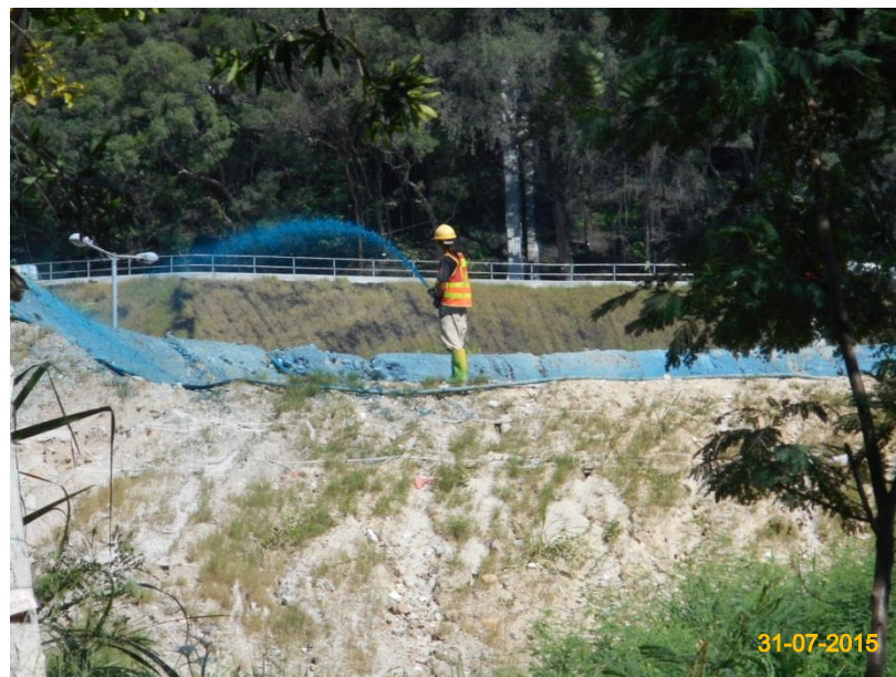
Item 4. Hydro-seeding or sheeting provided at stockpile.
