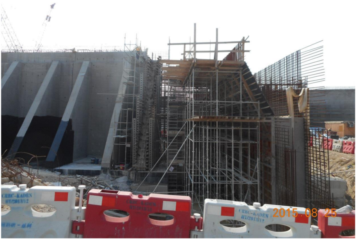
Location of the Retaining Wall F
