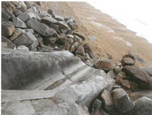
Photo 17a/17b: The portion of sand bed suspected trapped with mud near the outfall was washed off.
