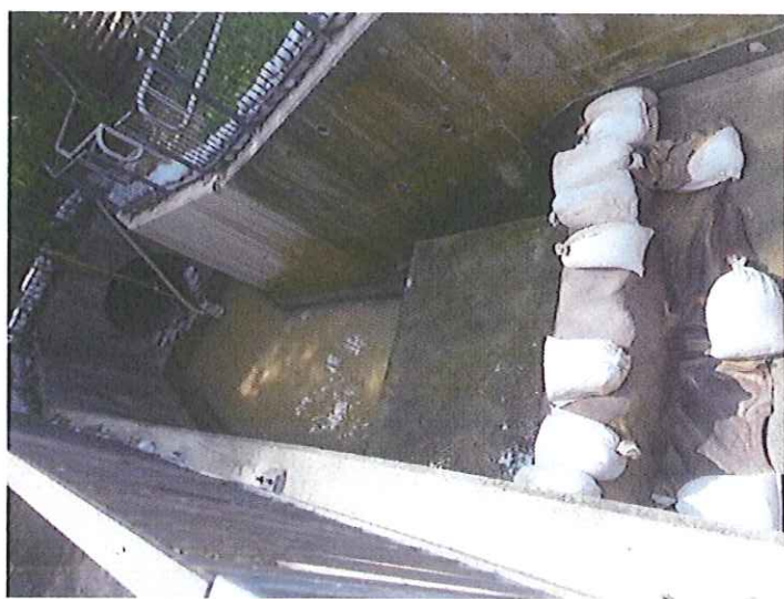
At East Portal, no water discharging.
