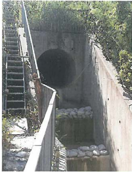
Photo 1: Sand bags were stacked at each step/level. Debris, grit and silt inside the cascade were removed.
