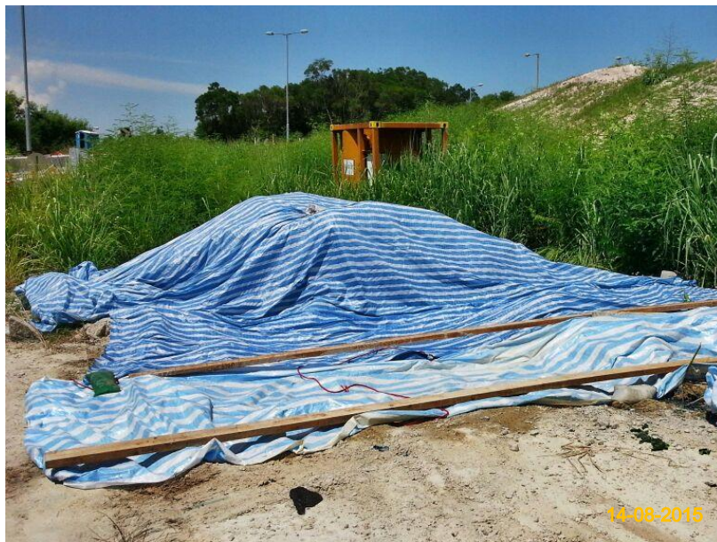
Item 4. Hydro-seeding or sheeting provided at stockpile.
