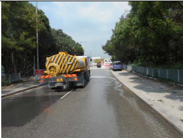
Photo 3 Water bowser was arranged for road cleaning on the Lung Mun Road and the associated roads
