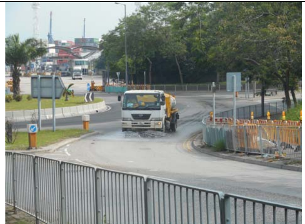
Photo 4 Water bowser was arranged for road cleaning on the Lung Mun Road and the associated roads
