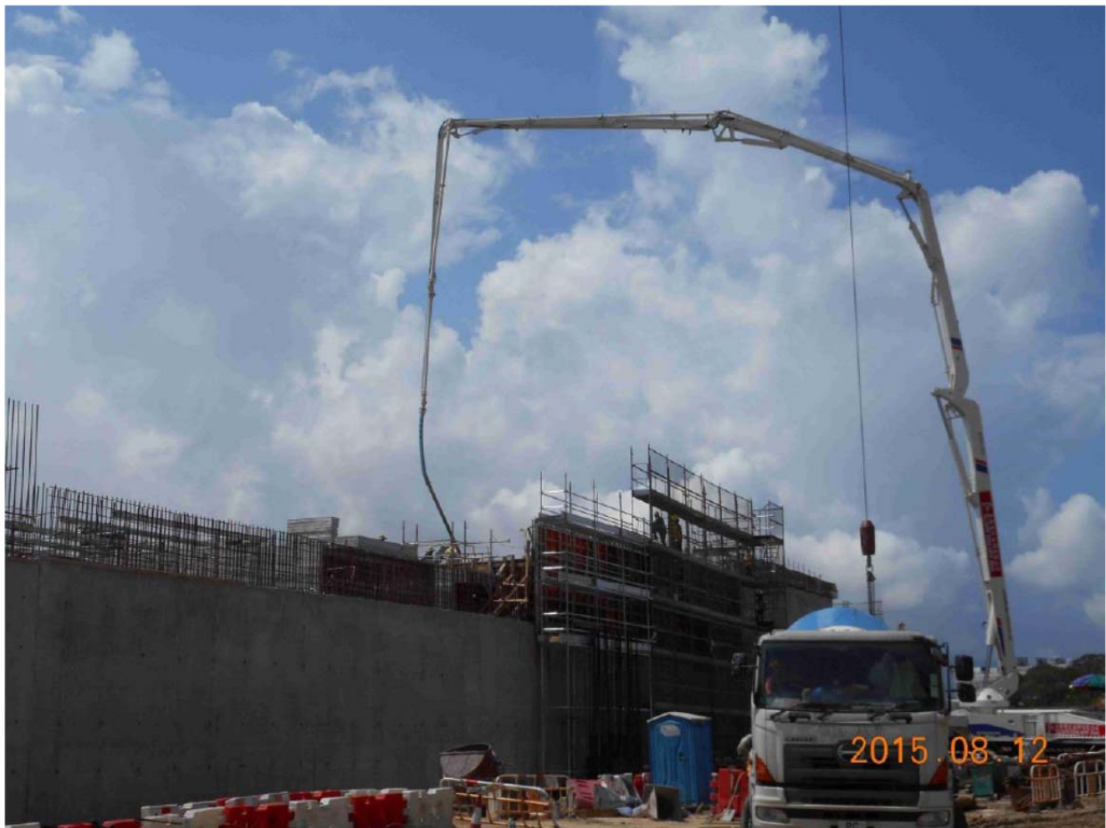
Location of the Retaining Wall B
