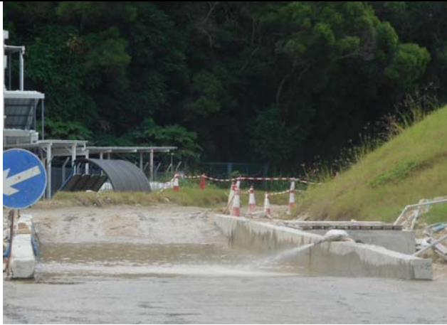
Photo 1 Wheel washing facilities was provide at site exit
