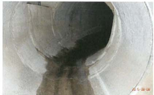
Photo 18a/18b: The 1800 dia. pipe cleaning works was completed.
