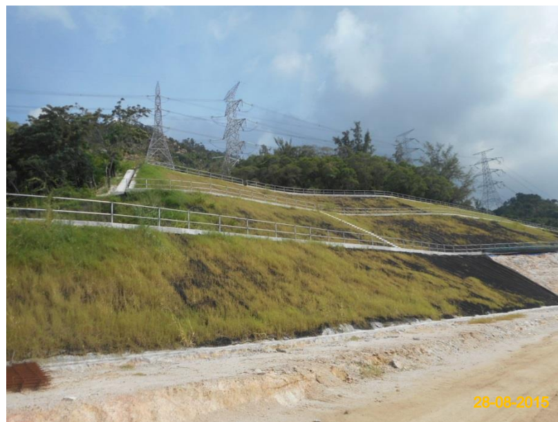
Item 4. Hydro-seeding or sheeting provided at stockpile.
