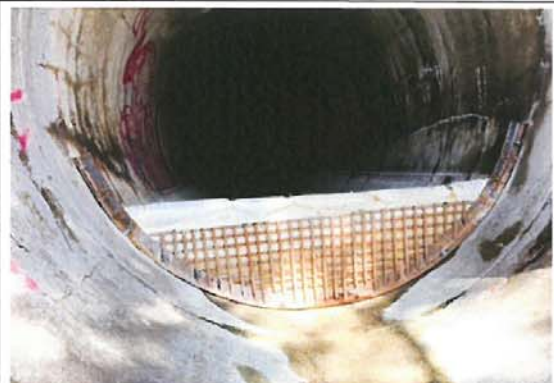
Photo 6: The concerned drainage pipe (near the pipe jacking works) was sealed up.
