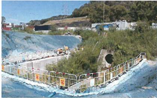
Photo 1: Sand bags were stacked at each step/level. Debris, grit and silt inside the cascade were removed.
