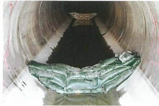
Photo 8a: Silt screen was installed. Photo 8b: Sand bags were deployed
