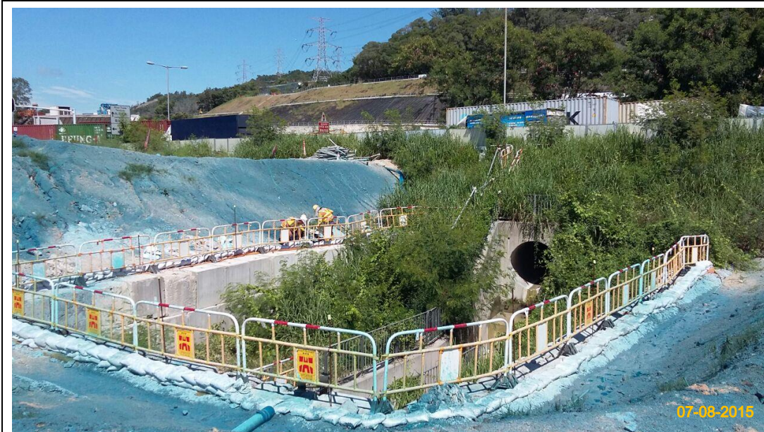
Item 4. Hydro-seeding or sheeting provided at stockpile.
