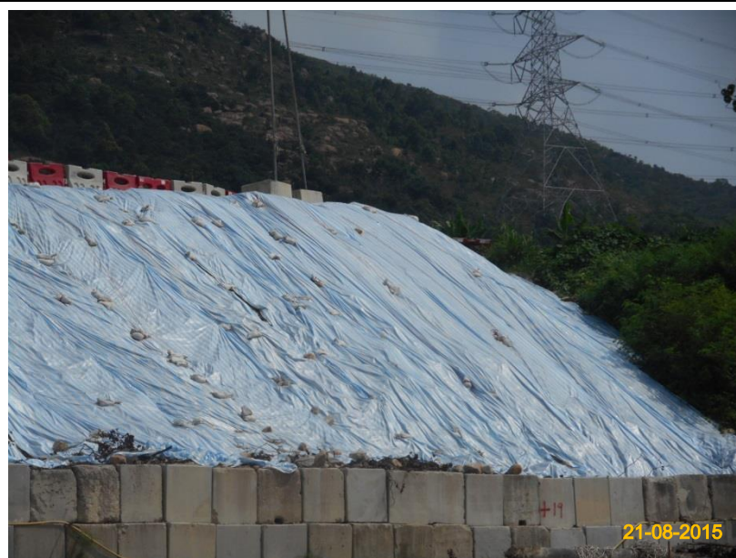
Item 4. Hydro-seeding or sheeting provided at stockpile.
