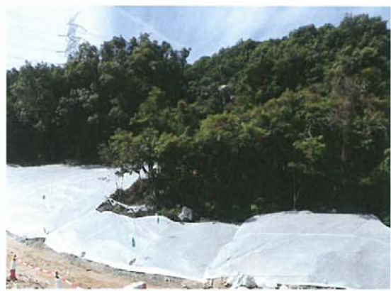
Photo 12: The exposed slope above the cascade was covered.
