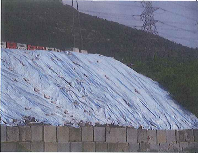
Tarpaulin was provided at exposed slope.
