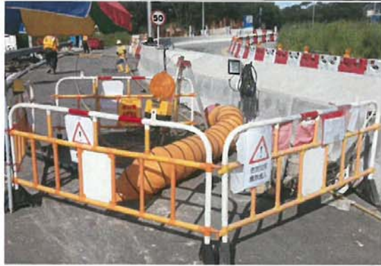
Photo 5: The area near the desilting tank was tidied up and a cement bund was formed to contain the dripping water.
