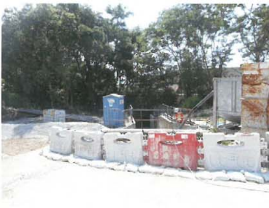
Photo 11: The haul road above the cascade was paved with concrete.
