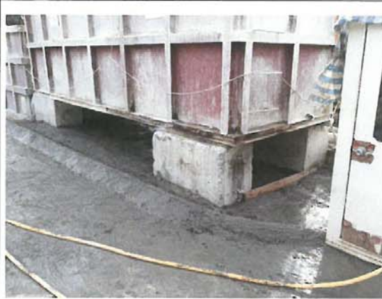
Photo 5: The area near the desilting tank was tidied up and a cement bund was formed to contain the dripping water.
