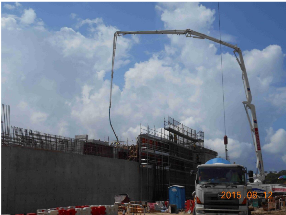
Location of the Retaining Wall B
