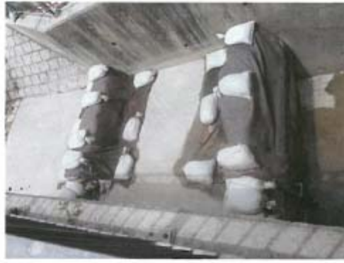
Photo 6: Maintain geo-textiles on top of sandbags in the cascade.
