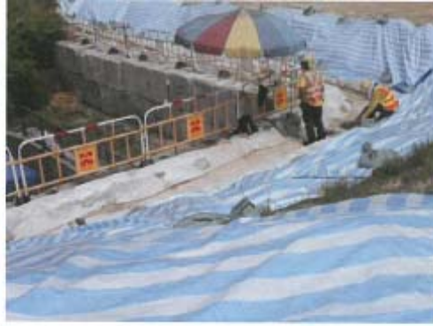
Photo 12: Cover exposed slopes.
