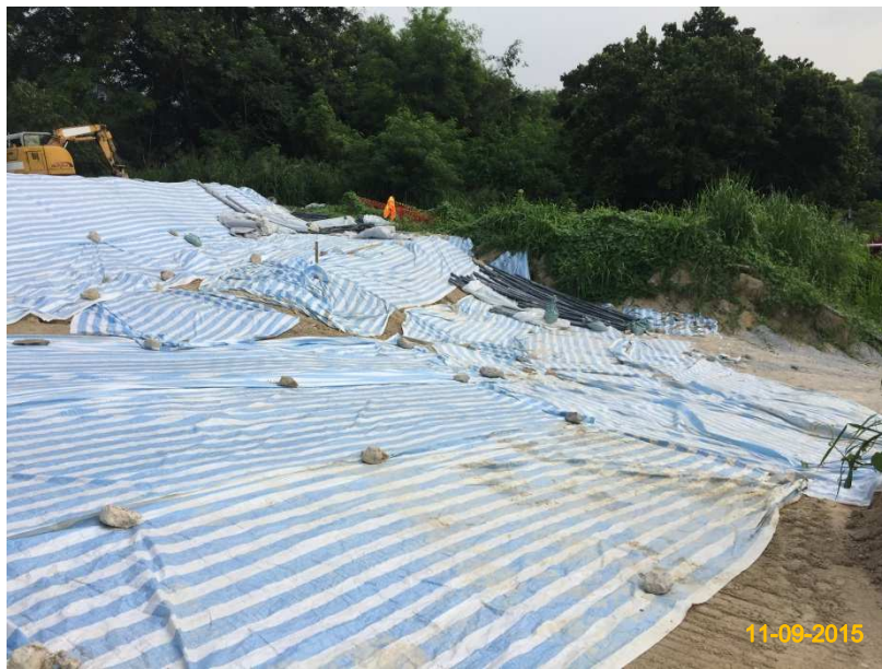
Item 4. Hydro-seeding or sheeting provided at stockpile.
