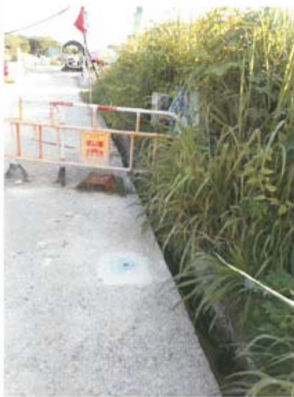
Photo 7: U-channel at +35mPD platform blocked.
