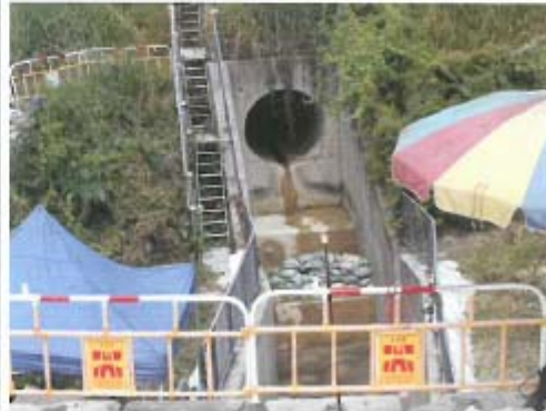
Photo 8: Clean up the associated u-channels
