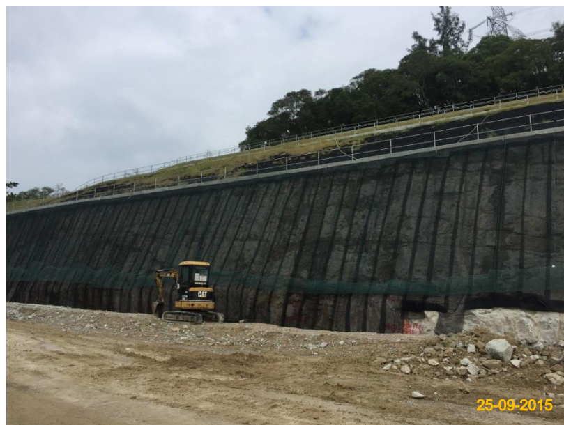
Item 4. Hydro-seeding or sheeting provided at stockpile.
