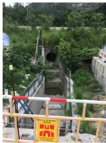
MH5: Cascade condition
