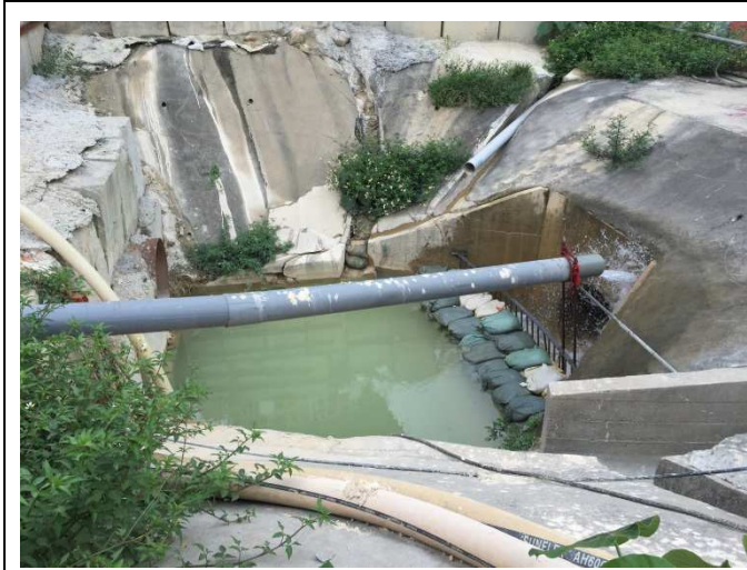
Stream A: Outfall pit was in normal condition.
