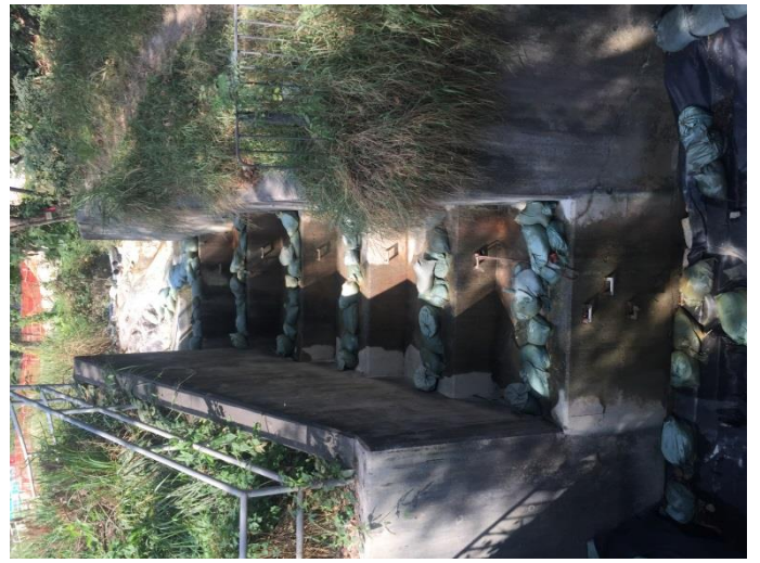
Stream B Outfall: Cascade step channel condition
