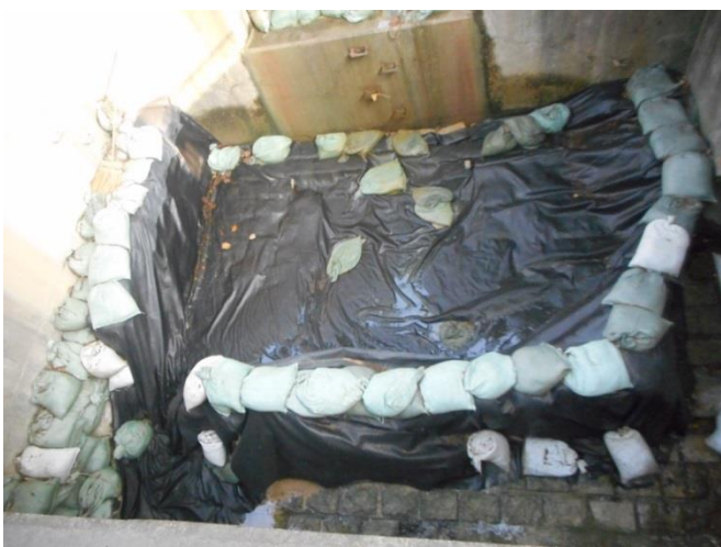
Stream B Outfall: Cascade was in normal condition.
