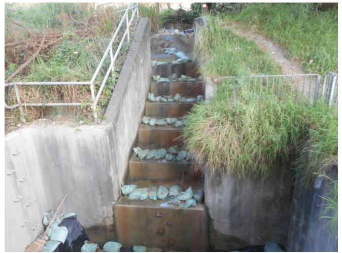
Stream B Outfall: Cascade step channel condition
