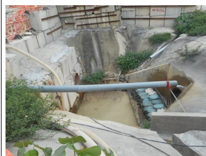
Stream A Outfall: pumped muddy water and discharged after treatment.
