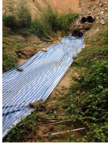
Stream B: Tarpaulin was used to avoid treated water disturbing.
