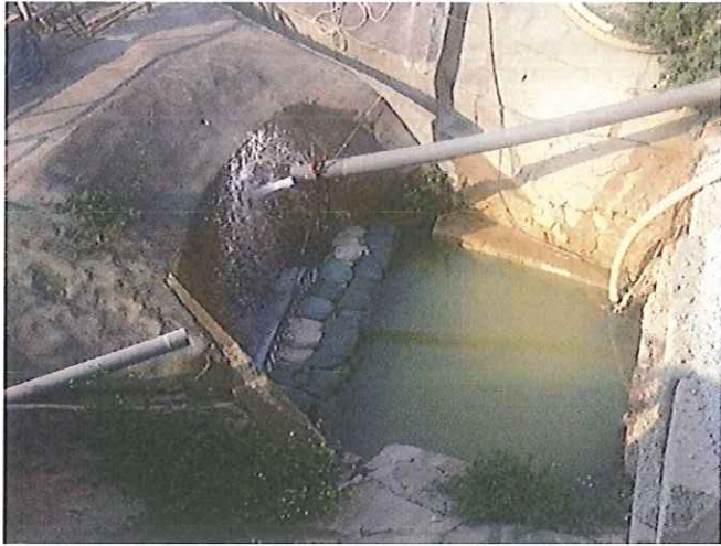
Stream A Outfall: in normal condition.
