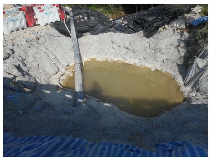
Stream B Pit 1: in normal condition.
