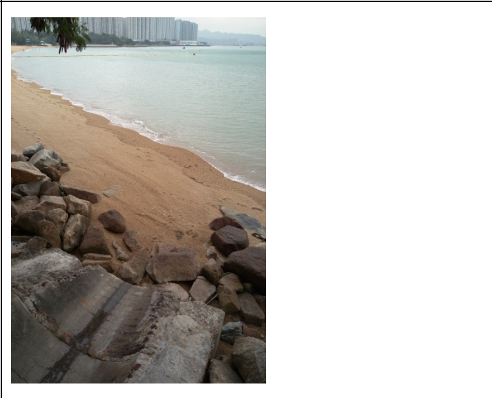
Outfall 1: No muddy water leaking out
