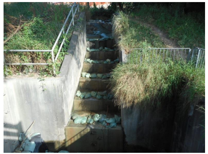
Stream B Outfall: Cascade step channel condition
