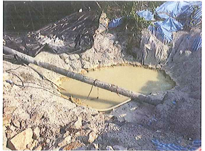
Stream B Pit 1: in normal condition.
