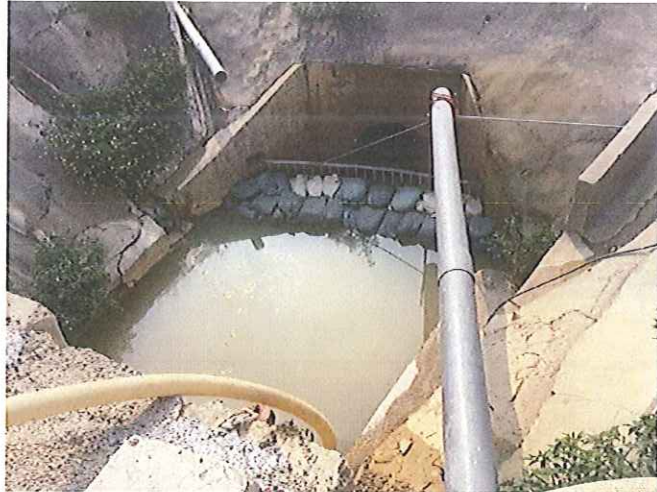
Stream A Outfall: in normal condition.
