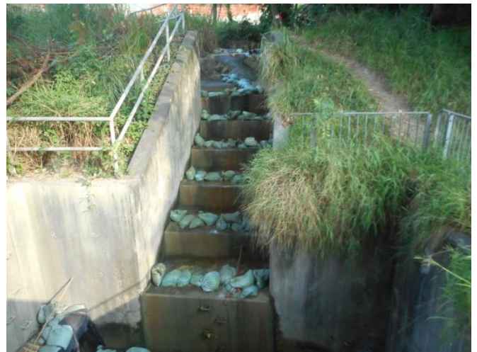
Stream B Outfall: Cascade step channel condition
