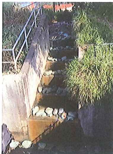
Stream B Outfall: Cascade step channel condition
