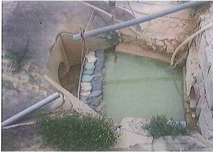
Stream A: Outfall pit was in normal condition.
