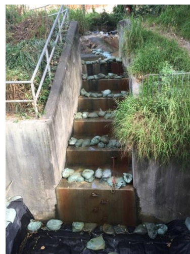
Stream B Outfall: Cascade step channel condition
