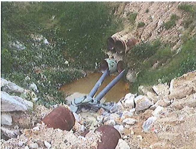
Stream B: Treated water was directly discharged to downstream bypass the Pit 2.
