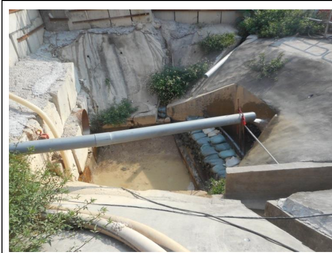
Stream A Outfall: pumped muddy water and discharged after treatment.
