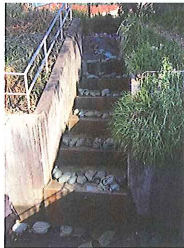
Stream B Outfall: Cascade step channel condition
