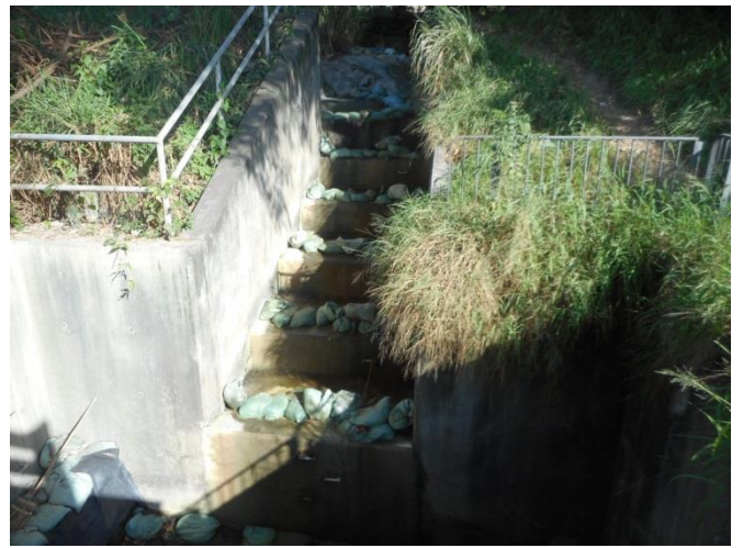
Stream B Outfall: Cascade step channel condition
