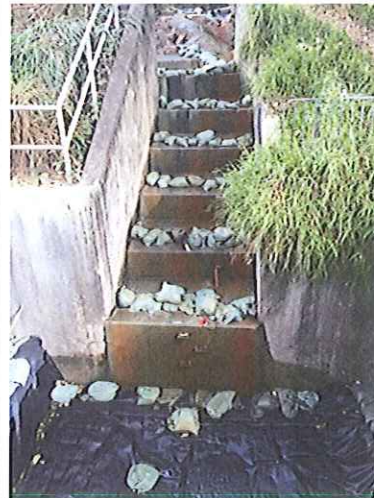
Stream B Outfall: Cascade step channel condition
