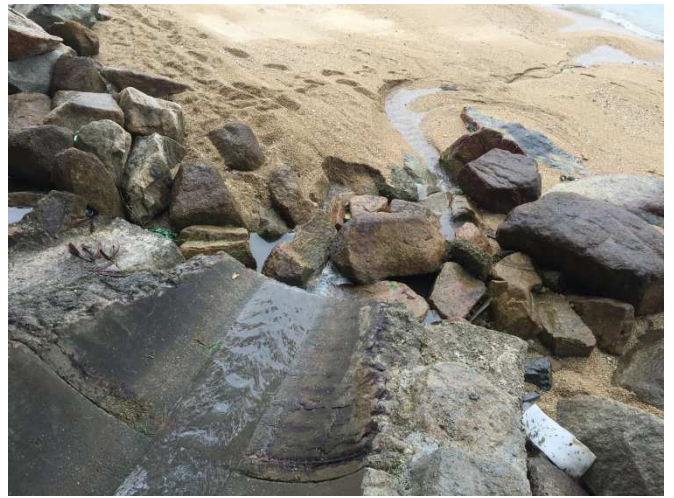
Outfall 1: Clean water is discharging.
