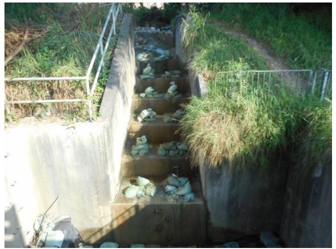
Stream B Outfall: Cascade step channel condition
