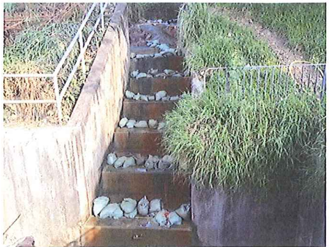
Stream B Outfall: Cascade step channel condition
