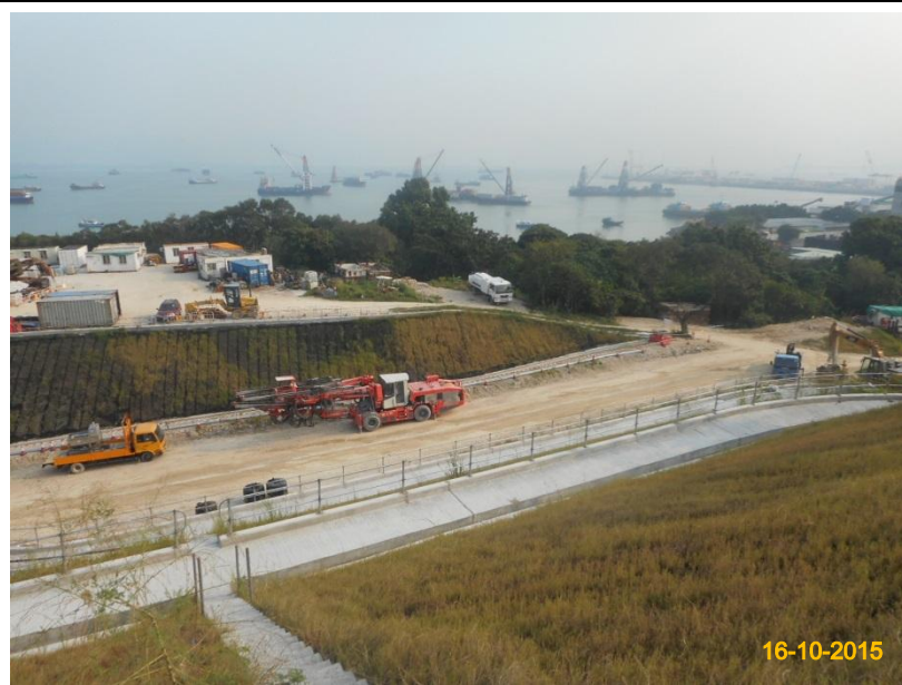
Item 4. Hydro-seeding or sheeting provided at stockpile.
