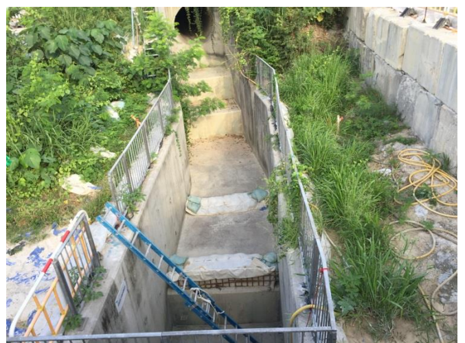
MH5 Cascade: No water is discharging.
