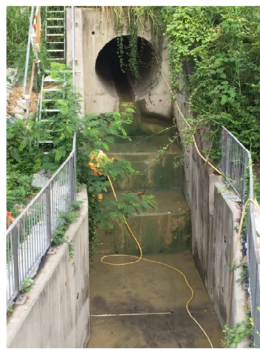
MH5: Cascade condition
