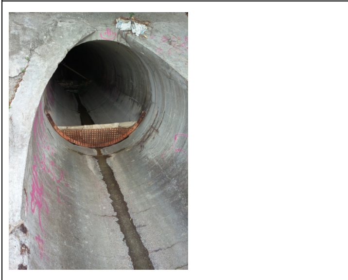
Outfall 1: No muddy water leaking out
