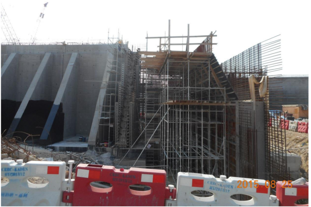
Location of the Retaining Wall F
