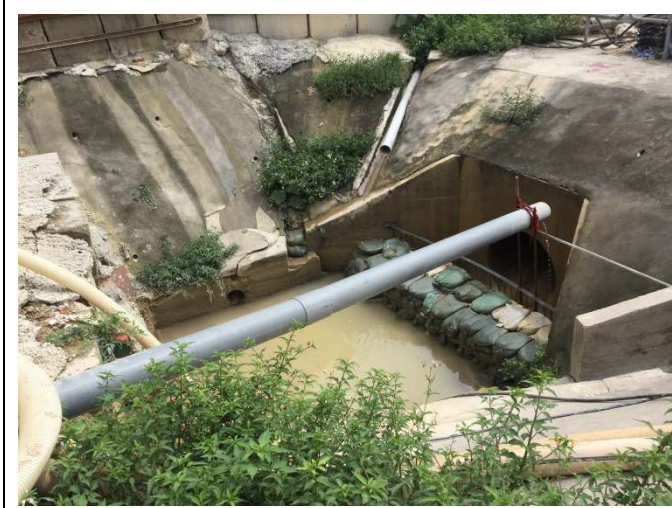
Stream A: Outfall pit in normal condition.
