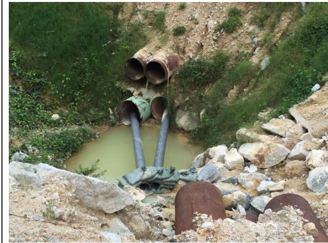
Stream B: Treated water was directly discharged to downstream bypass the Pit 2.
