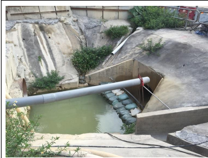
Stream A Outfall: in normal condition.
