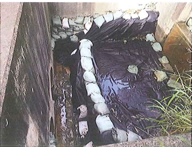
Stream B Outfall: Cascade was in normal condition.
