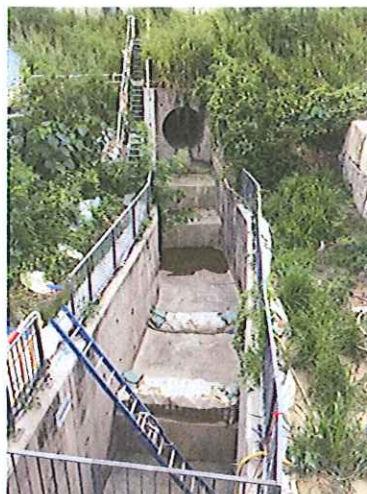
MH5: Cascade condition
