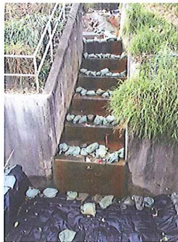
Stream B: Cascade step channel condition
