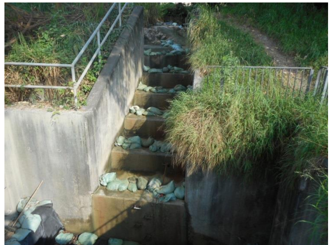
Stream B Outfall: Cascade step channel condition
