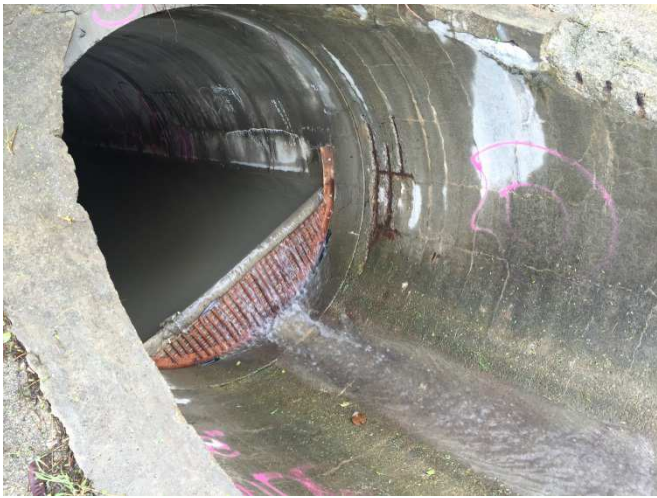
Outfall 1: Outfall condition is OK.
