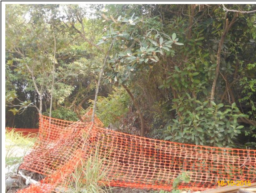
Item 1. Existing trees on boundary of the Project Area have been protected carefully during construction.
