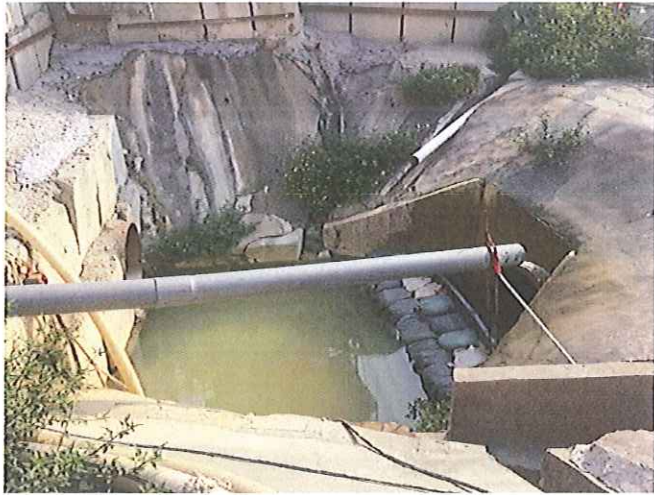
Stream A Outfall: in normal condition.
