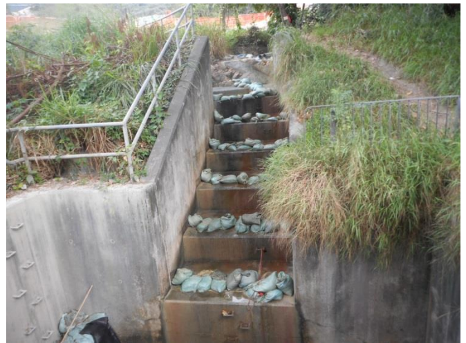
Stream B Outfall: Cascade step channel condition
