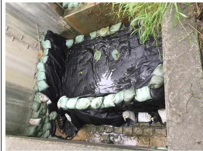
Stream B: Cascade was in normal condition.
