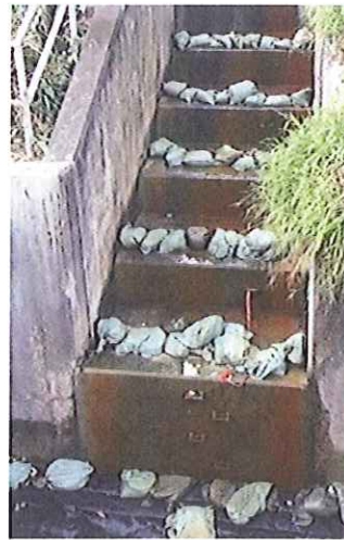
Stream B Outfall: Cascade step channel condition
