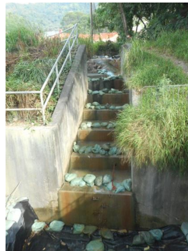
Stream B Outfall: Cascade step channel condition
