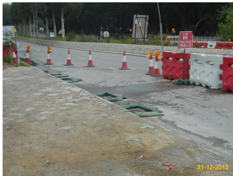
Item 7. Ensure no run-off into water body.
