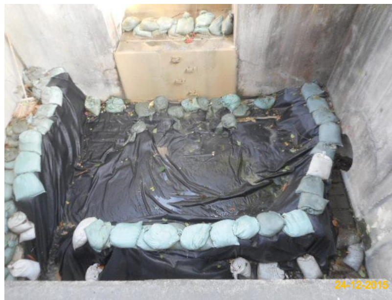
Item 7. Ensure no run-off into water body.
