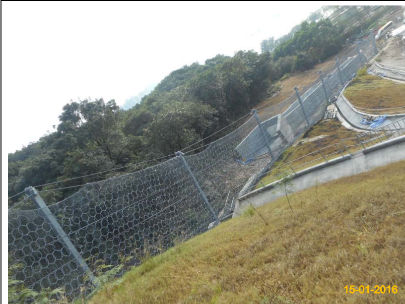
Item 4. Hydro-seeding or sheeting provided at stockpile.
