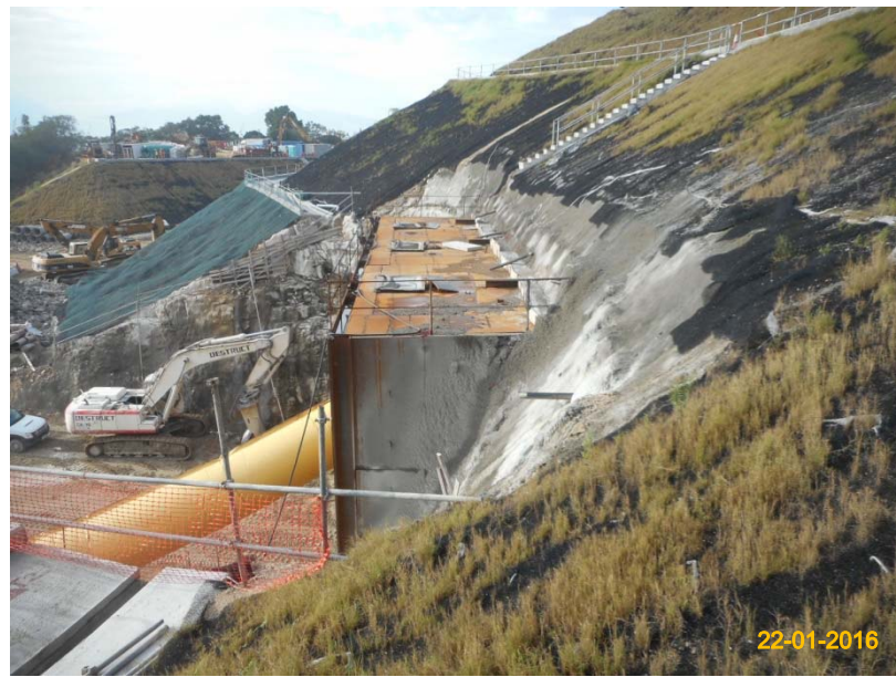
Item 4. Hydro-seeding or sheeting provided at stockpile.
