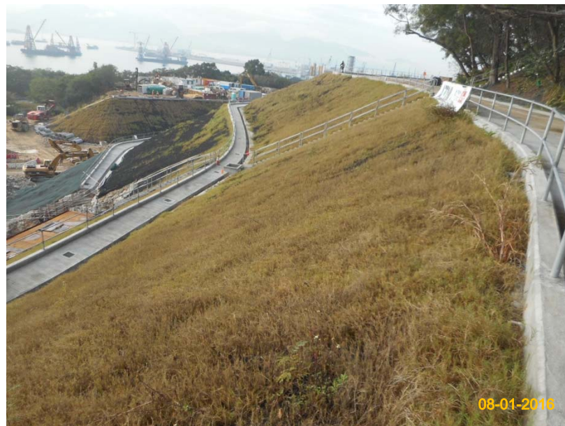
Item 4. Hydro-seeding or sheeting provided at stockpile.
