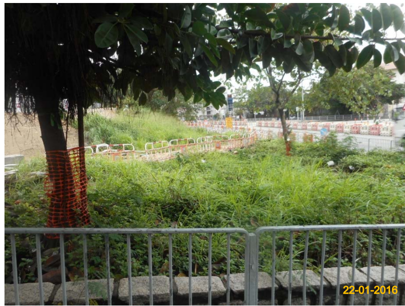
Item 1. Existing trees on boundary of the Project Area have been protected carefully during construction.
