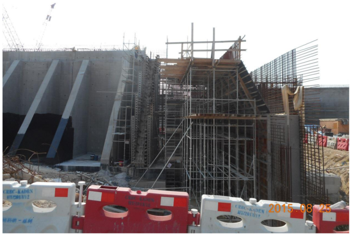
Location of the Retaining Wall F
