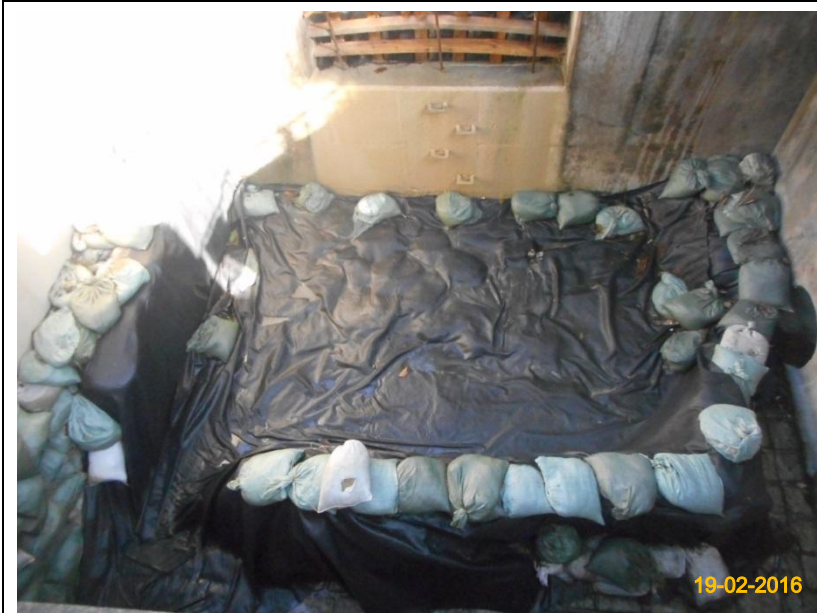
Item 7. Ensure no run-off into water body.
