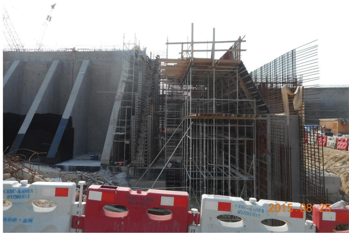
Location of the Retaining Wall F
