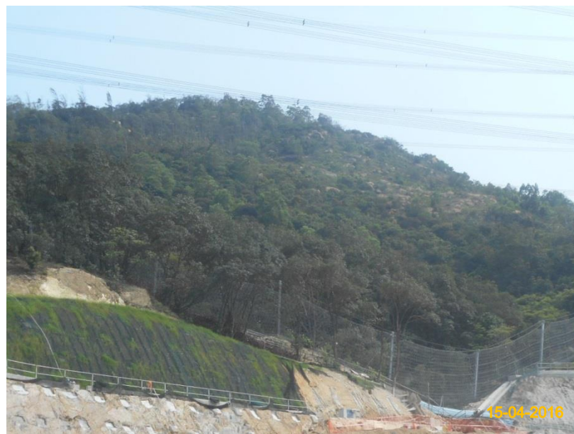
Item 4. Hydro-seeding or sheeting provided at stockpile.
