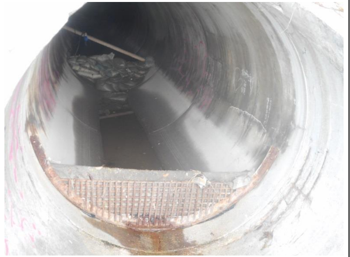
Outfall 1: No water is discharging.
