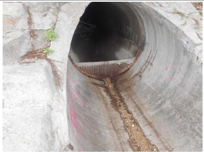
Outfall 1: No water is discharging.
