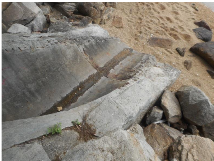
Outfall 1: No water is discharging.
