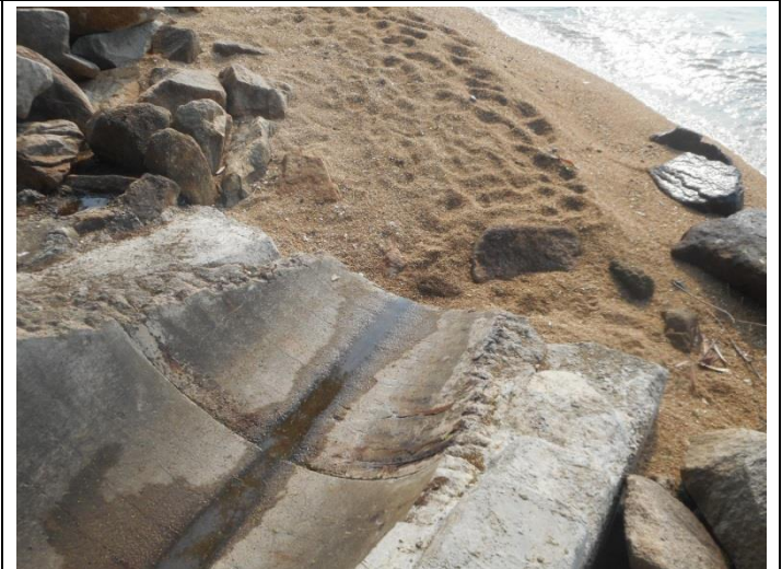
Outfall 1: No water is discharging.
