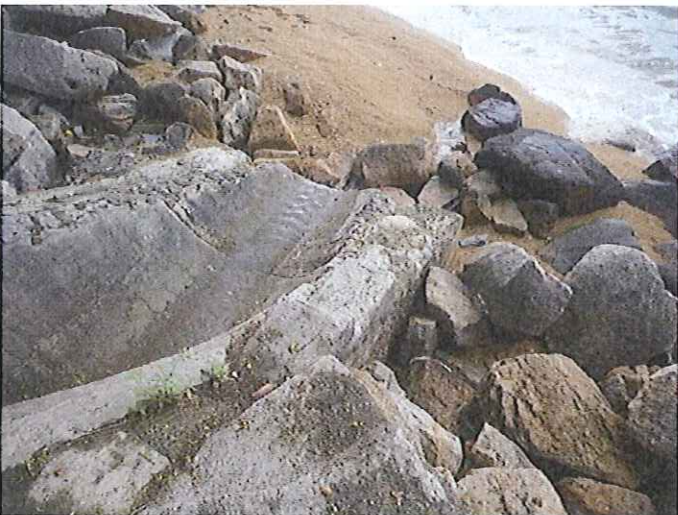
Outfall 1: No water is discharging.
