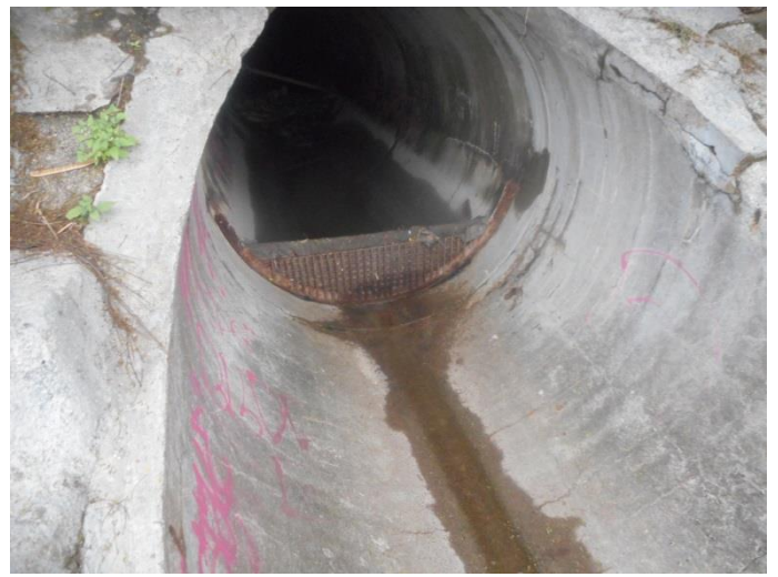
Outfall 1: No water is discharging.
