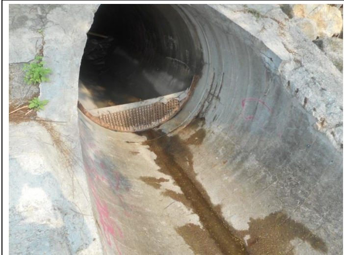
Outfall 1: No water is discharging.
