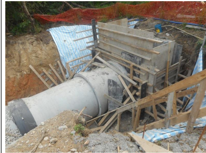
East Portal: No water is discharged.
