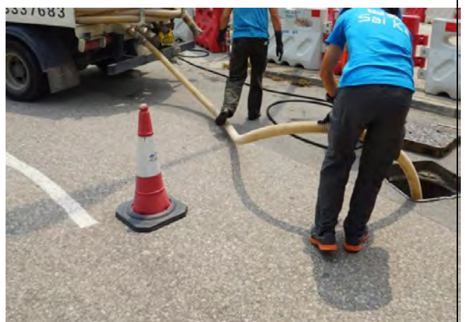
Photo 6 Drainage cleansing works for Ho Fuk Street.
