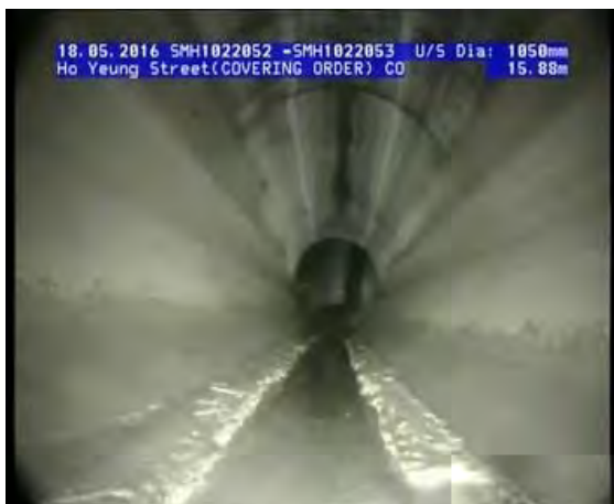
Photo 5 CCTV drainage survey at Ho Yeung Street.
