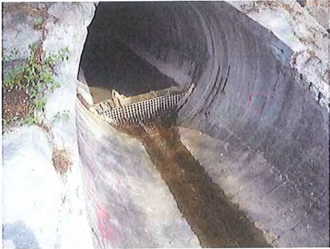
Outfall 1: Clean water is discharging.
