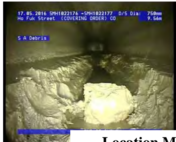
Photo 4 CCTV drainage survey at Ho Fuk Street.
