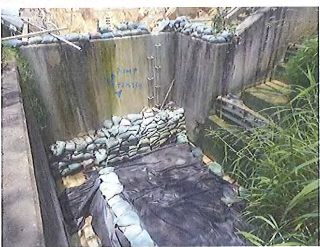
Stream B Outfall: clean water is discharging.
