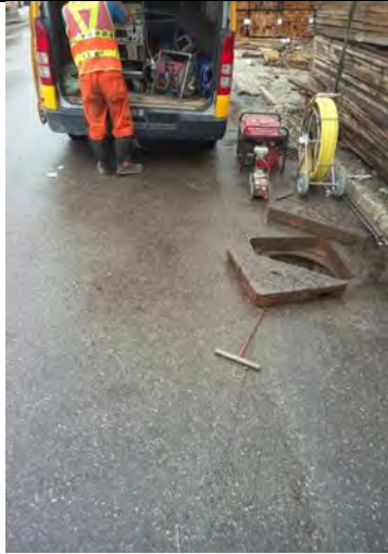
Photo 7 Drainage cleansing works for Ho Fat Lane.
