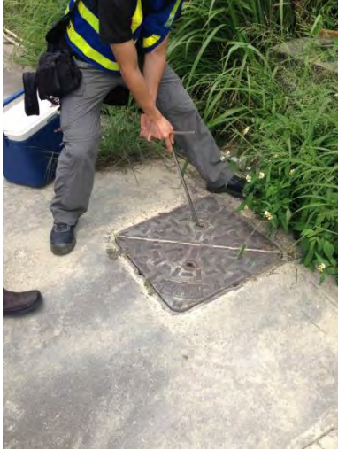
Photo 1 EPD inspecting the concerned manhole on 11 May 2016.
