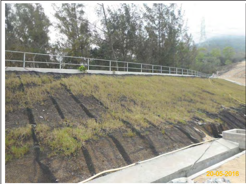
Item 4. Hydro-seeding or sheeting provided at stockpile.
