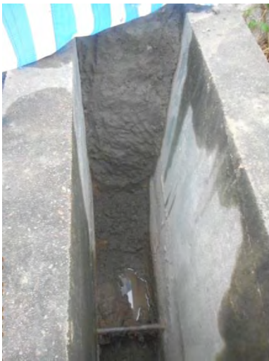
Photo 3 CKJV plugged the inlet of SCH1008705 to ensure no water entering.
