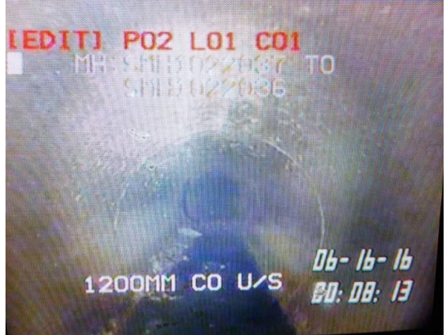
Photo 6 CCTV drainage survey at Ho Yeung Street.
