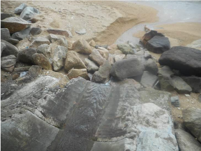
Outfall 1: Clean water is discharging.
