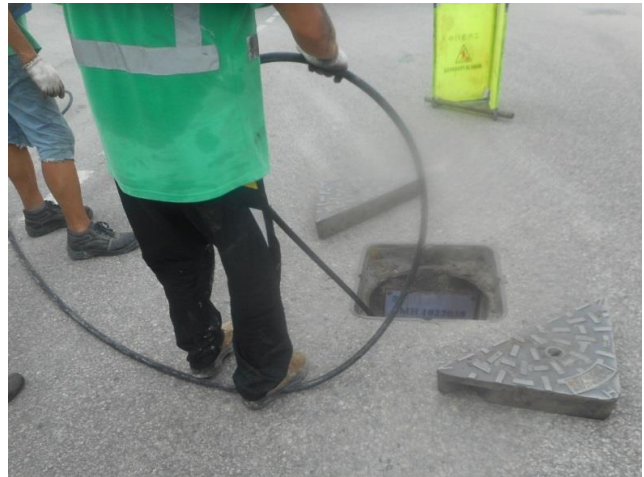
Photo 4 Drainage cleansing works for Ho Yeung Street.
