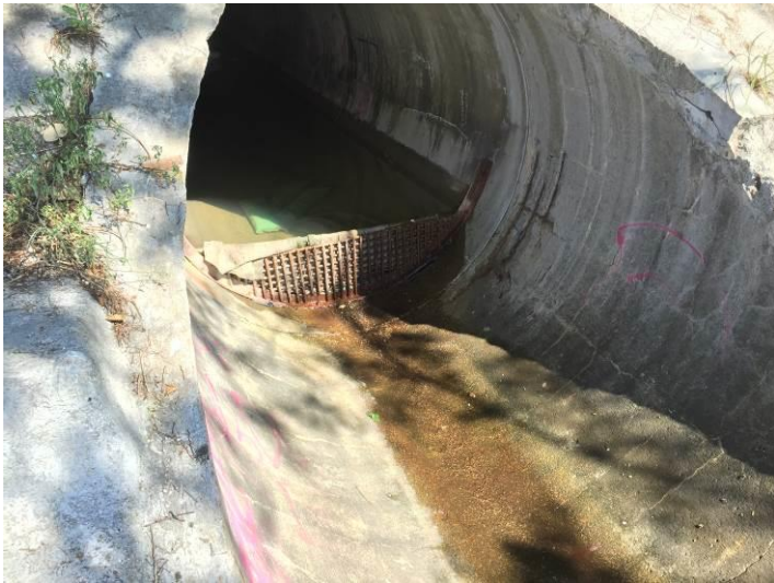
Outfall 1: Clean water is discharging.
