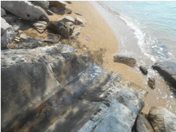
Outfall 1: Clean water is discharging.
