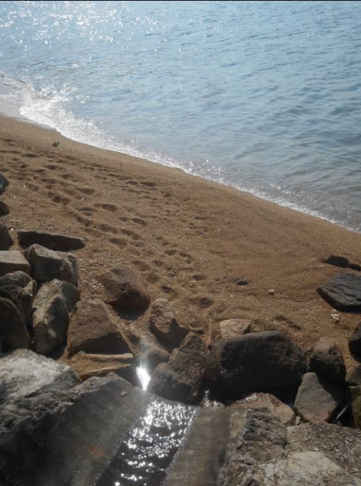
Outfall 1: Clean water is discharging.
