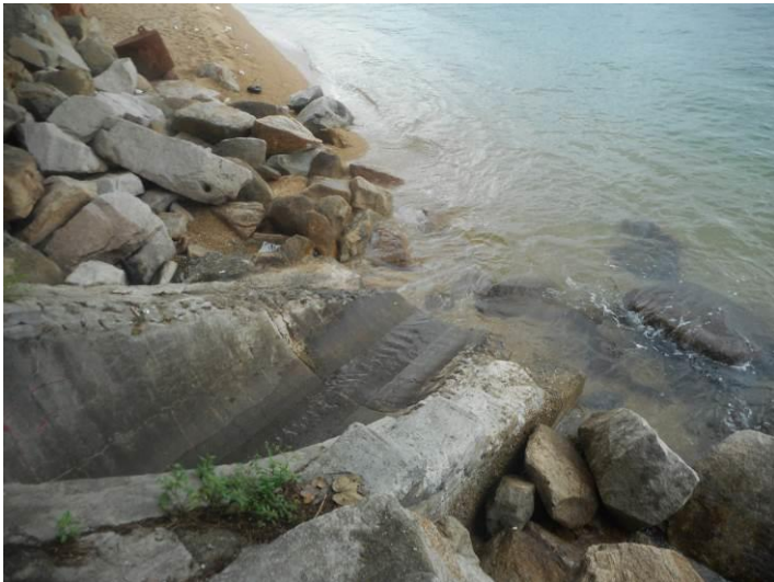
Outfall 1: Clean water is discharging.
