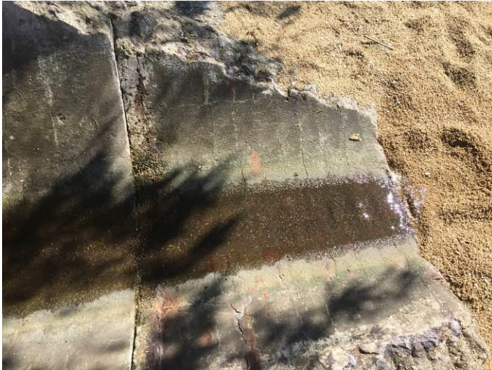
Outfall 1: Clean water is discharging.
