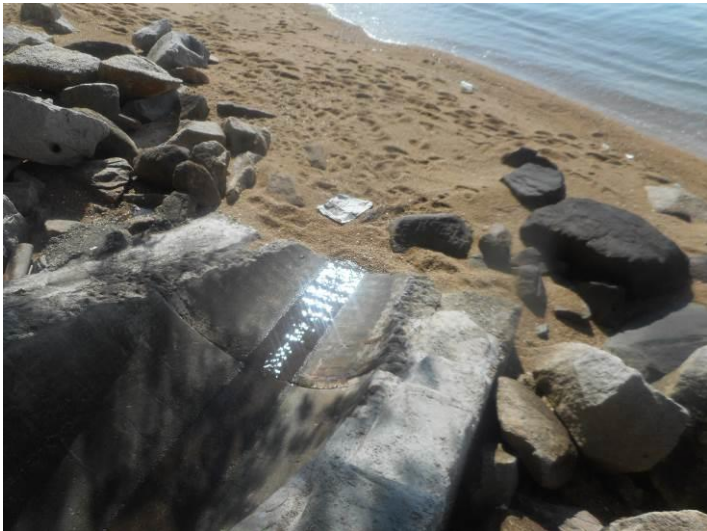
Outfall 1: Clean water is discharging.
