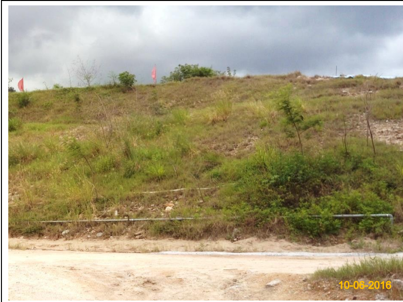
Item 4. Hydro-seeding or sheeting provided at stockpile.
