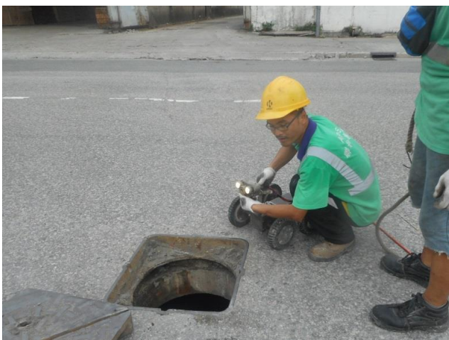
Photo 5 CCTV drainage survey at Ho Yeung Street.
