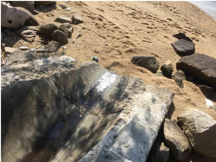
Outfall 1: Clean water is discharging.
