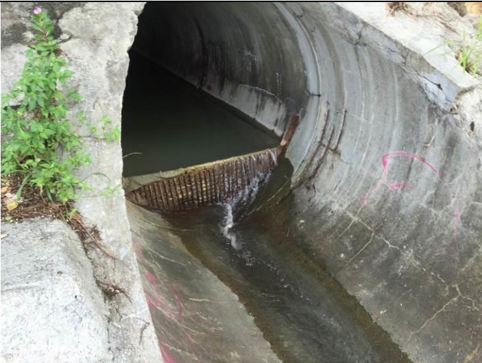
Outfall 1: Clean water is discharging.
