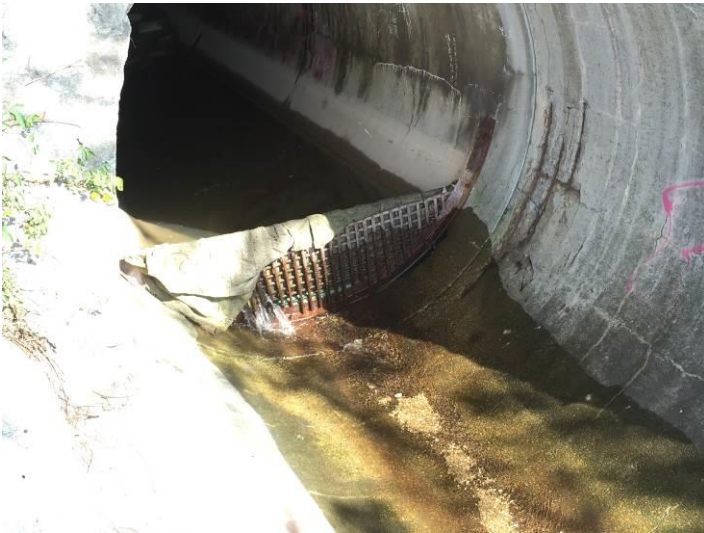
Outfall 1: Clean water is discharging.
