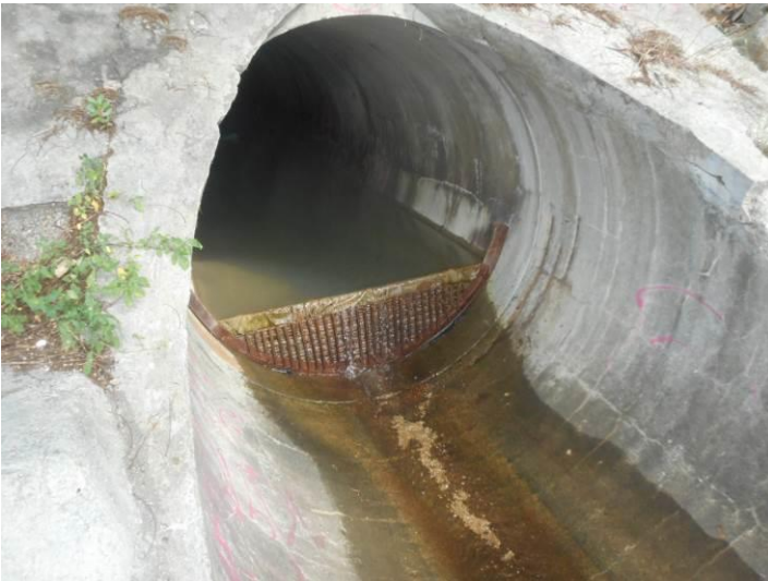
Outfall 1: Clean water is discharging.
