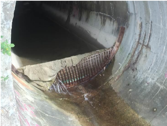
Outfall 1: Clean water is discharging.
