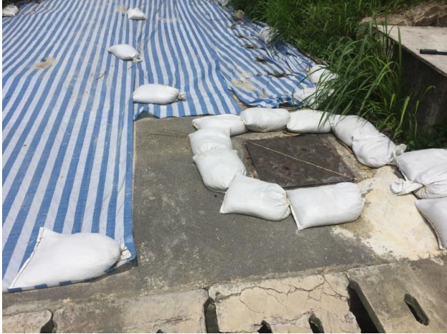
Photo 1 Adjacent area of manhole SCH1008705.
