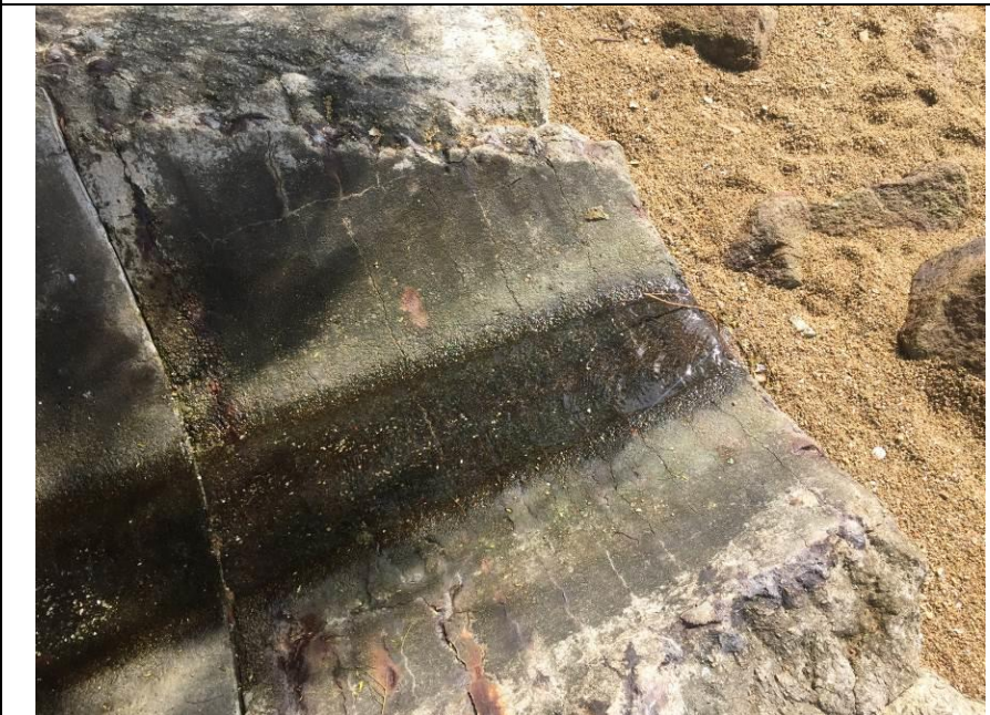
Outfall 1: Clean water is discharging.
