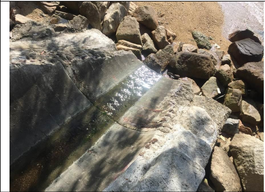
Outfall 1: Clean water is discharging.
