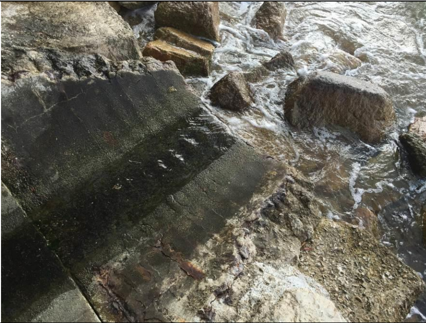
Outfall 1: Clean water is discharging.
