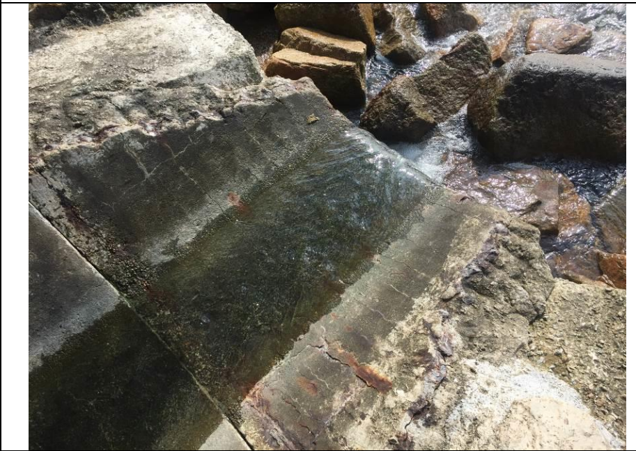
Outfall 1: Clean water is discharging.
