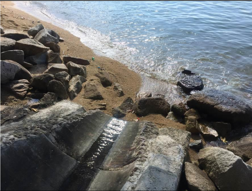
Outfall 1: Clean water is discharging.
