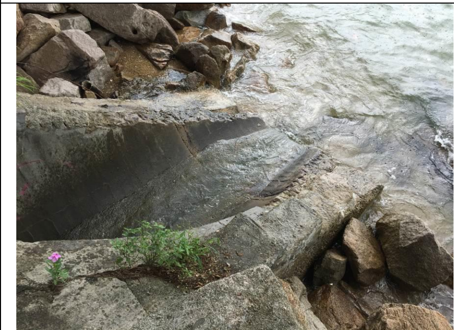
Outfall 1: Clean water is discharging.
