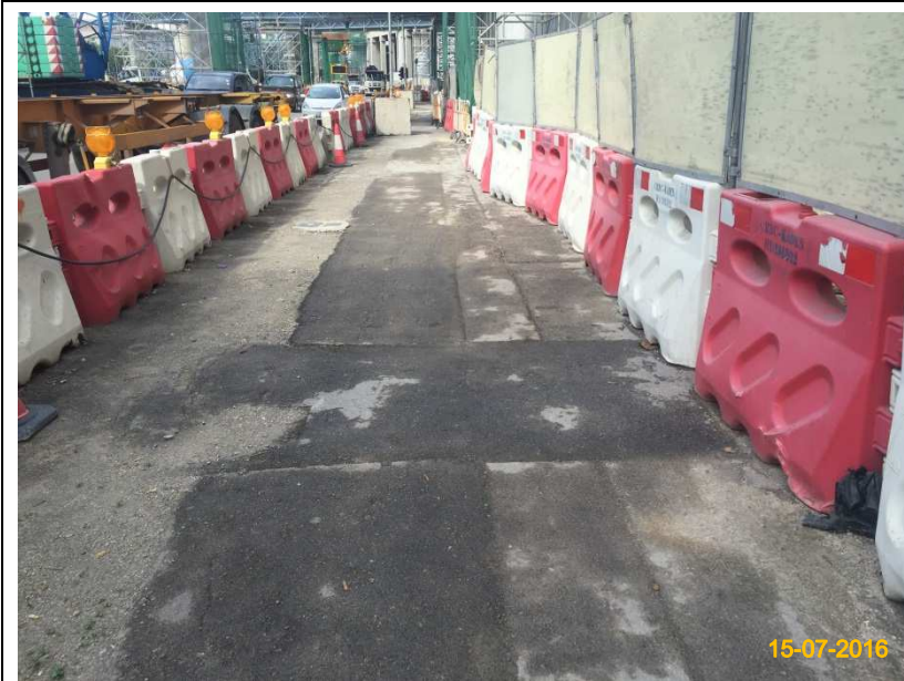
Item 5. Hoarding with panel around works area & Item 6. Temporary traffic management lighting.
