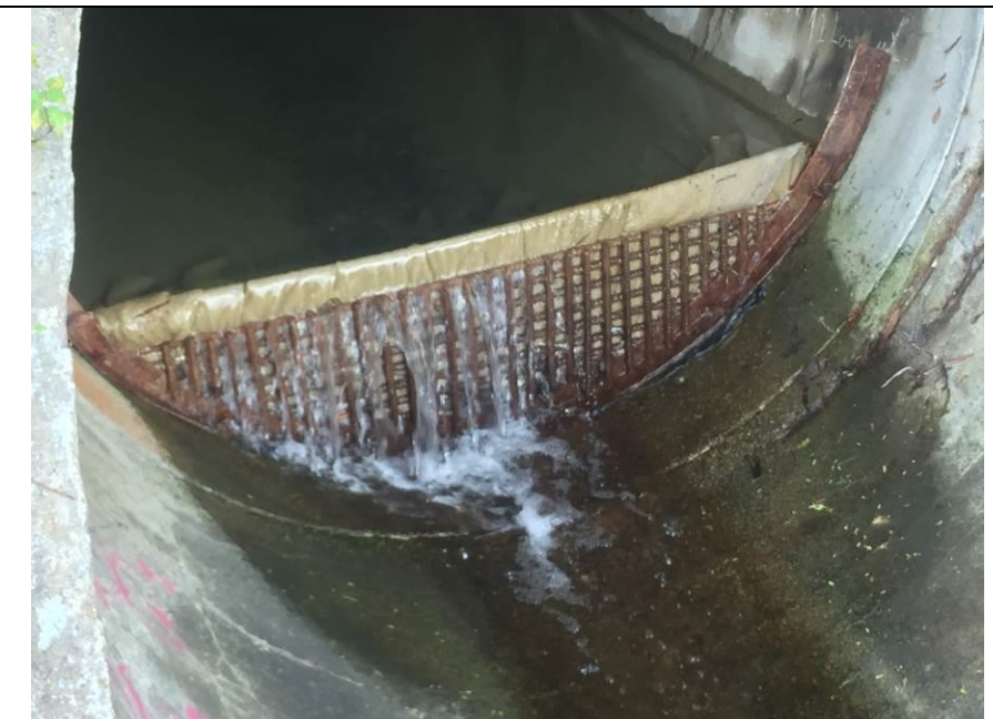
Outfall 1: Clean water is discharging.
