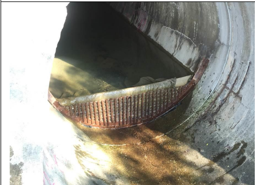
Outfall 1: Clean water is discharging.
