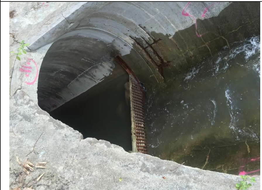
Outfall 1: Clean water is discharging.
