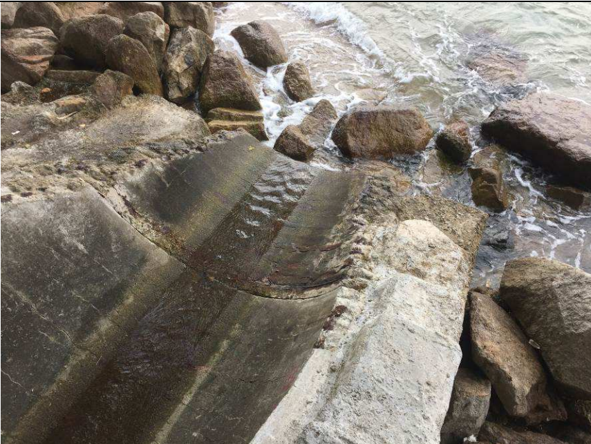
Outfall 1: Clean water is discharging.
