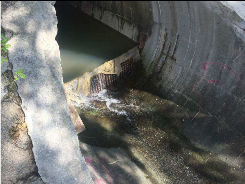
Outfall 1: Clean water is discharging.
