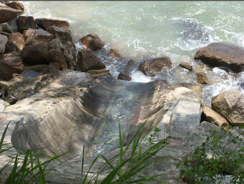
Outfall 1: Clean water is discharging.
