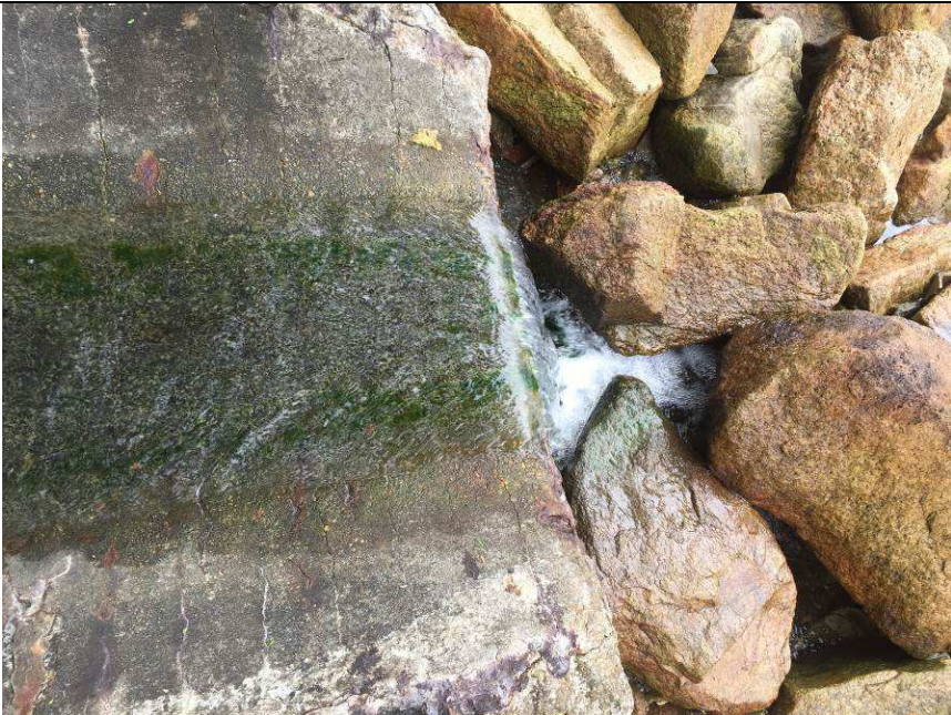
Outfall 1: Clean water is discharging.
