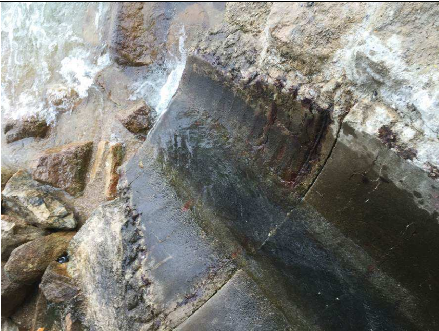
Outfall 1: Clean water is discharging.
