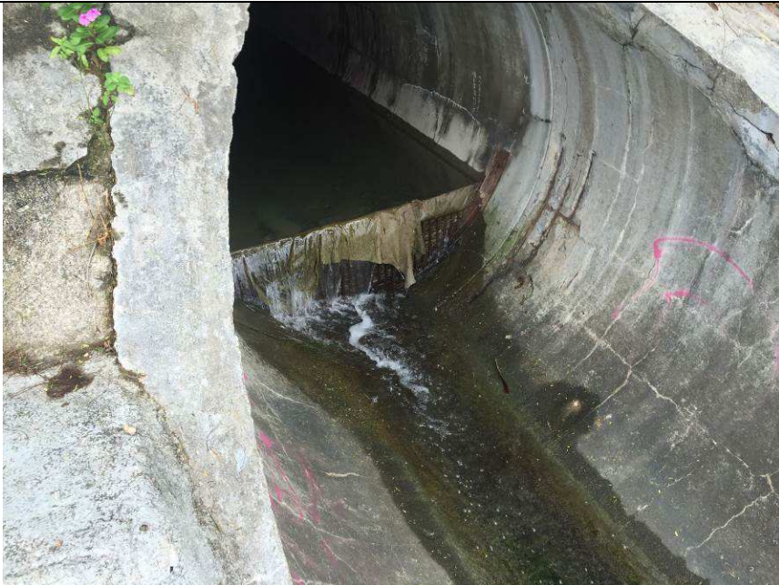
Outfall 1: Clean water is discharging.
