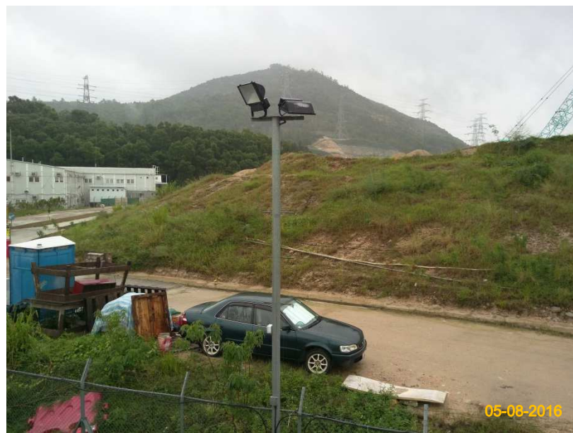
Item 4. Hydro-seeding or sheeting provided at stockpile.
