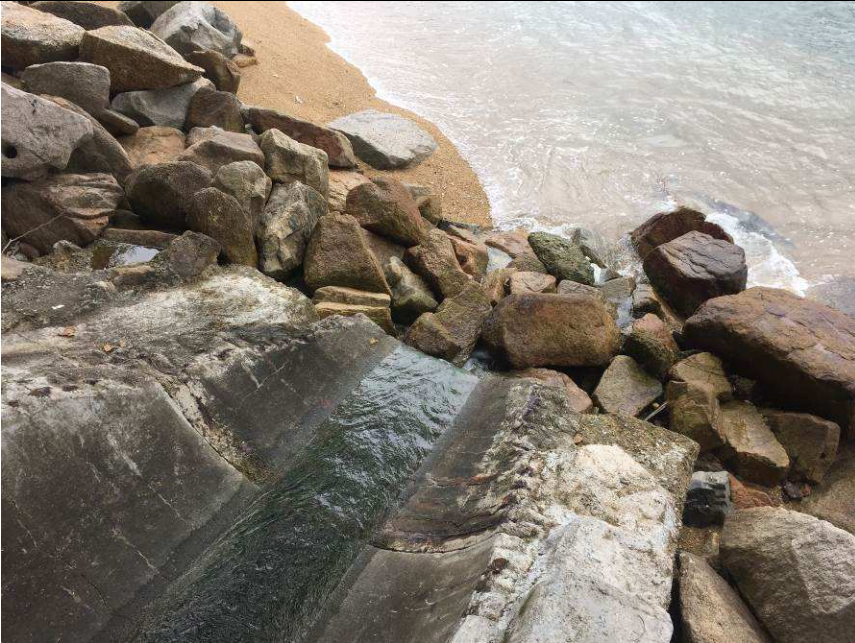
Outfall 1: Clean water is discharging.
