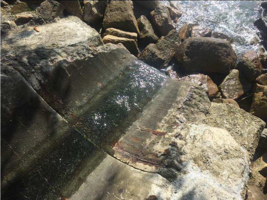
Outfall 1: Clean water is discharging.
