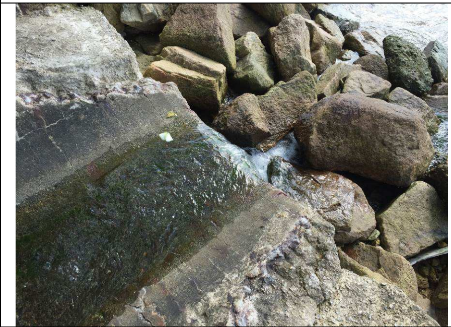
Outfall 1: Clean water is discharging.
