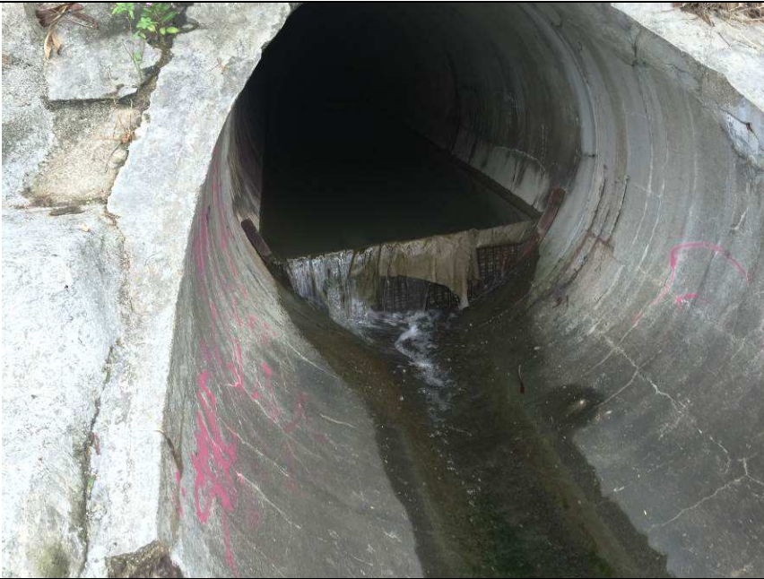
Outfall 1: Clean water is discharging.
