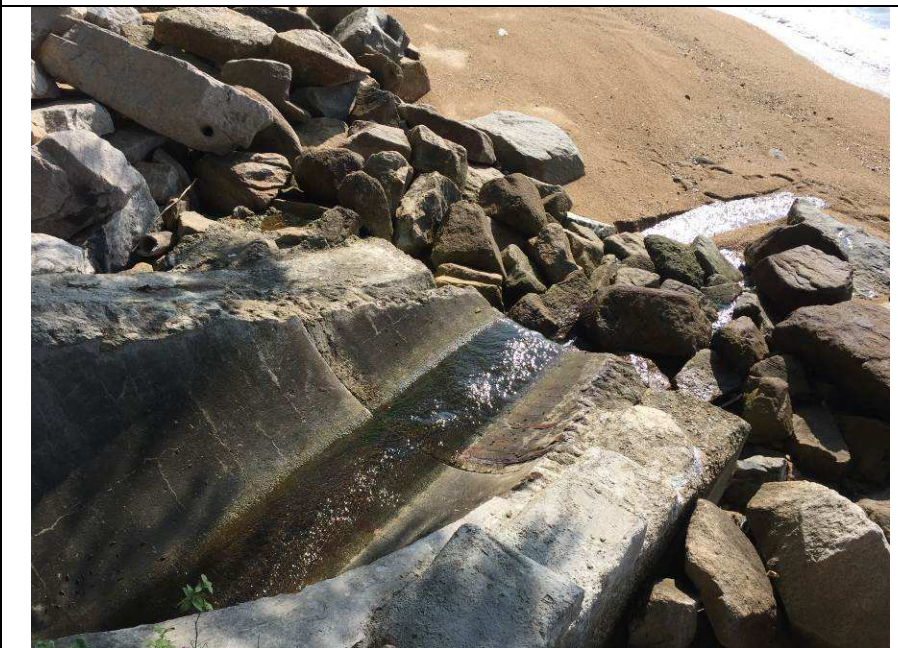
Outfall 1: Clean water is discharging.
