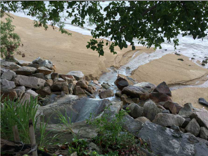
Outfall 1: Clean water is discharging.
