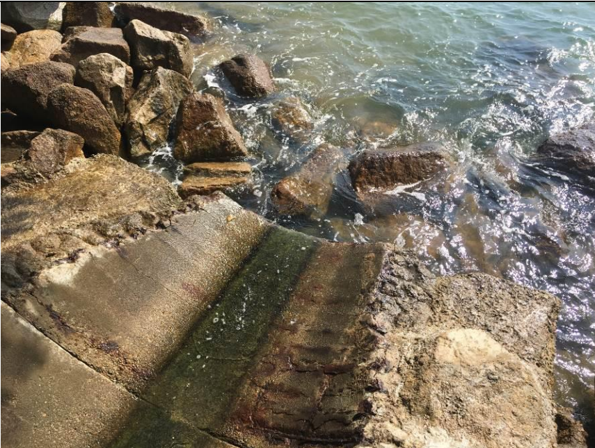
Outfall 1: Clean water is discharging.
