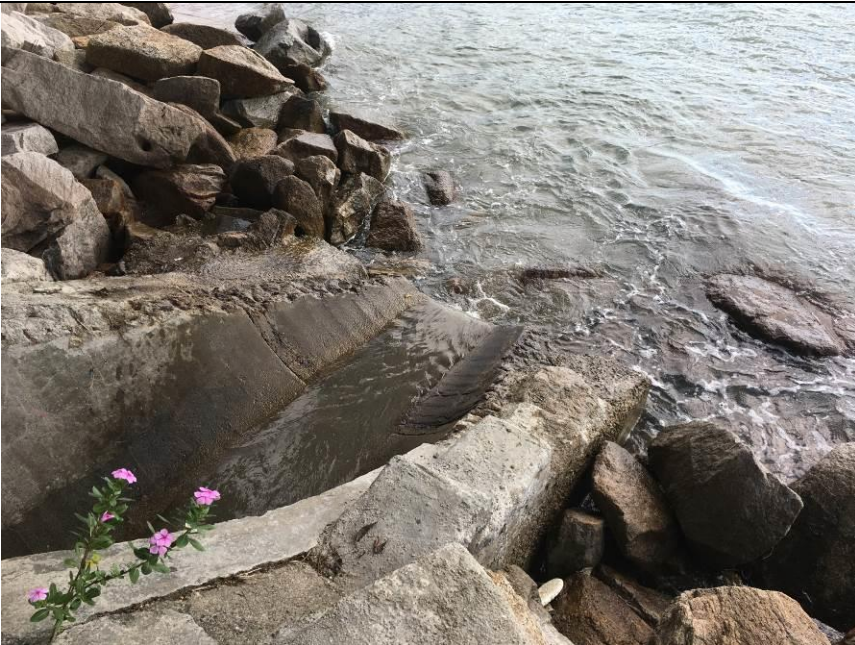
Outfall 1: Clean water is discharging.
