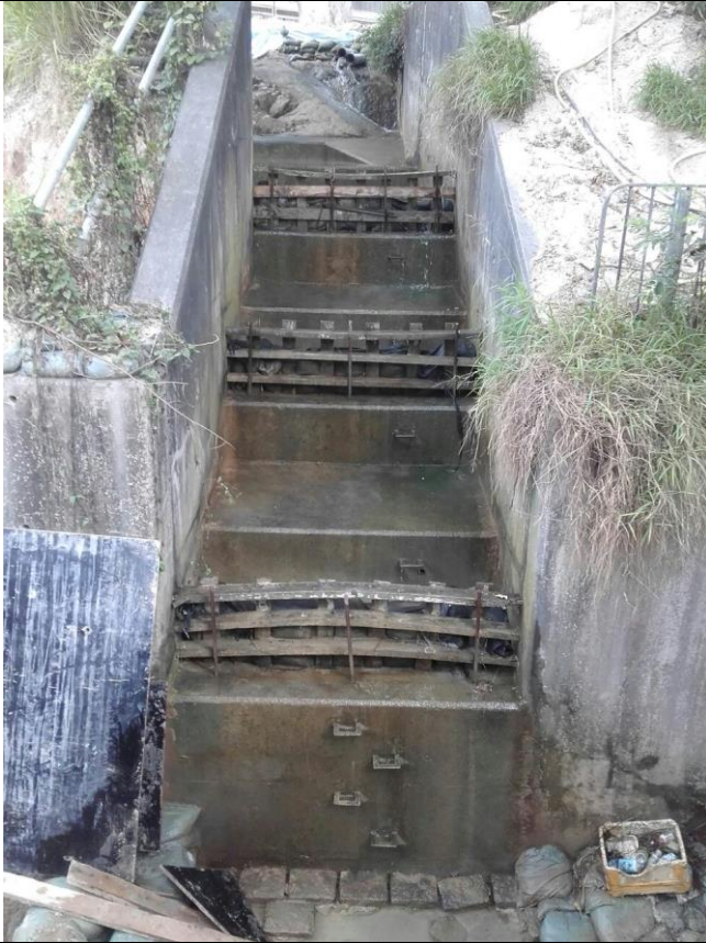
Stream B Outfall: clean water is discharging.
