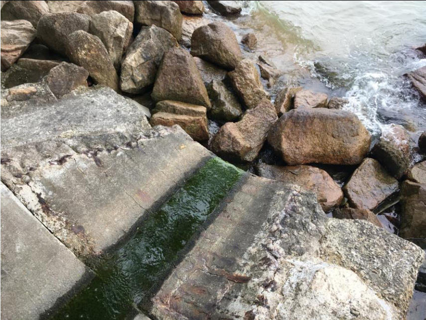
Outfall 1: Clean water is discharging.
