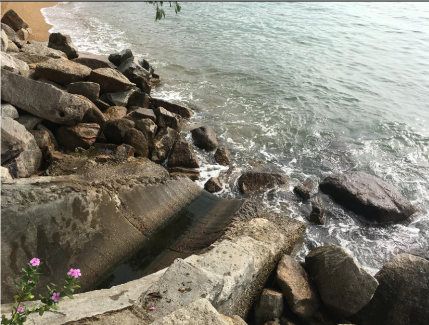
Outfall 1: Clean water is discharging.
