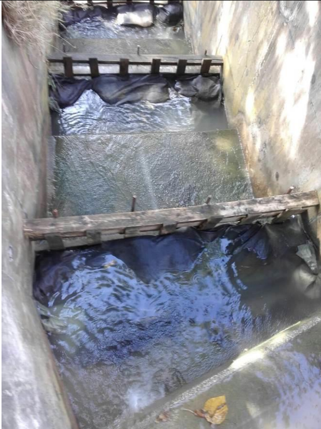
Stream B Outfall: clean water is discharging.
