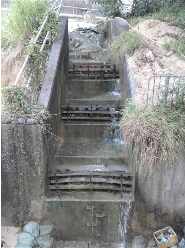
Stream B Outfall: clean water is discharging.
