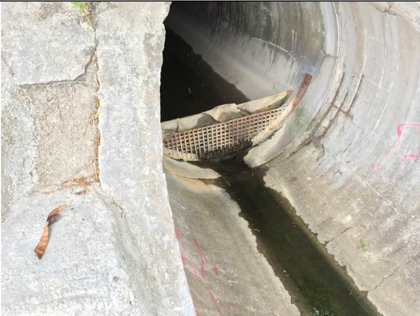
Outfall 1: Clean water is discharging.
