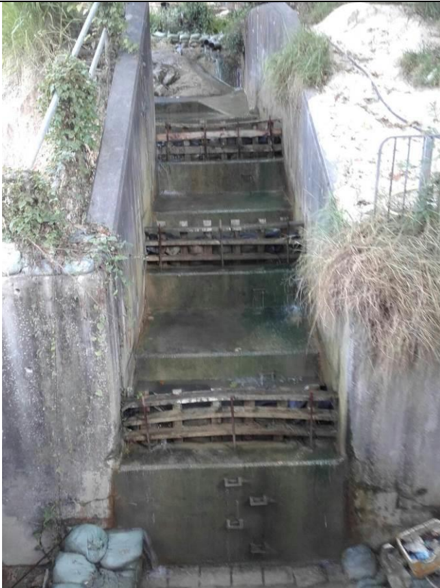
Stream B Outfall: clean water is discharging.
