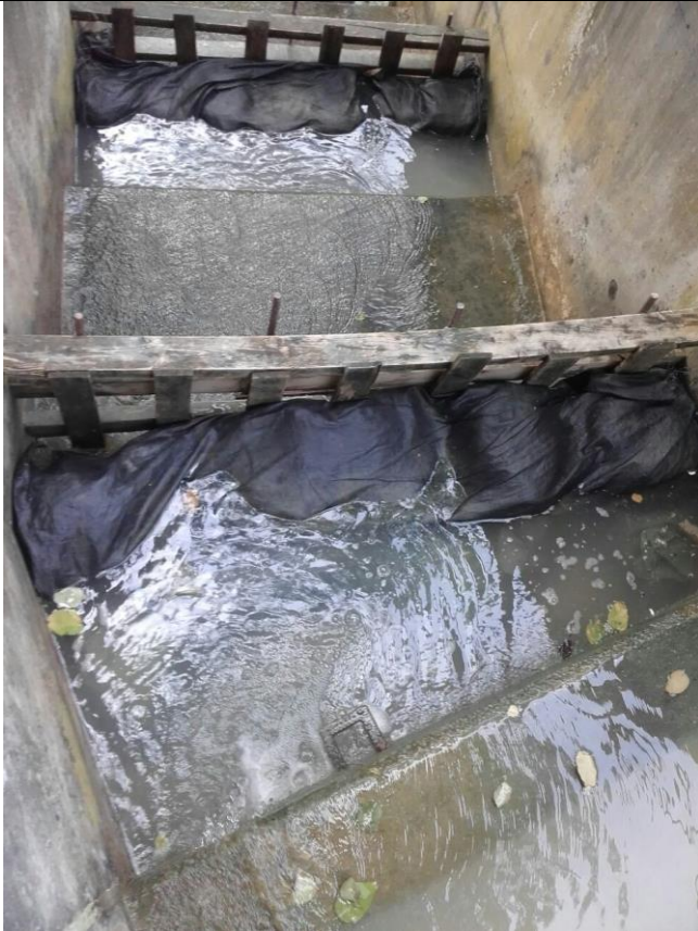
Stream B Outfall: clean water is discharging.
