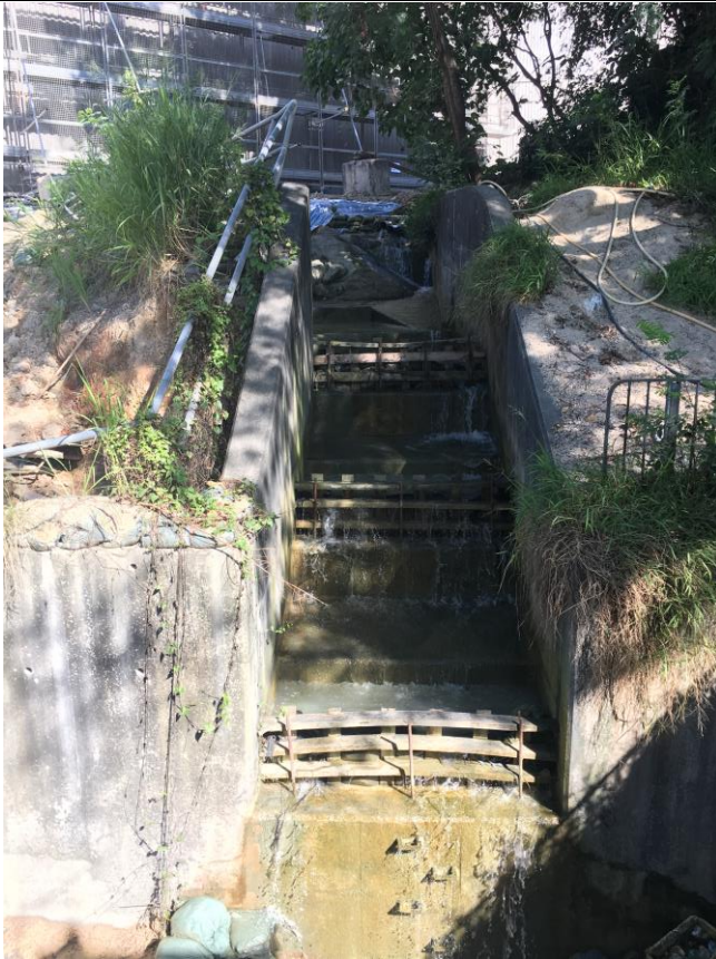
Stream B Outfall: clean water is discharging.
