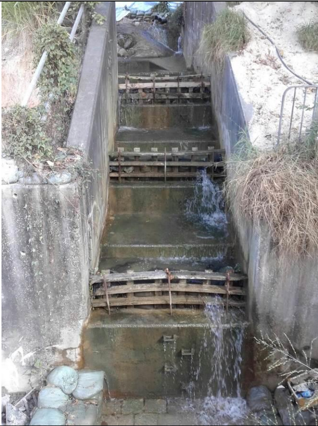
Stream B Outfall: clean water is discharging.
