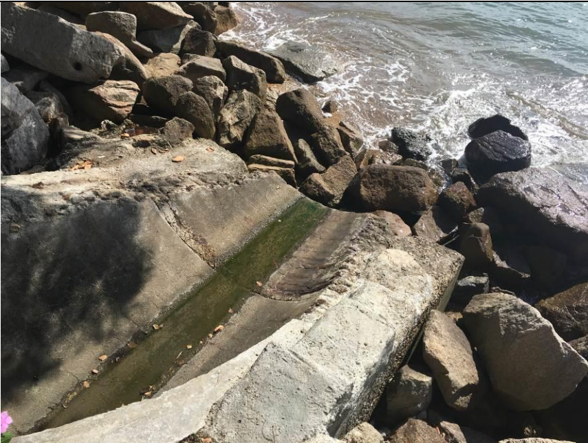
Outfall 1: Clean water is discharging.
