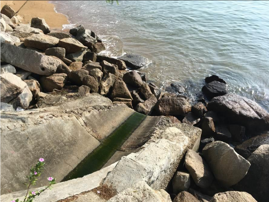
Outfall 1: Clean water is discharging.
