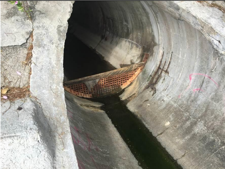
Outfall 1: Clean water is discharging.
