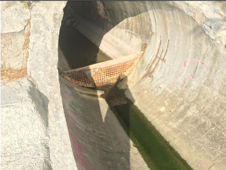
Outfall 1: Clean water is discharging.
