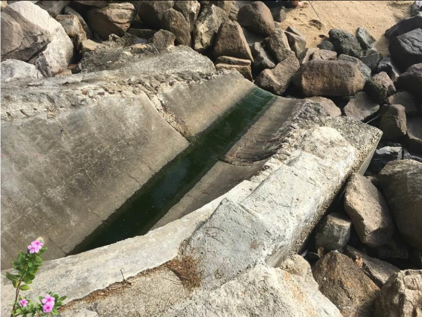
Outfall 1: Clean water is discharging.
