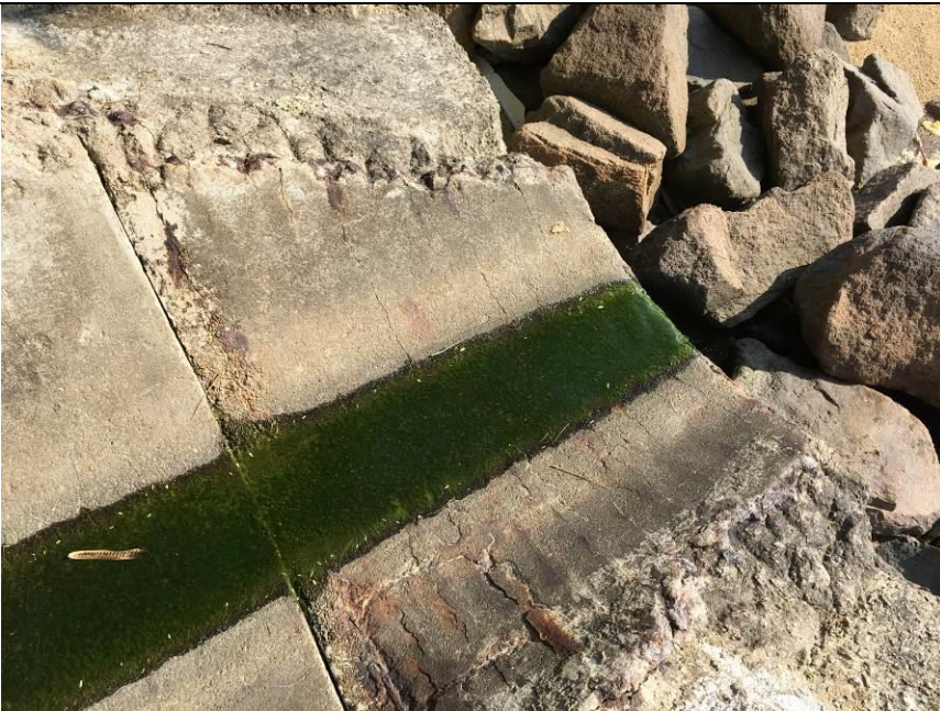
Outfall 1: Clean water is discharging.
