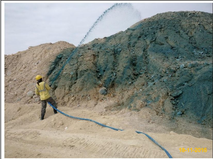
Item 4. Hydro-seeding or sheeting provided at stockpile.
