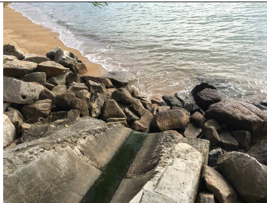
Outfall 1: Clean water is discharging.
