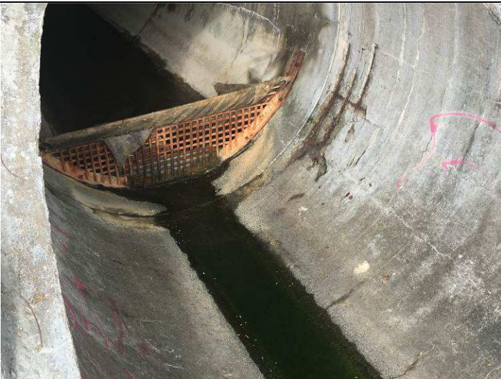
Outfall 1: Clean water is discharging.
