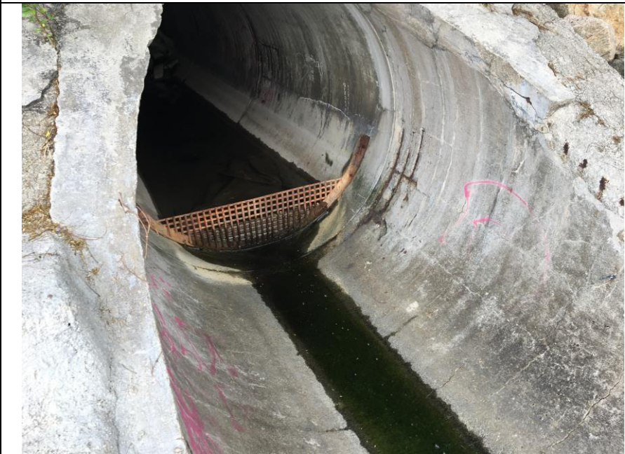
Outfall 1: Clean water is discharging.
