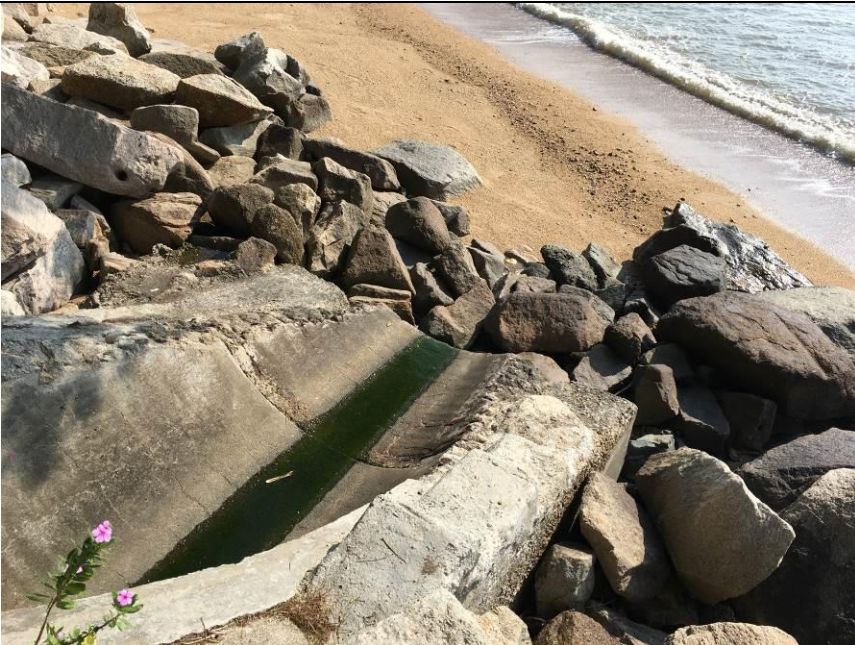
Outfall 1: Clean water is discharging.
