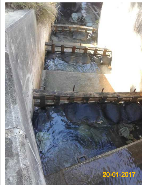
Item 7. Ensure no run-off into water body.
