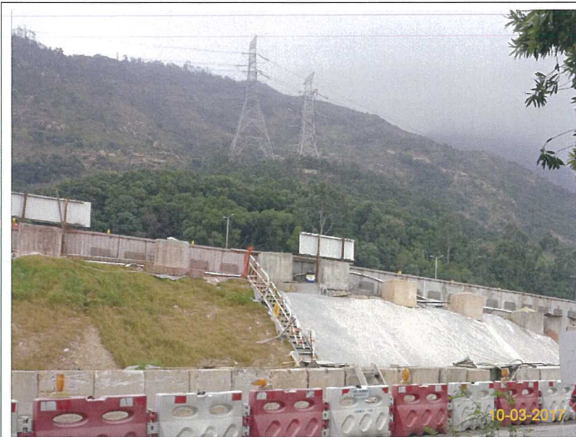
Item 4. Hydro-seeding or sheeting provided at stockpile.
