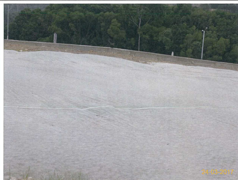
Item 4. Hydro-seeding or sheeting provided at stockpile.
