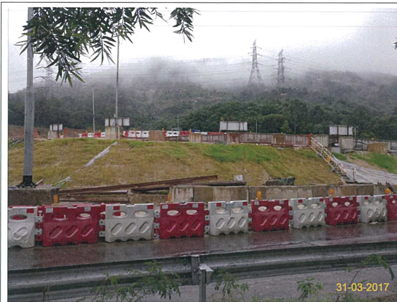
Item 4. Hydro-seeding or sheeting provided at stockpile.
