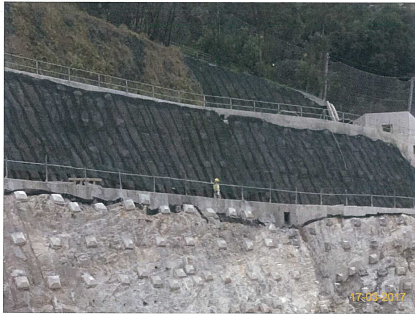
Item 4. Hydro-seeding or sheeting provided at stockpile.
