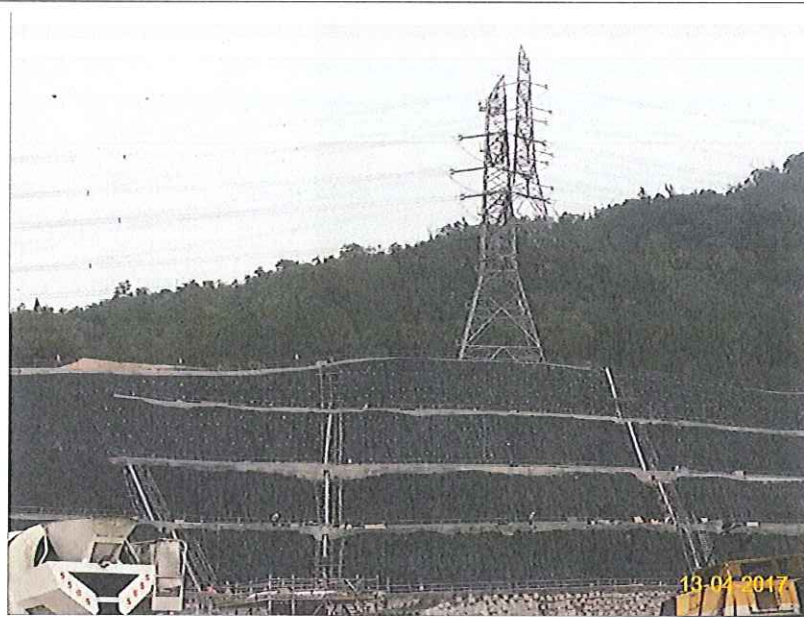
Item 4. Hydro-seeding or sheeting provided at stockpile.
