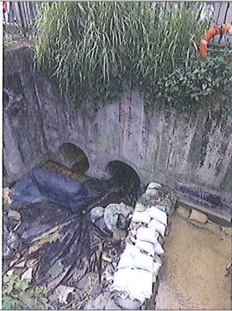
Stream B Outfall: clean water is discharging.
