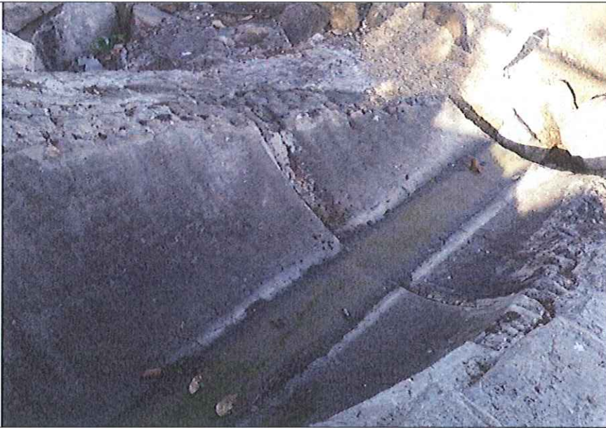
Outfall 1: Clean water is discharging.
