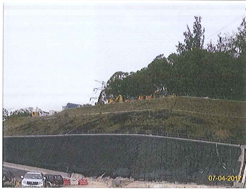
Item 4. Hydro-seeding or sheeting provided at stockpile.
