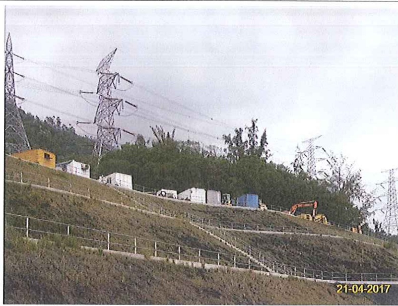
Item 4. Hydro-seeding or sheeting provided at stockpile.
