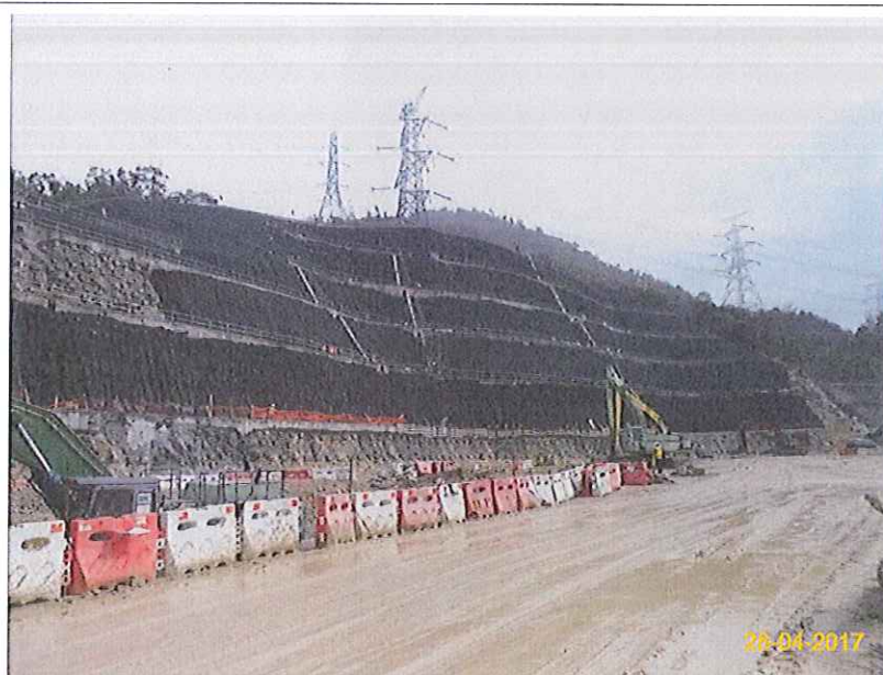
Item 4. Hydro-seeding or sheeting provided at stockpile.
