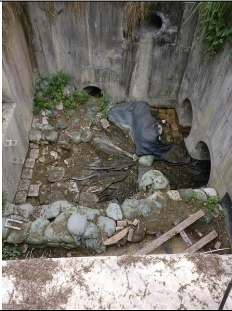
Stream B Outfall: No water is discharging.
