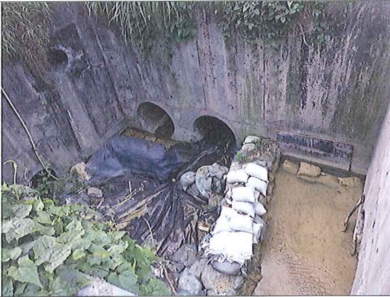
Stream B Outfall: clean water is discharging.
