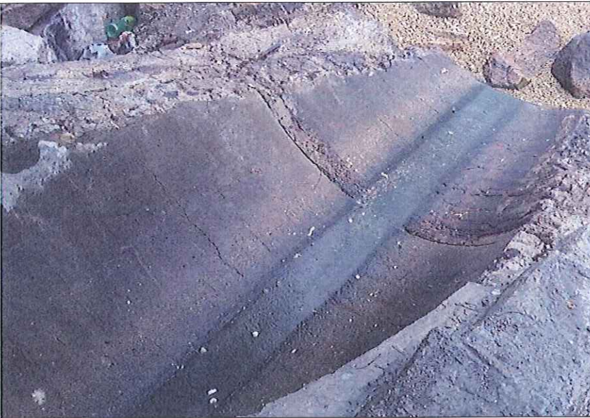
Outfall 1: Clean water is discharging.
