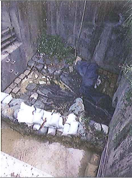
Stream B Outfall: clean water is discharging.
