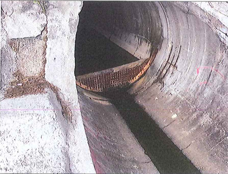
Outfall 1: Clean water is discharging.
