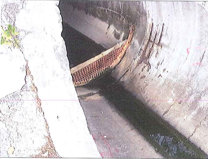
Outfall 1: Clean water is discharging.
