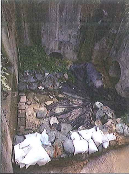
Stream B Outfall: clean water is discharging.
