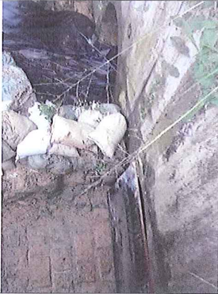
Stream B Outfall: Clean water is discharging.
