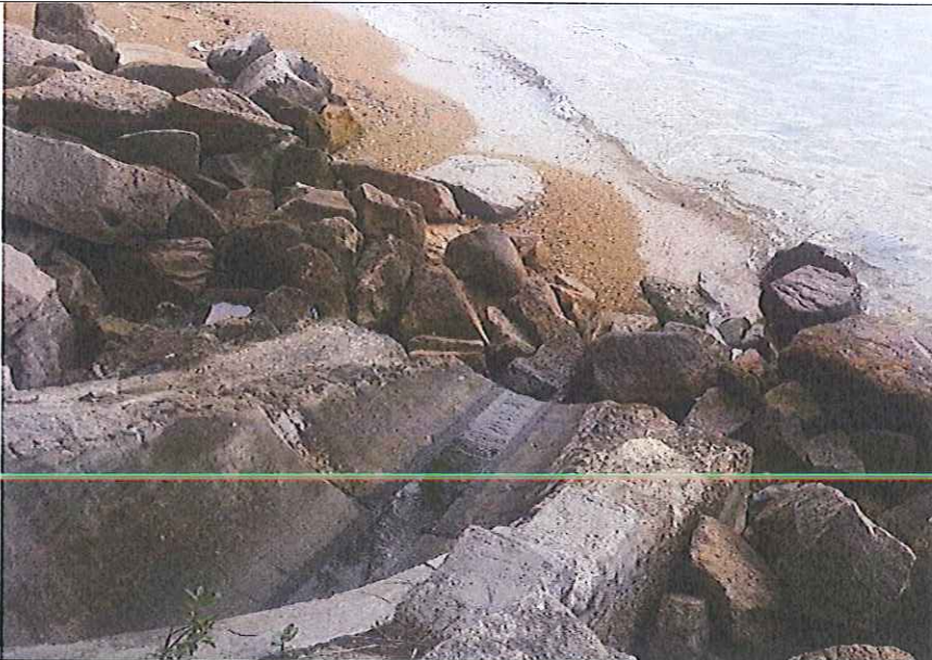
Outfall 1: No water is discharging.
