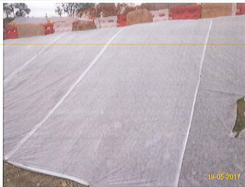
Item 4. Hydro-seeding or sheeting provided at stockpile.
