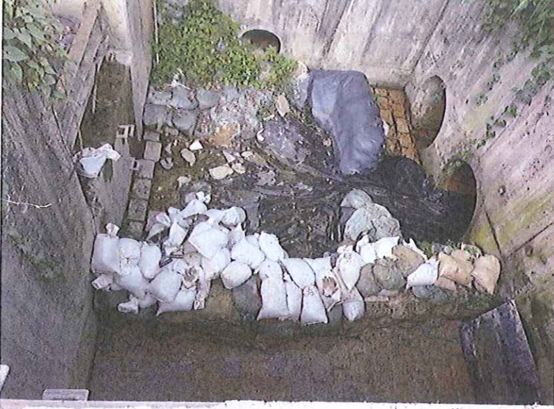
Stream B Outfall: clean water is discharging.
