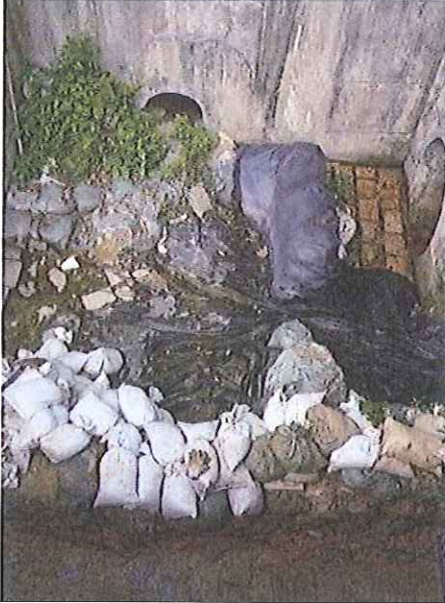
Stream B Outfall: clean water is discharging.
