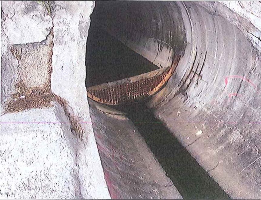
Outfall 1: Clean water is discharging.
