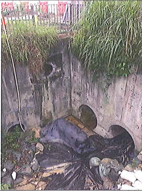
Stream B Outfall: No water is discharging.
