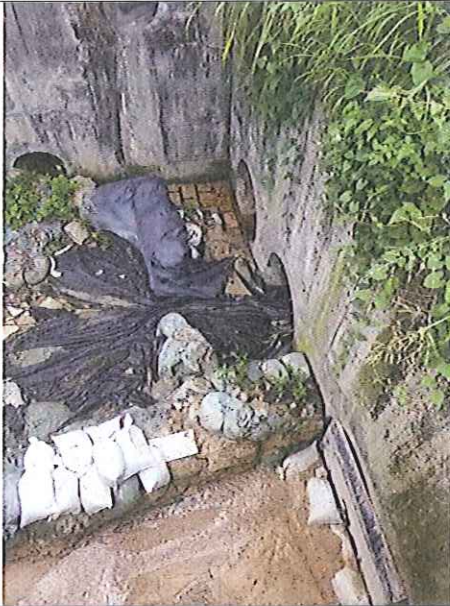
Stream B Outfall: clean water is discharging.
