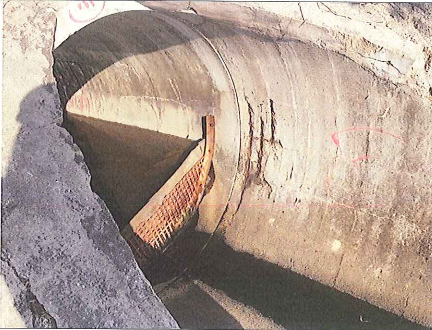
Outfall 1: Clean water is discharging.
