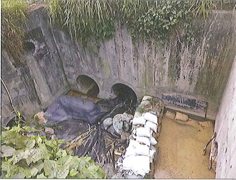
Stream B Outfall: No water is discharging.
