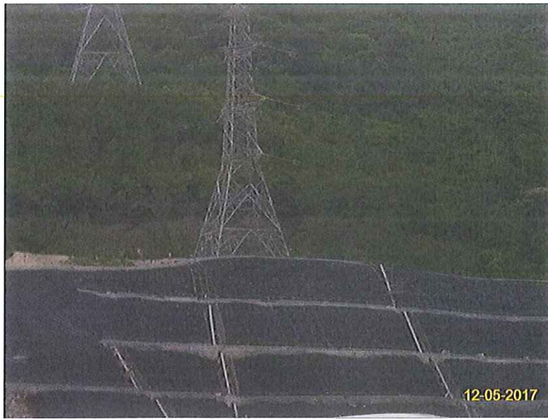
Item 4. Hydro-seeding or sheeting provided at stockpile.
