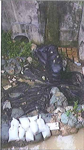
Stream B Outfall: clean water is discharging.
