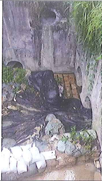
Stream B Outfall: No water is discharging.
