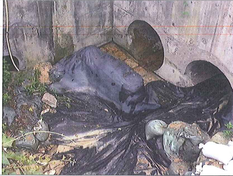
Stream B Outfall: No water is discharging.
