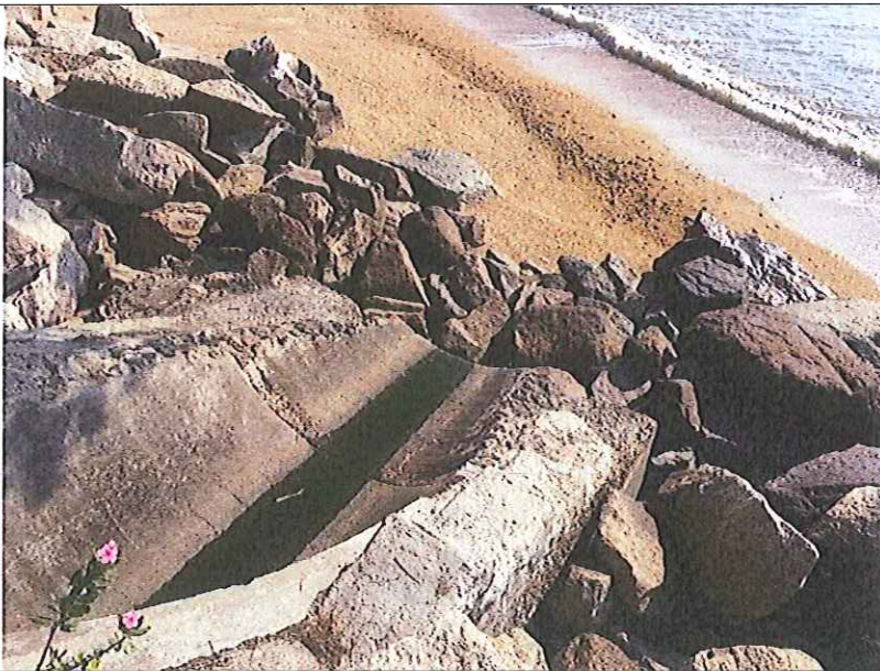
Outfall 1: Clean water is discharging.
