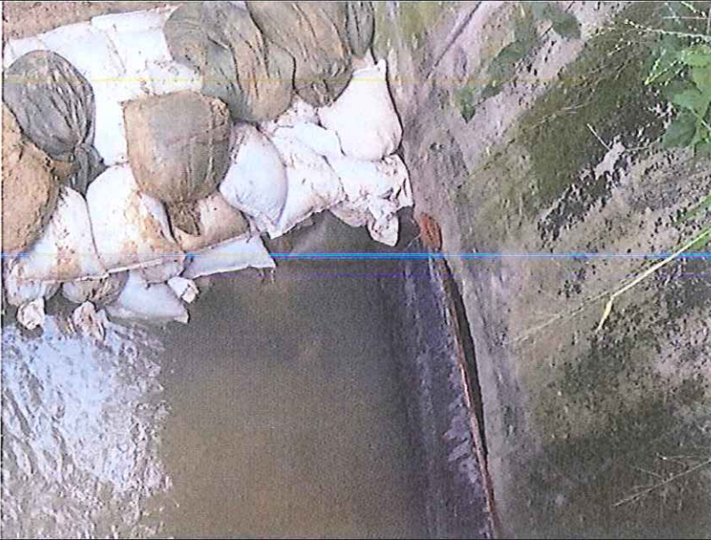
Stream B Outfall: clean water is discharging.
