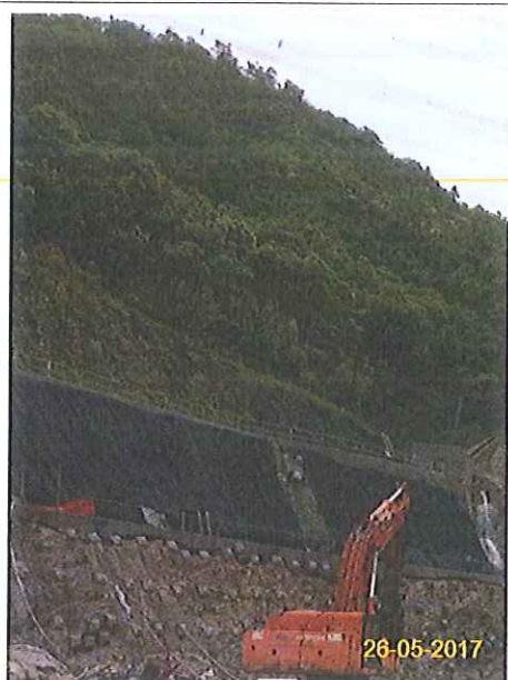
Item 4. Hydro-seeding or sheeting provided at stockpile.
