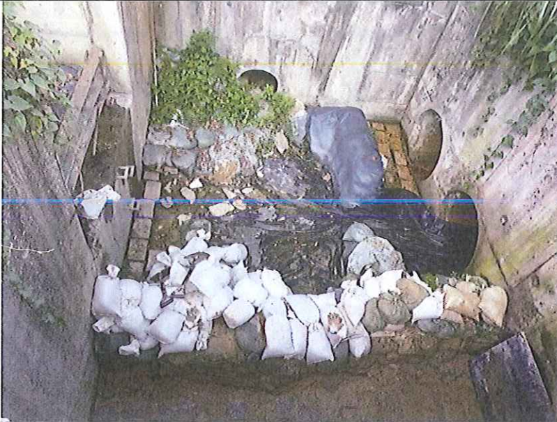
Stream B Outfall: No water is discharging.
