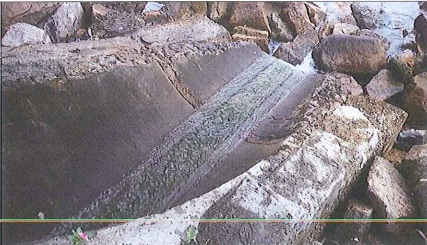
Outfall 1: No water is discharging.
