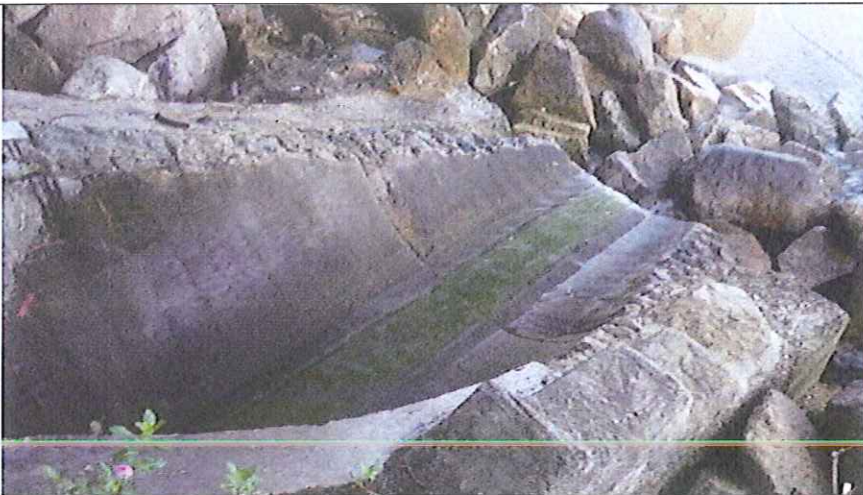
Outfall 1: No water is discharging.
