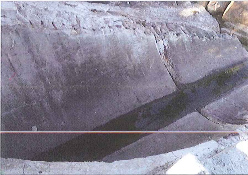
Outfall 1: Clean water is discharging.
