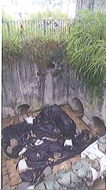
Stream B Outfall: No water is discharging.
