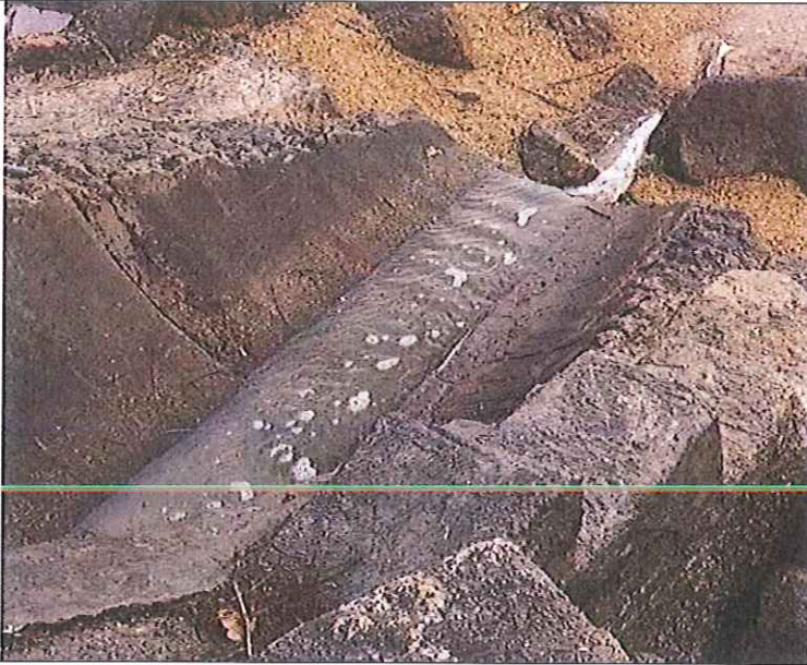
Outfall 1: Clean water is discharging.
