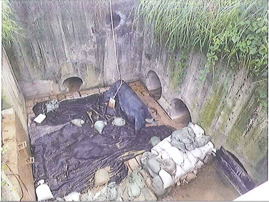
Stream B Outfall: No water is discharging.
