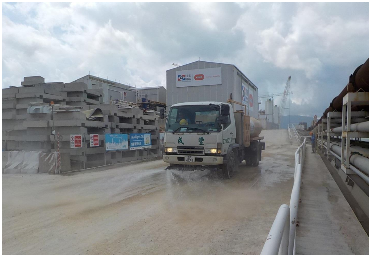
Use of water truck on exposed soil within the Project site and associated work areas. (Works Area Portion N-C)
